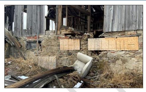
Photograph 5: Destabilized rubblestone foundation wall
