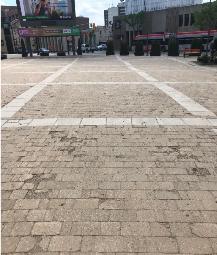
Garden Square requires resurfacing. Robust materials should be specified to carry vehicular and pedestrian traffic. Replacement cost has not been quantified.
