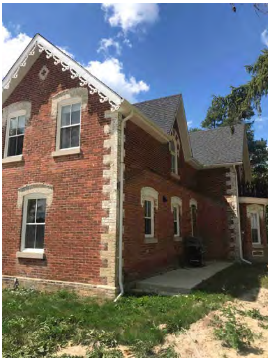
FRONT & SIDE ELEVATIONS – heritage attributes include dichromatic brickwork, painted brick moulds, cross gable roof with a center gable and decorative bargeboards, bay window with decorative iron railings
