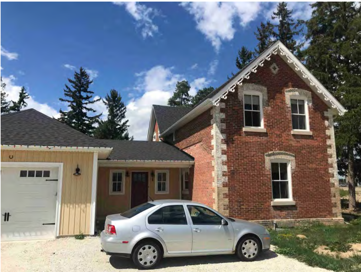
EXISTING REAR ADDITION – a modern entryway and garage oriented towards Grafton Crescent are attached to the rear elevation of the heritage building – this addition will be removed and the new addition will be attached in the same location
