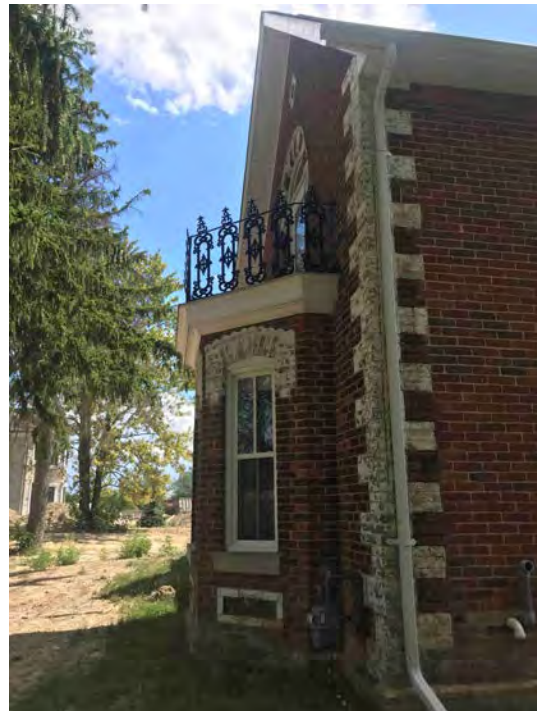
FRONT & SIDE ELEVATIONS – heritage attributes include dichromatic brickwork, painted brick moulds, cross gable roof with a center gable and decorative bargeboards, bay window with decorative iron railings
