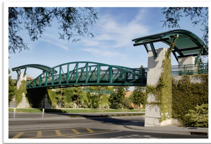
Figure 5 – Representative Photograph of Prefabricated Bowstring Arch Bridge
