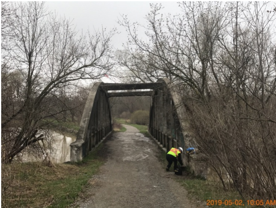
South elevation (looking north).
