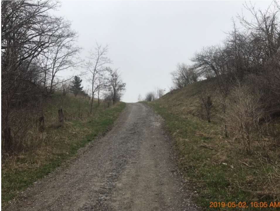
South approach (looking south).
