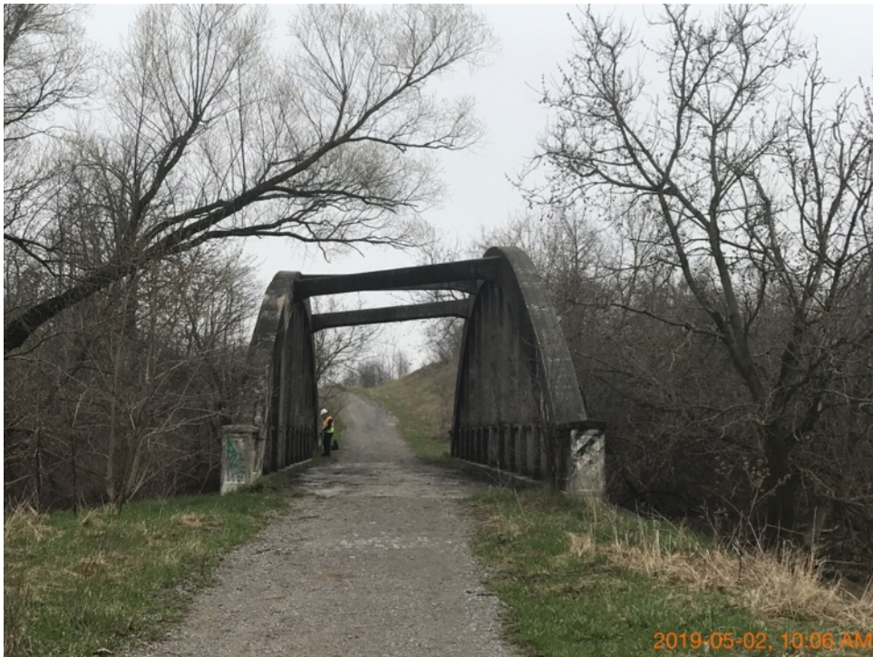
North elevation (looking south).
