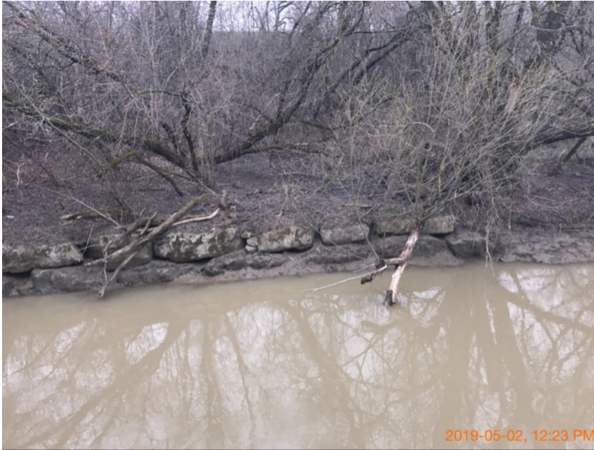
Failed trees in watercourse along south shoreline (upstream / west of bridge).
