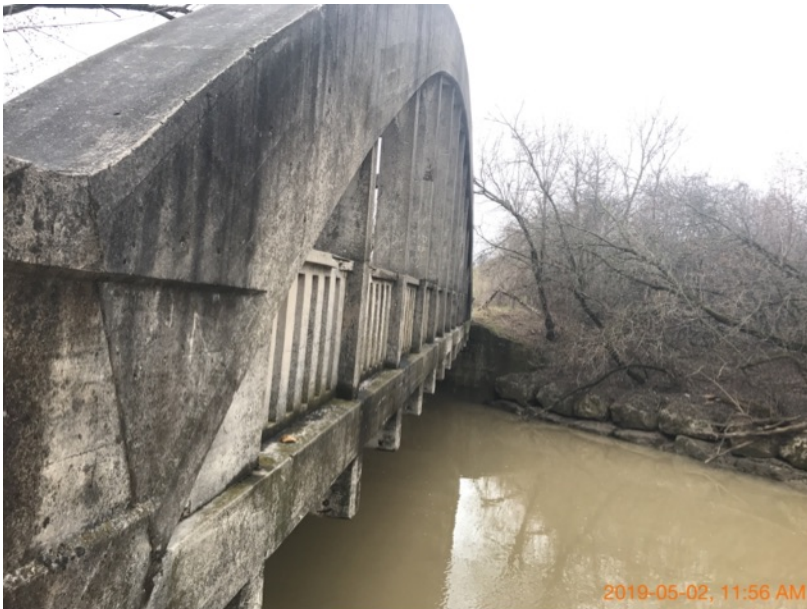
East fascia (looking north).
