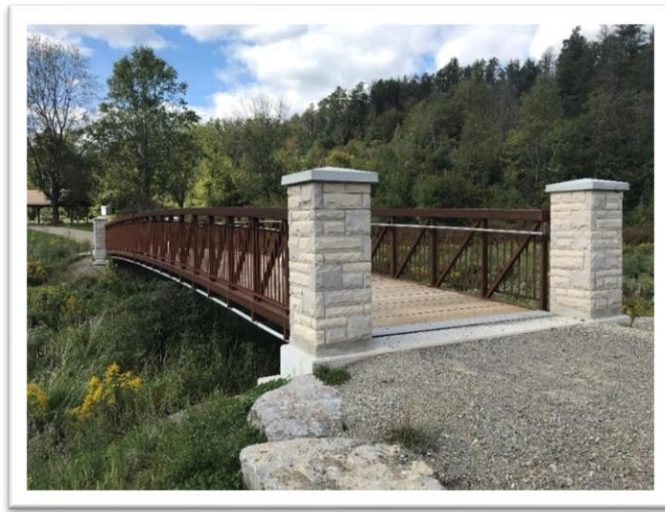
Figure 3 – Representative Photograph of Prefabricated Steel Pratt Truss Bridge
