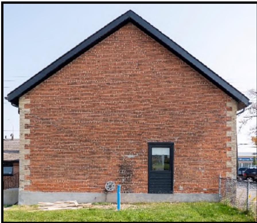
Figure 10: The south elevation of the 1874 Schoolhouse building, showing unoriginal door opening and some scarring to the left.
