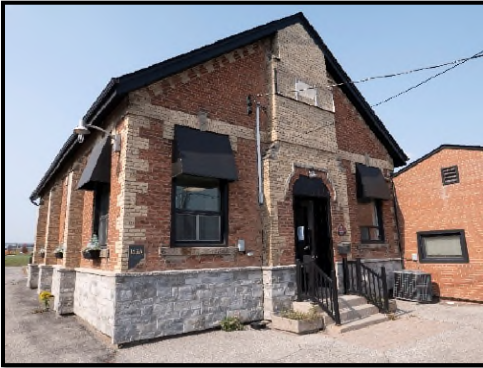
Figure 8: The west elevation of the 1874 Schoolhouse building, with the original brickwork visible on the closest bay where the veneer wall has been removed.
