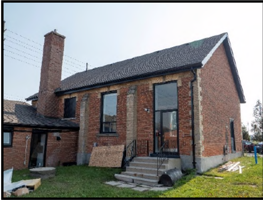
Figure 10: The south elevation of the 1874 Schoolhouse building, showing unoriginal door opening and some scarring to the left.
