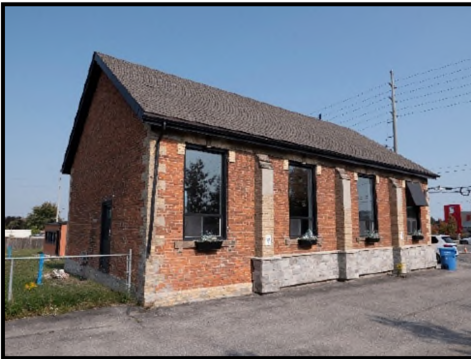
Figure 8: The west elevation of the 1874 Schoolhouse building, with the original brickwork visible on the closest bay where the veneer wall has been removed.
