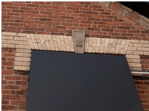
Figure 12: Typical eared jack arch as seen on the south elevation, aligned with the projecting band course and embellished with a cast keystone.
