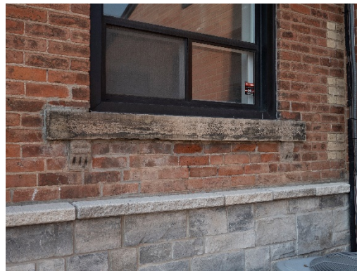
Figure 13: Typical window sill seen on the south elevation, with tooled sandstone sill above two cast masonry brackets. The high deterioration of the brackets is common to the entire structure.
