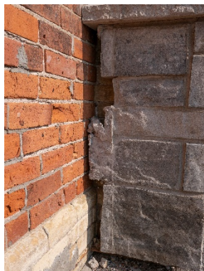
Figure 10: Historic brickwork is visible in behind the veneer stones, and the previously covered brickwork to the left shows spalling and mortar loss.
