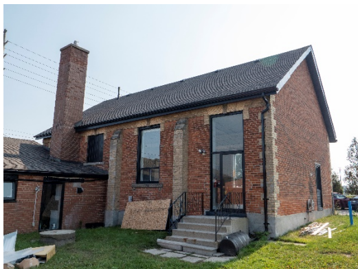
Figure 7: The east elevation of the 1874 Schoolhouse building, showing one original and three modified window openings.
