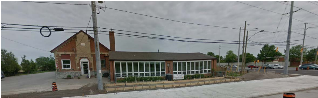
Figure 21: 2012 Google image showing the 1950s additions prior to construction of transit shelter obscuring the current view. Differences in roof sag are seen between the two sections, along with a zipper joining suggesting different times of construction (Google 2012).
