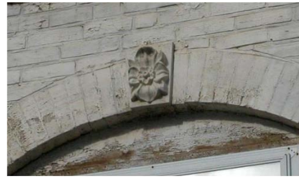
Figure 32: Image of an arch at the Haggartlea Estate in Brampton, showing the keystone which might be a cast stone detail. The photo also shows horizontal tooling in the surrounding brick joints similar to that of the Schoolhouse (Heritage Report: Reasons for Designation Haggartlea 28 Elizabeth Street North).
