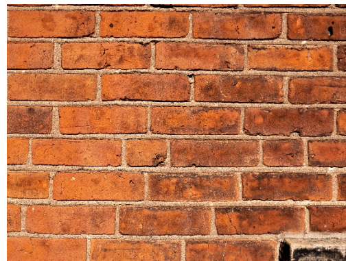
Figure 11: A section of intact mortar. Some degree of horizontal tooling is evident by lines demarcating horizontal and vertical joints.
