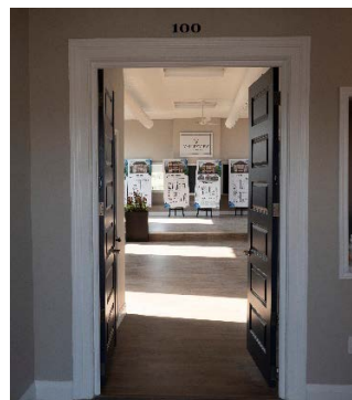
Figure 19: Mouldings on the doorway leading to the main classroom. Note unoriginal baseboards and new frame built within the original to support current doors.
