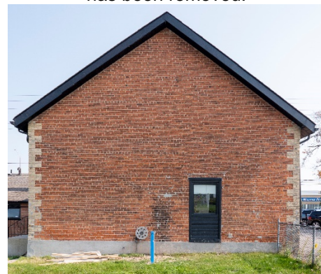
Figure 8: The north elevation of the 1874 Schoolhouse building, showing unoriginal door opening and some scarring to the left.
