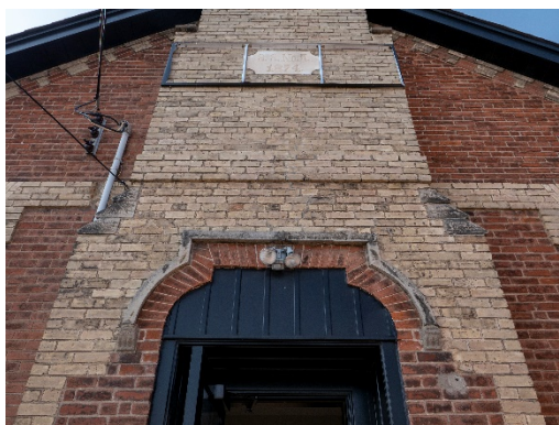
Figure 14: The projecting entry frontispiece, showing sandstone transition stones and hood mould. Despite its elaborate shape, the hood mould is built from three pieces of stone.
