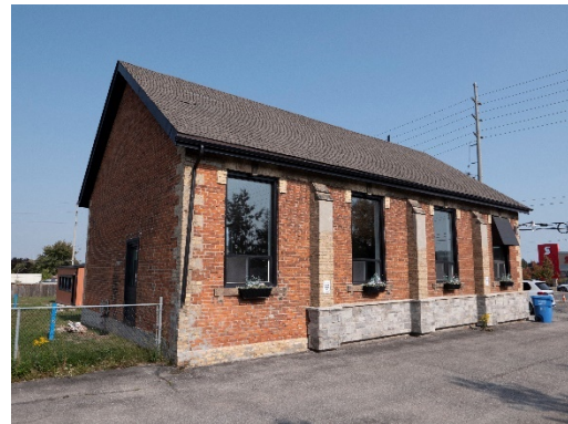
Figure 6: The west elevation of the 1874 Schoolhouse building, with the original brickwork visible on the closest bay where the veneer wall has been removed.
