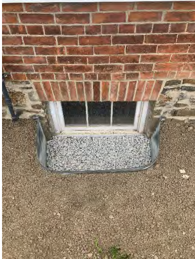
Figure 25: The west elevation of the McClure House building showing the fieldstone foundation (approximately 2 ft. high) capped by a flat arch head with a single order of soldier brick voussoirs, which is followed by a course of bricks laid in English bond. A window well was also recently added to prevent dirt and debris from entering through the basement window.
