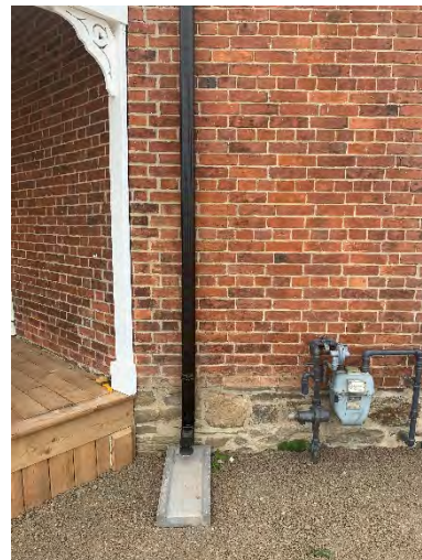
Figure 28: The exterior walls include red brick laid in English Garden Wall bond – three stretcher courses between each header course.
