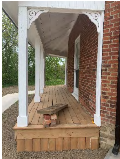
Figure 29: Verandah on the east façade with decorative wood square posts and brackets. The wooden deck level with the top of the fieldstone foundation is a recent addition to the house.
