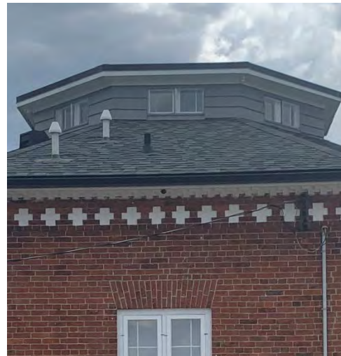
Figure 30: Restored asphalt shingle roofing and new roof vents. Hipped roof lantern has rectangular casement windows and contemporary wood siding as a cladding material.
