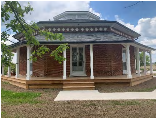
Figure 21: The main elevation (east) of the McClure House shows the original Flemish bond brick and decorative brick white cruciform pattern, wooden dentils, eaves supported by fretwork brackets and wrap around porch (2 elevations). The original French double doors are located in each of the three sides which face the road but, after the alterations in 2019, additional glass panel doors were added in front of the original doors.
