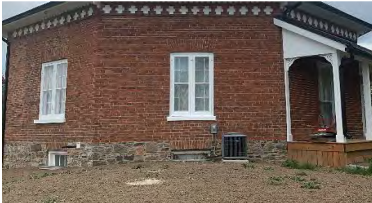
Figure 31: Rectangular windows topped by jack arches. The current replacement windows are double-hung windows with multi-pane sashes.
