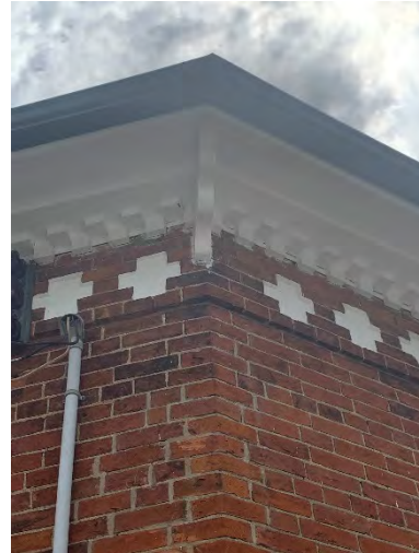
Figure 26: Dentils and a projecting band of decorative brickwork containing a contrasting white brick cruciform motif is present below the eaves.
