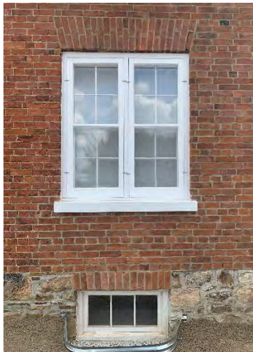
Figure 27: All doors and windows except the basement windows have jack arch heads formed by alternating soldier and rowlock brick voussoirs.
