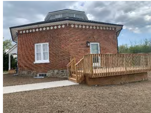
Figure 22: The west elevation of the McClure House building showing the rough fieldstone foundation, restored rear brick wall and the later added pathway and wooden deck.
