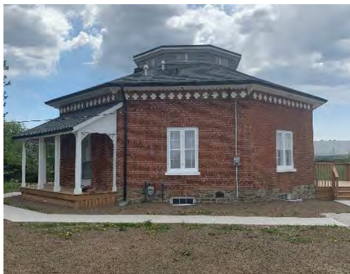
Figure 23: The north elevation of the McClure House building, showing original window openings with new replacement windows and roof drainage accessories. Note the window on the left does not include historic shutters which were present originally (See Figure 19).
