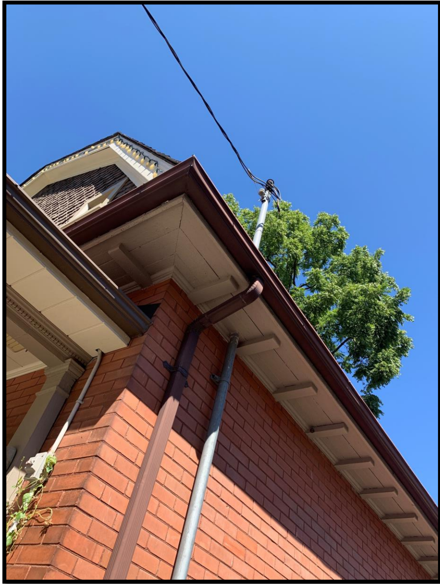
Photo 3: Corner showing cornice with modillion block
