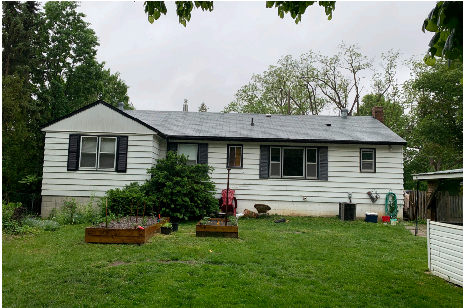
View of Rear (East) Elevation from the backyard. The south end of the house is an early addition to the original 1950's home. The extent of the addition is marked by the left gable end that projects slightly out into the rear yard.
