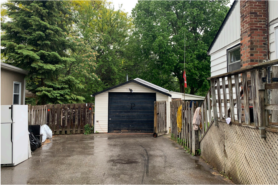
View of the existing detached garage at the end of the driveway. The garage is a 1-storey structure clad with off-white vinyl siding, with a contrasting black door. A wood board fence separates the backyard from the driveway.
