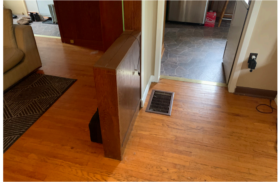
View of the pony wall/shelving unit which separates the dining room and living room. A metal strip marks the transition from vinyl to hardwood flooring, which was carried through the remainder of the main floor.
