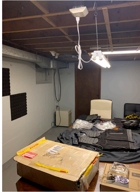
View of basement underneath south addition. Former window in the original foundation wall has been covered. Floor structure above is visible, as ceiling has been left uncovered. The room serves as storage space.
