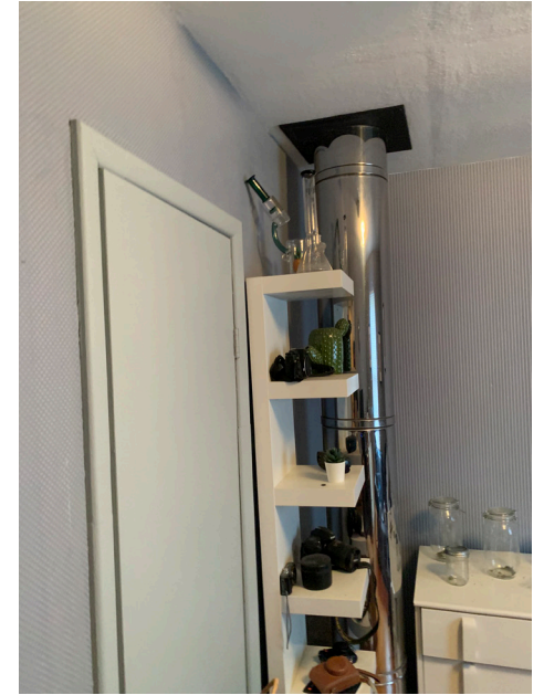
View of the lounge room. There is a chimney flue in the corner of the room that runs from the basement and through the roof.
