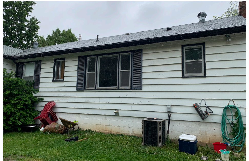
View of Rear (East) Elevation. It is consistent in appearance with the front elevation. Masonry block foundation transitions to white wood overlap siding. Aluminum soffit and asphalt roofing. Black vinyl window shutters are carried over to the back.
