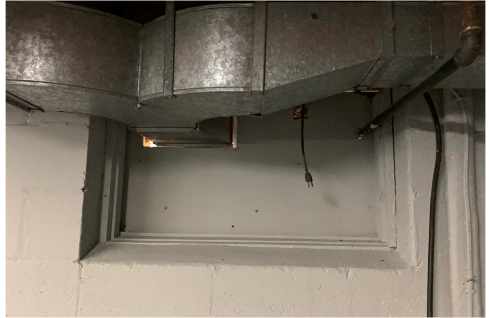
Detailed view of the blocked out window in the original foundation wall. An opening has been cut to allow the mechanical duct to run through.
