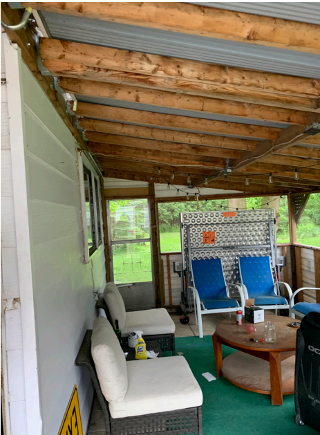
View of the sunroom/screened porch in the outbuilding. Sheltered by an aluminum shed roof with exposed wood framing.
