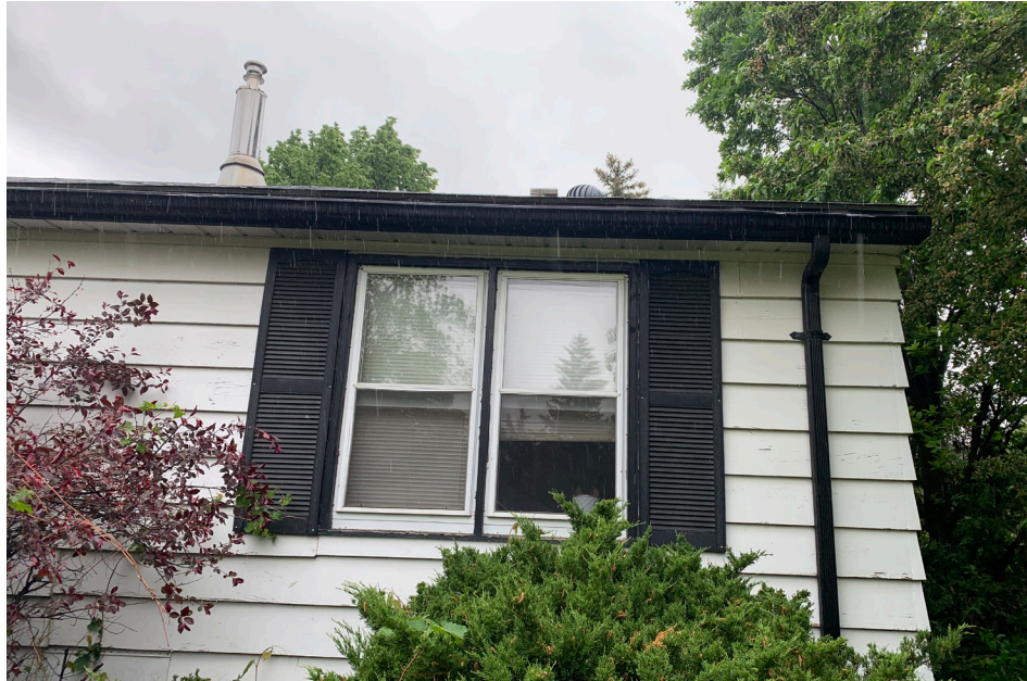
Detailed view of window on Front (West) Elevation. Typical example of the windows all around the facade. White vinyl window with surrounding wood trim. Black shutters and window trim are in contrast to the white siding.
