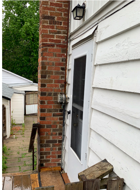
Detailed view of side entry. Note the difference in brick along the height of the chimney stack, which transitions from a smooth to rough texture, suggesting an extension to or repairs to the chimney.
