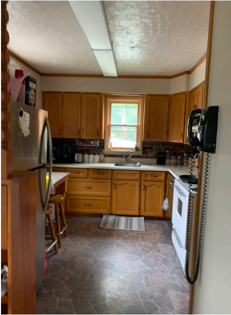
View of the kitchen looking across the room towards the backyard. Walls and ceiling are both of drywall construction. The floor is finished with a stone textured vinyl. Wood trims run along the ceiling and doorways.
