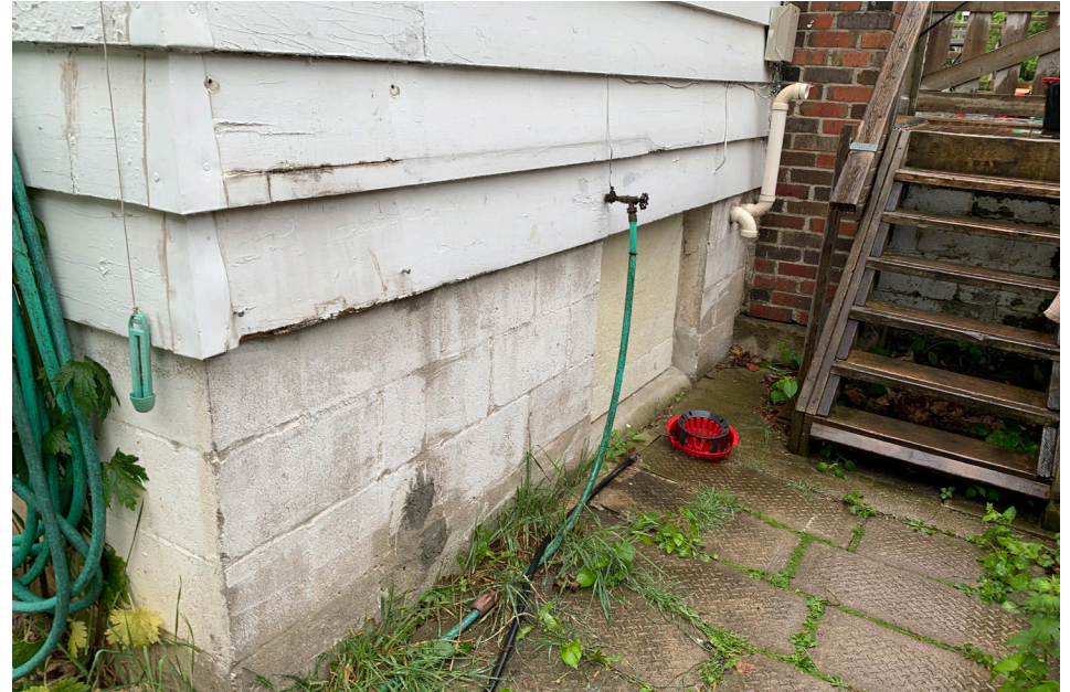
Detailed view of the foundation along the North Elevation. The foundation of the house is masonry block. The basement window has been covered up. The wood deck at the front of the house connects to the rear yard, with a wood staircase that leads down to a small paved area.
