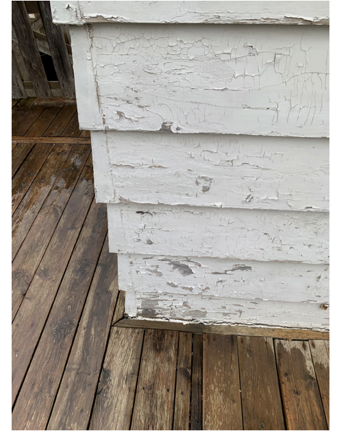
Front Facade Detail. Paint is peeling from the wood siding in places all along the facade. House is in need of maintenance.
