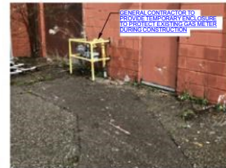
12 GAS METER TO REMAIN
