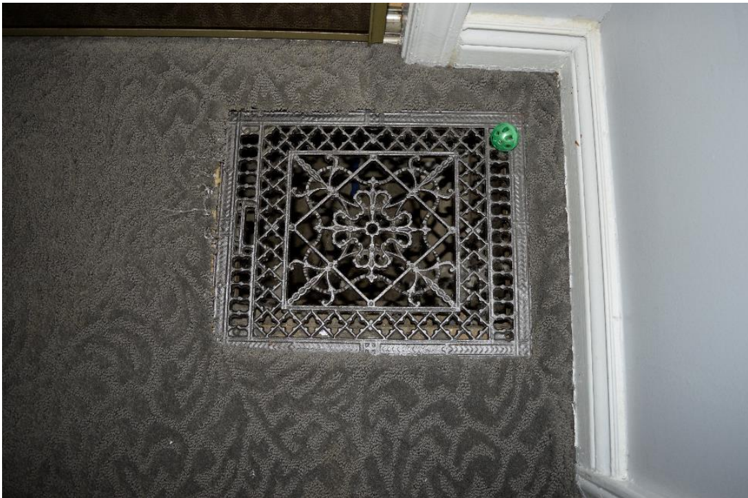
Image 68: Example of original floor grate
