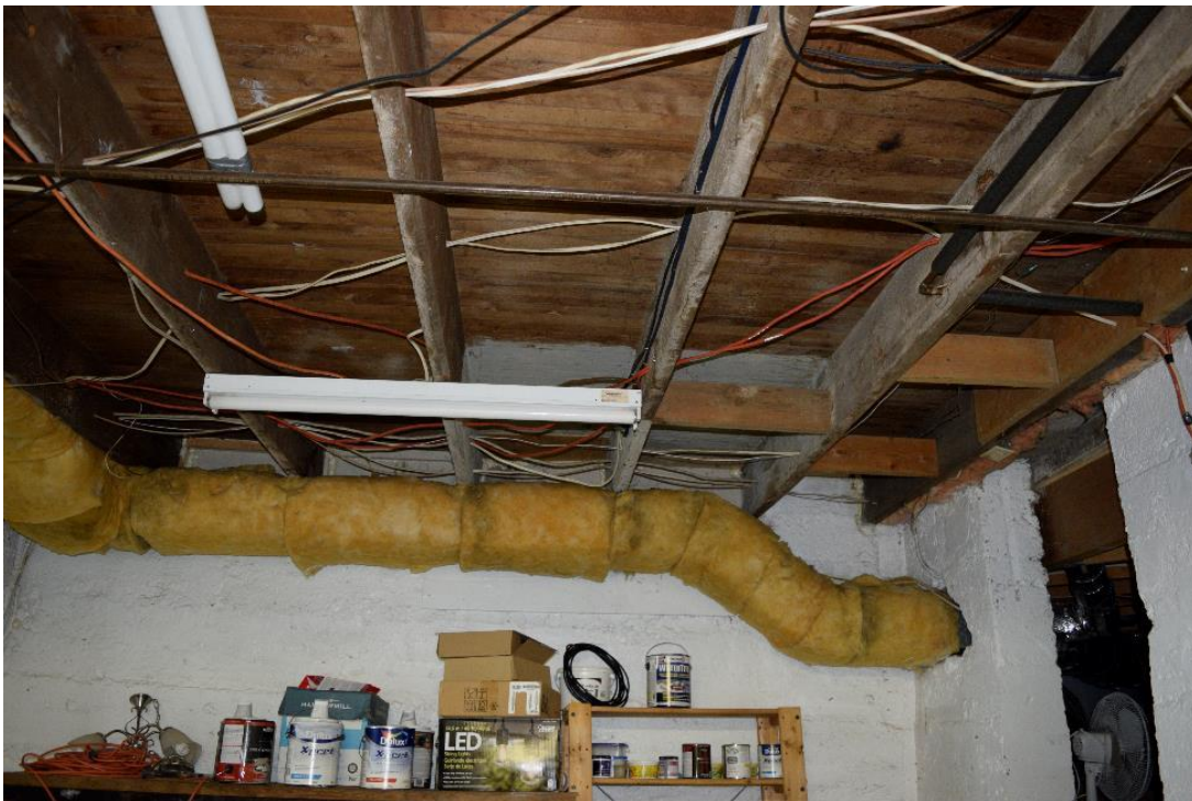
Image 64: Typical floor joists and subfloor
