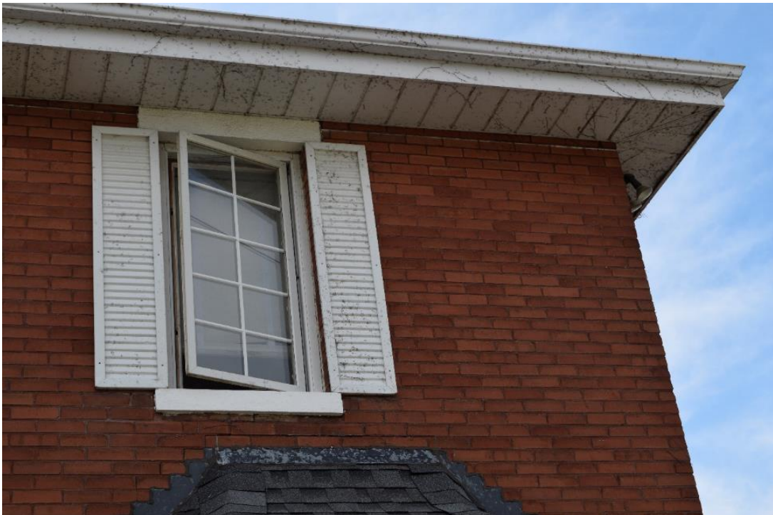
Image 44: Typical window, note cast lug sill and oversized lintel. Facia and soffit has been clad in aluminum.
