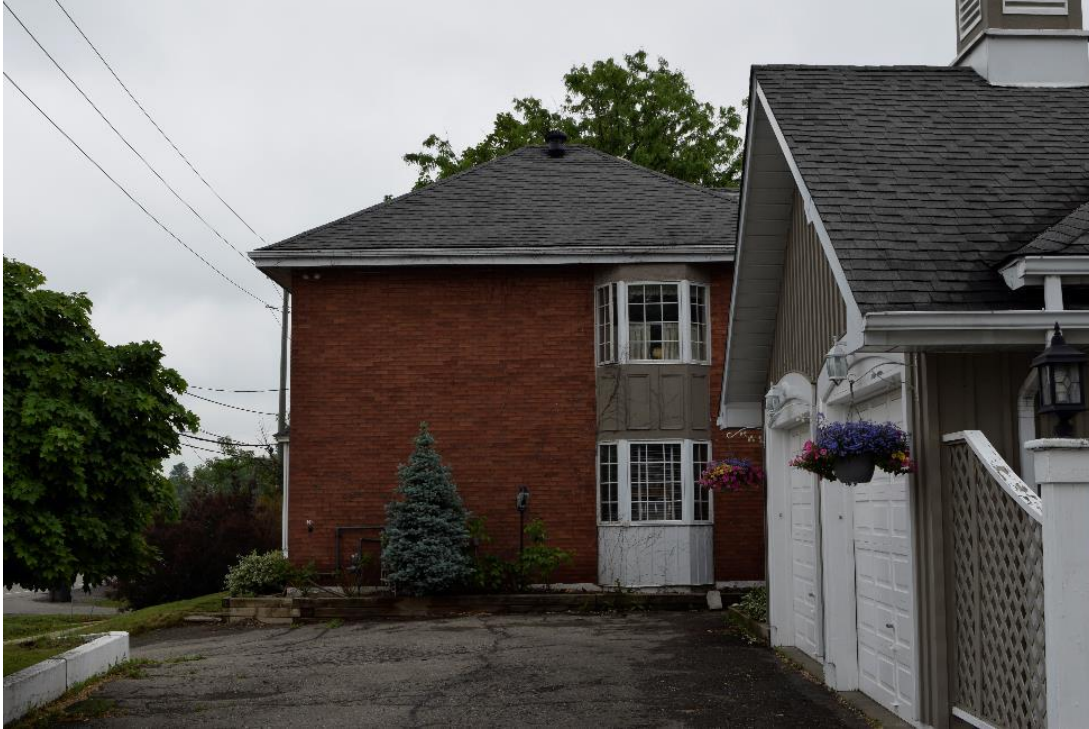
Image 41: two story bay, non original, brick has been cut to accommodate it.
