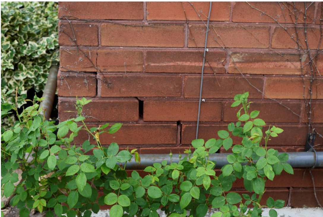
Image 40: Evidence of foundation settling as observe on northwest corner of structure.
