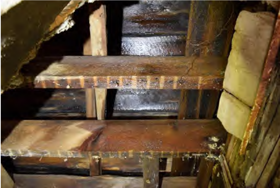
Image 65: Water damage associated with roof structure.
