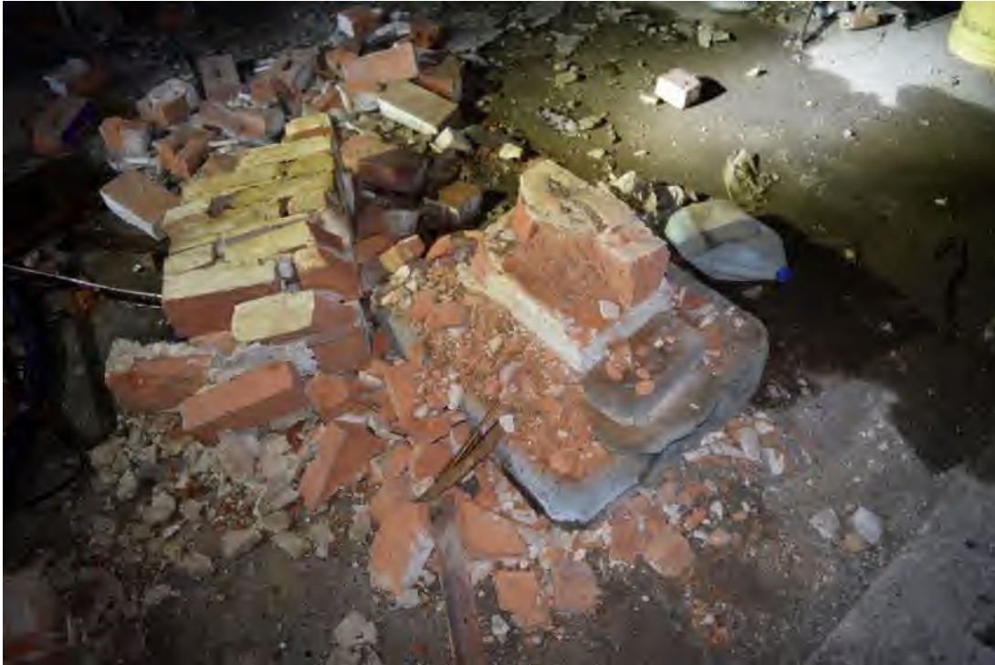
Image 52: Remains of brick support column in northern half of basement.
