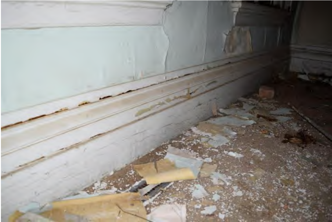
Image 54: Example of original baseboard present in southeast room, first floor.
