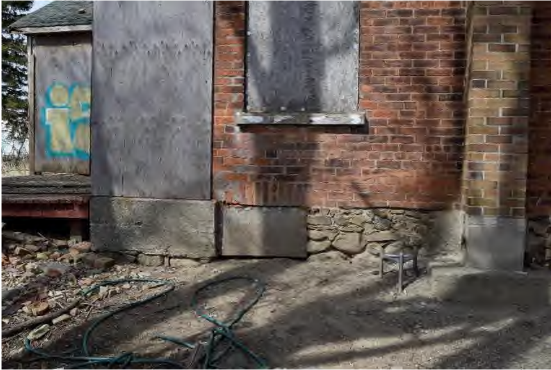
Image 29: Past foundation repair on southwest corner of structure, plywood is covering extensive delamination of exterior brick.
