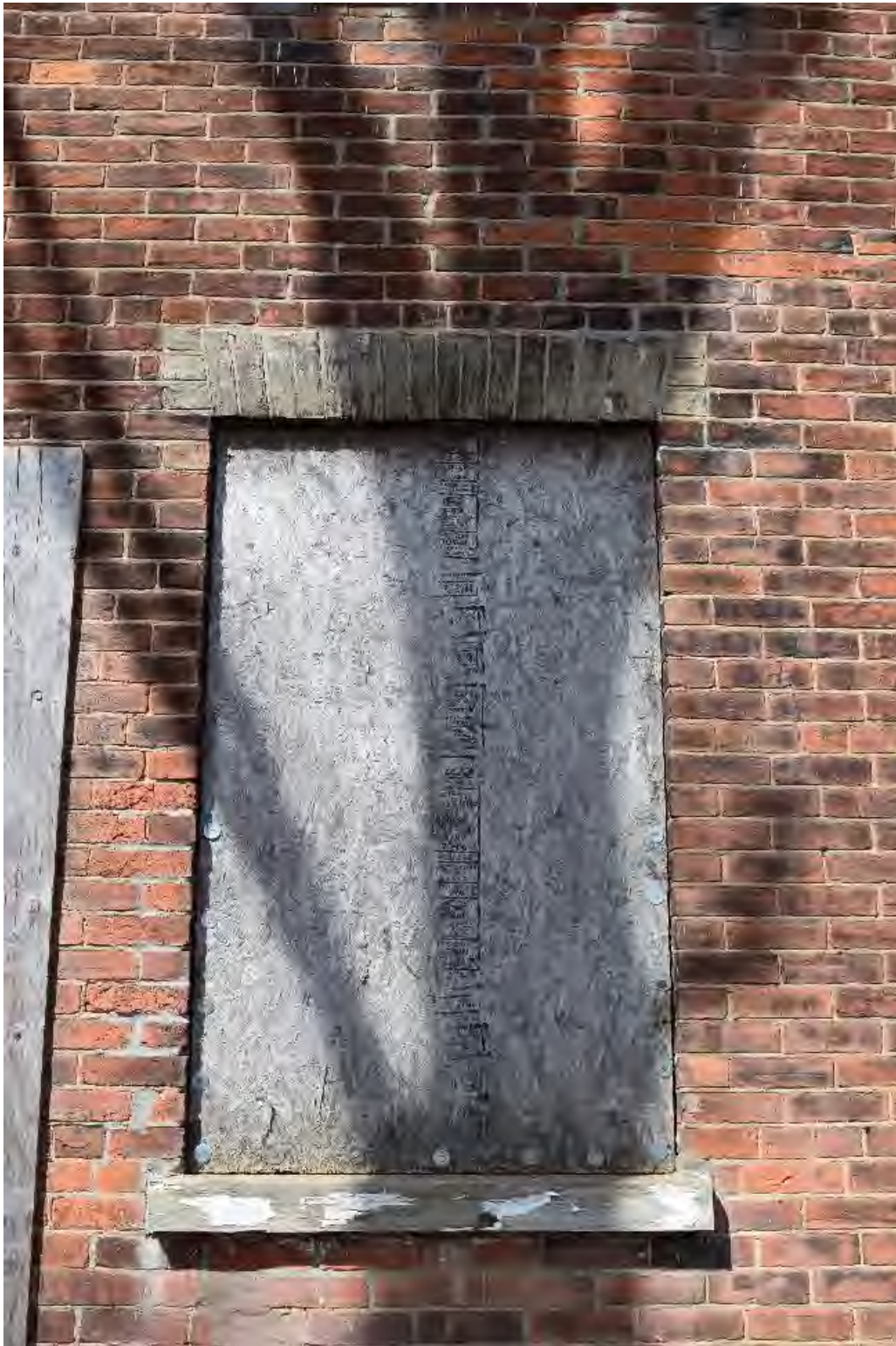
Image 20: Typical window opening on south and west of faces of structure, note use of decorative voussoir but lack of label.
