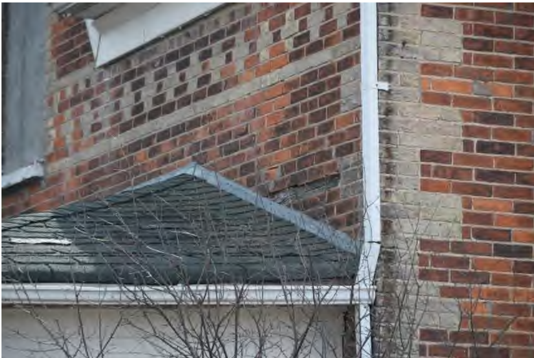
Image 24: Connection between brick structure and front veranda, note presence of wooden ledger set into brick work.
