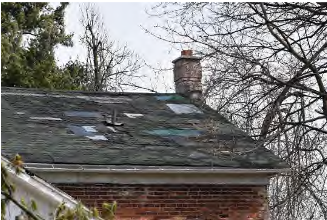
Image 28: Roof damage resulting in degradation of underlying structure, note non-original chimney.
