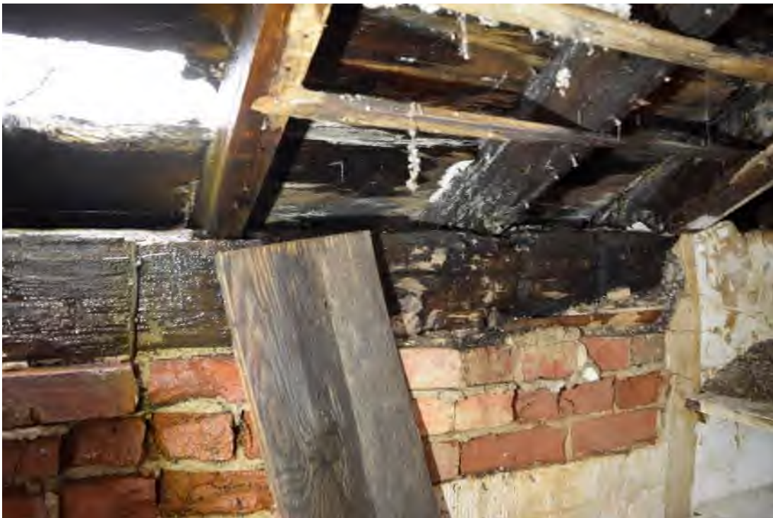
Image 64: Extensive water damage typical of that associated with roof structure.
