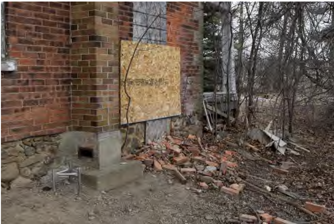
Image 30: Plywood covering structural damage associated with southeast corner of structure.
