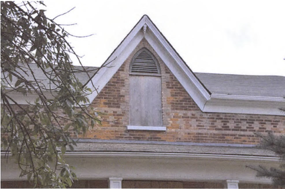
Centre Gable With Finial and Decorative Brickwork
