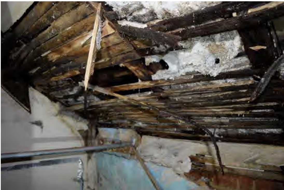
Image 66: Typical condition of ceiling damage on second floor.
