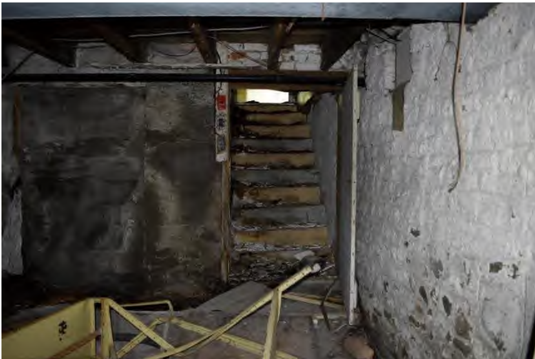
Image 51: Access stairs to basement, note concrete infill to left of steps, facing west.
