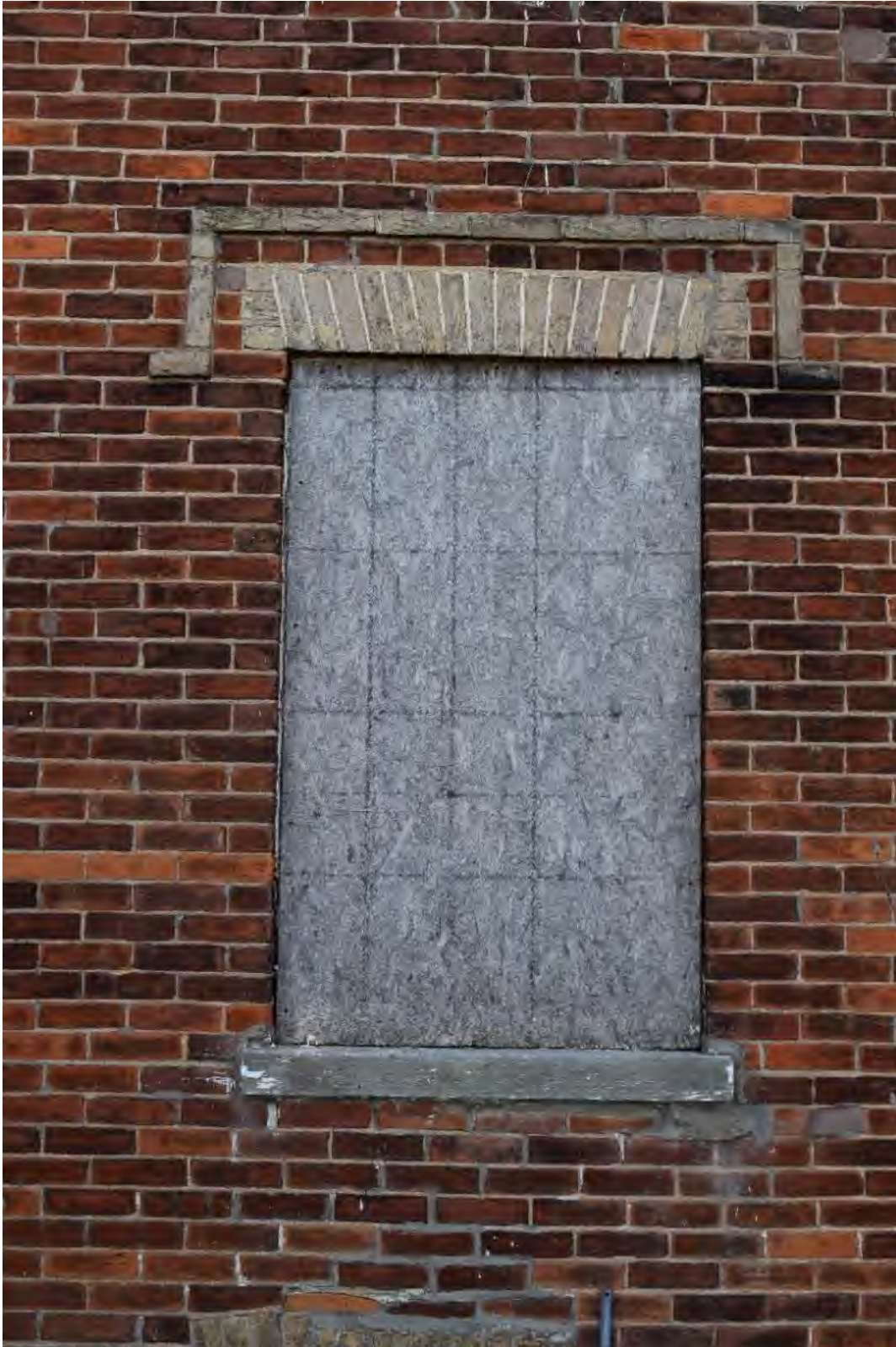
Image 19: Typical window opening on north and east of structure, note decorative voussoirs and associated upper label.
