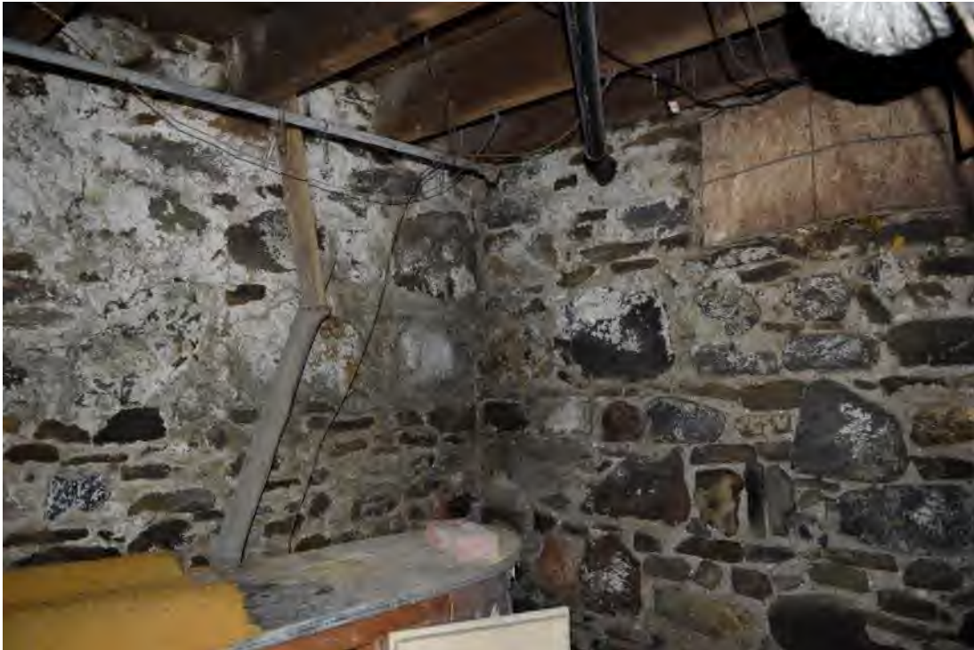
Image 49: Interior of field stone foundation, south half of structure.
