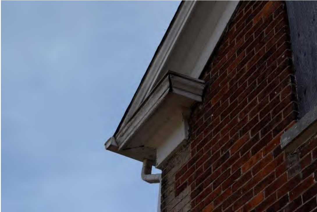
Image 23: Cornice return, present on all corners of the structure.
