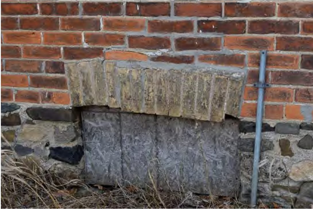
Image 25: Typical voussoir associated with basement windows, note past repair attempts.
