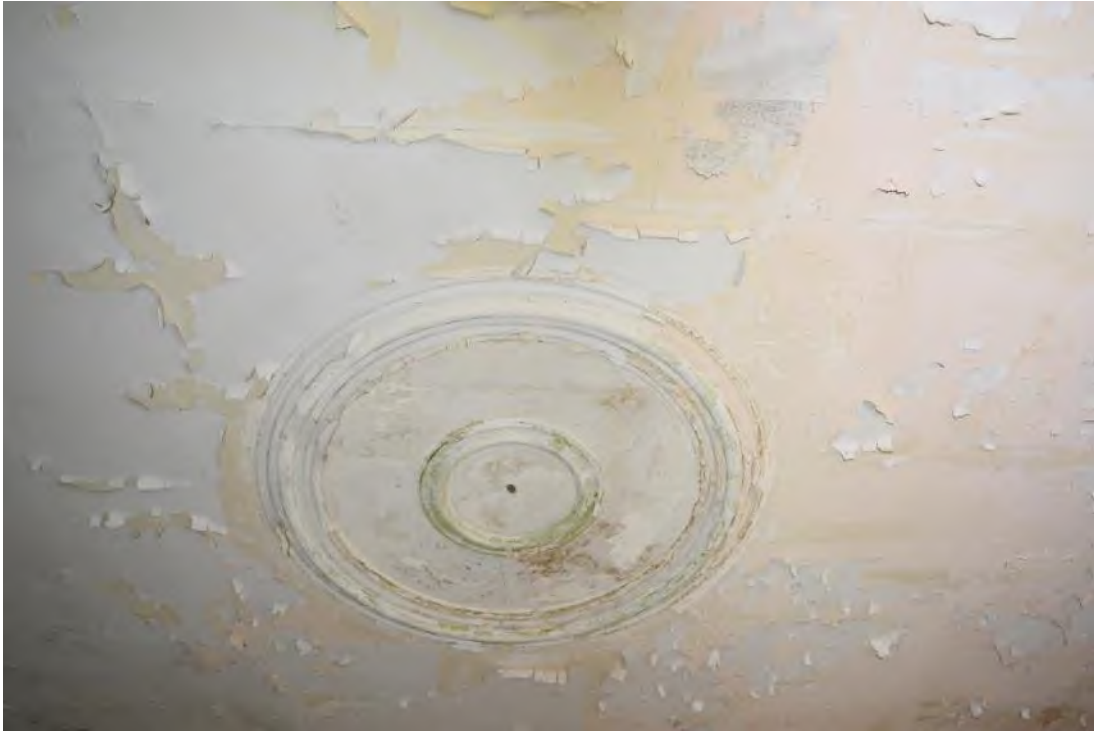
Image 61: Plaster ceiling medallion in southeast room, first floor.
