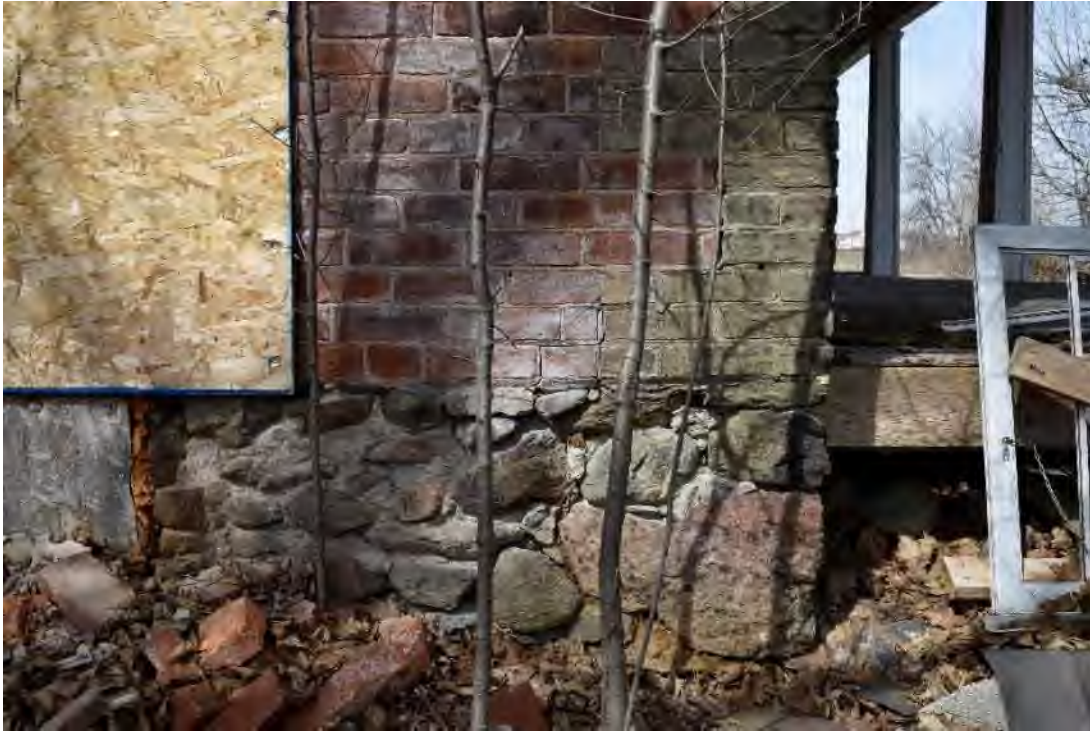
Image 17: Closeup of field stone foundation, southeast corner of structure
