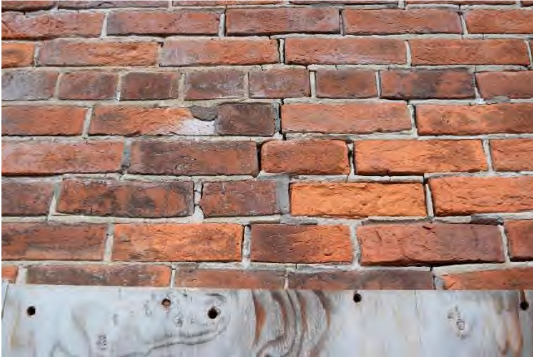
Image 27: Close up of brick damage, typical of that seen on structure.
