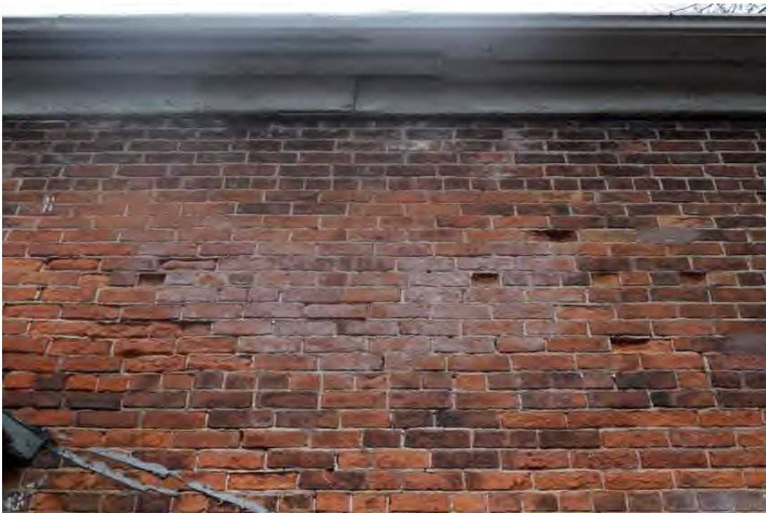
Image 26: Extensive water damage to brick on west face of structure, damage also visible to the wooden soffit and frieze.
