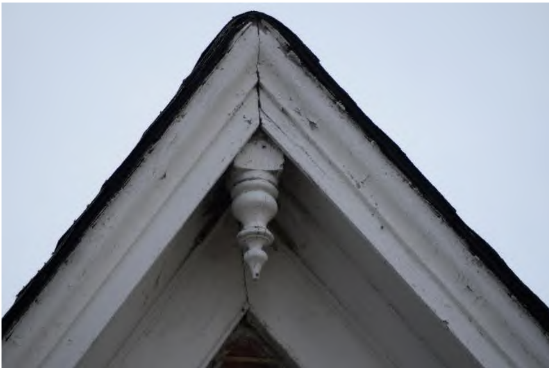
Image 22: Moulded fascia frieze and soffit with drop pendent in central gable dormer.
