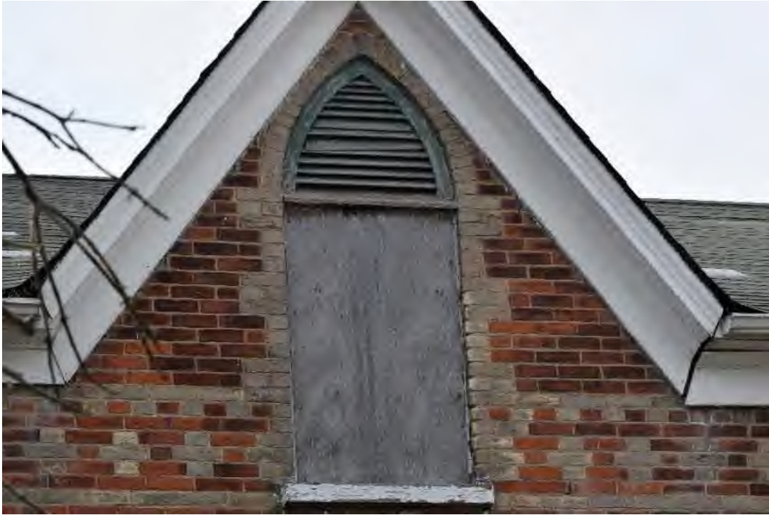
Image 21: Pointed window in central gable dormer, note dichromatic brickwork.
