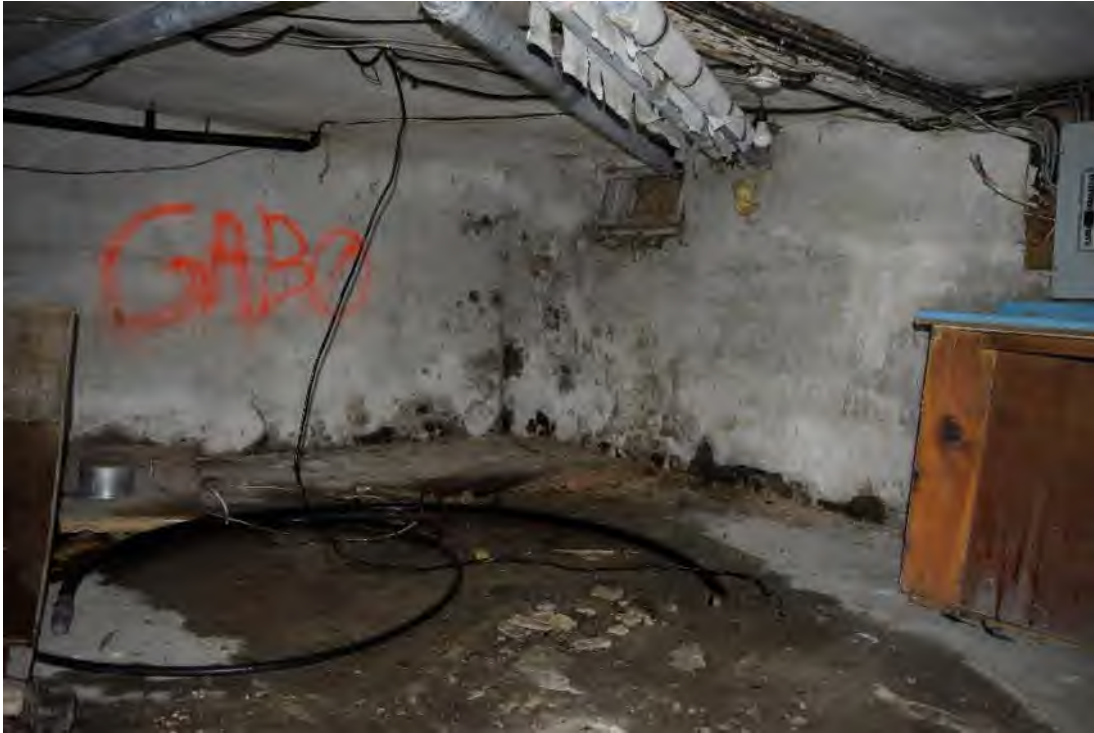
Image 50: Limewashed interior of north half of basement.
