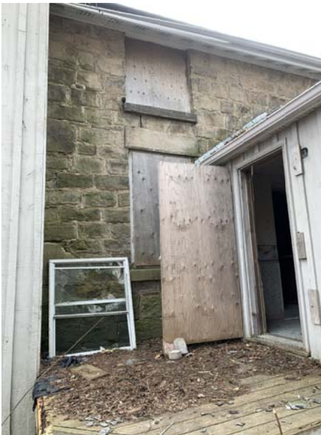
Figure 14: Stone sill and lintel to be restored
