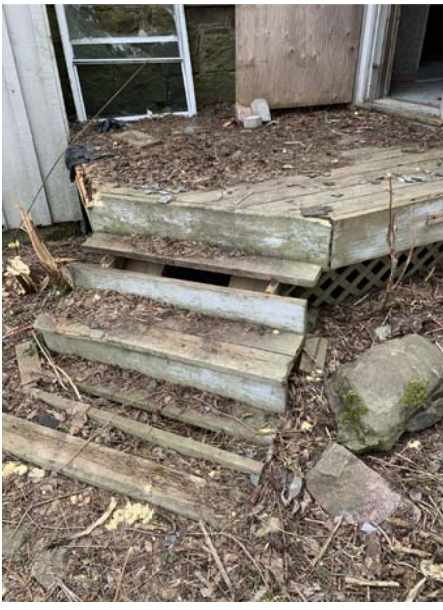
Figure 14: North porch entry steps to be removed & replaced
