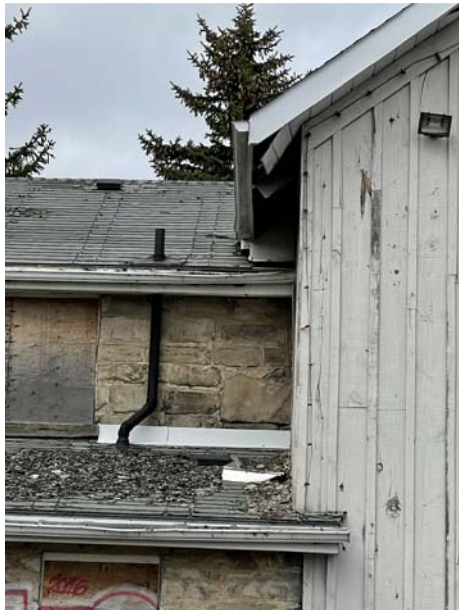
Figure 16: Roof accessories to be replaced
