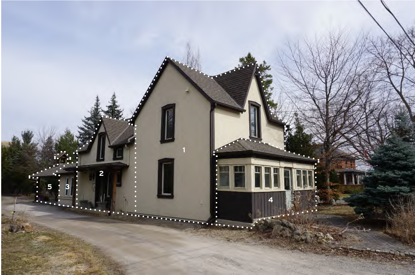
Phasing of construction - 1) Original 2-storey house, 2) First addition, 3) Second addition, 4) Enclosed Porch, 5) Outdoor Sitting Area. Source: ATA, 2021.
