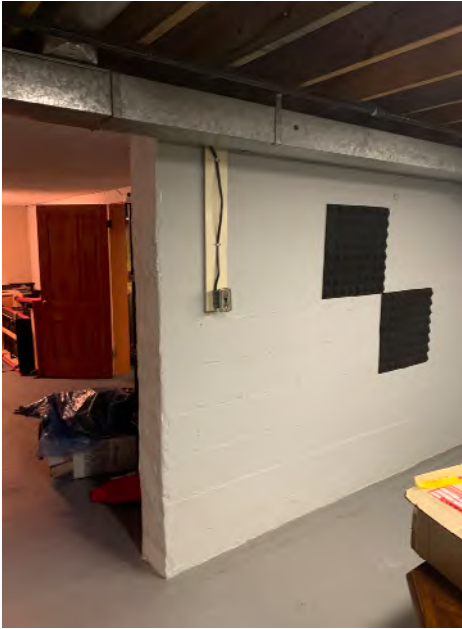
View of masonry block foundation wall of the original footprint. Doorway has been cut into the foundation walls and plastered over.
