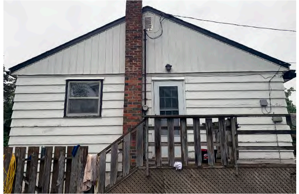
View of North Elevation. A low pitched side gable profile. The house is clad with a combination of wood overlap siding up to the underside of the roof and vinyl siding in the gable. A brick chimney stack is located to the east of the side entrance door, which is also accessed from the raised wood deck.
