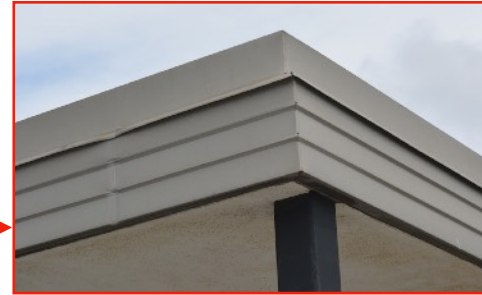
Close-up of a corner of the canopy, showing seam details of the metal flashing. Note the damage on the left
