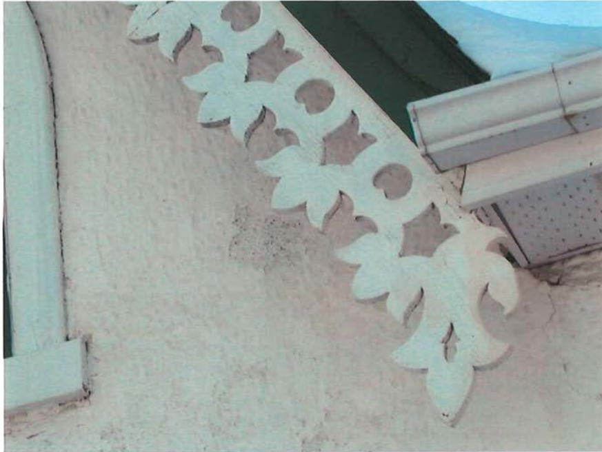
Figure 4: Detail of decorative vergeboard on front gabled wall dormer.
