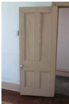
Figure 25 -Cracks in Interior Door
