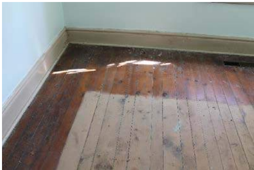
Figure 21 - Discoloration on Hardwood Flooring
