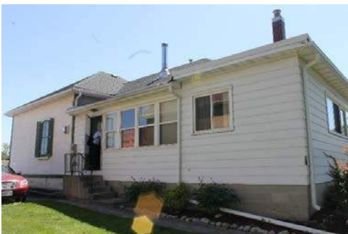
Figure 38 - "EII" Addition as seen on North Elevation clad in metal siding
