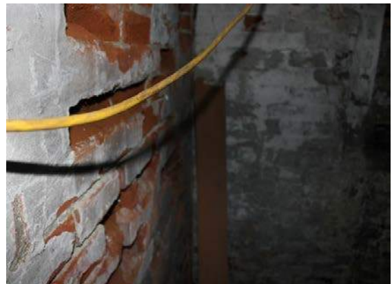
Figure 45 - Missing Brick Features in Foundation Wall facing north
