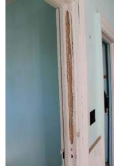
Figure 24 - Cracks & Peeling on Wood Door Frame
