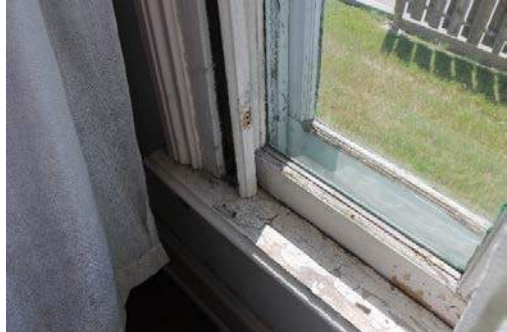
Figure 23 - Chipped & Decayed Window Sills & Frames
