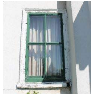
Figure 29 - Peeling Paint on Window Frame
