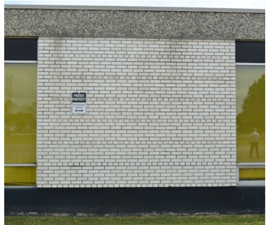
Example of brick panel on the main (west) elevation. Dirt from water damage is noticeable at the top and will be cleaned. The signage post will be removed and mortar patched.
