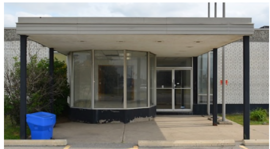
Close-up of main entrance with the display case, double door and canopy supported by steel columns, which will all be replaced with new reproductions.
