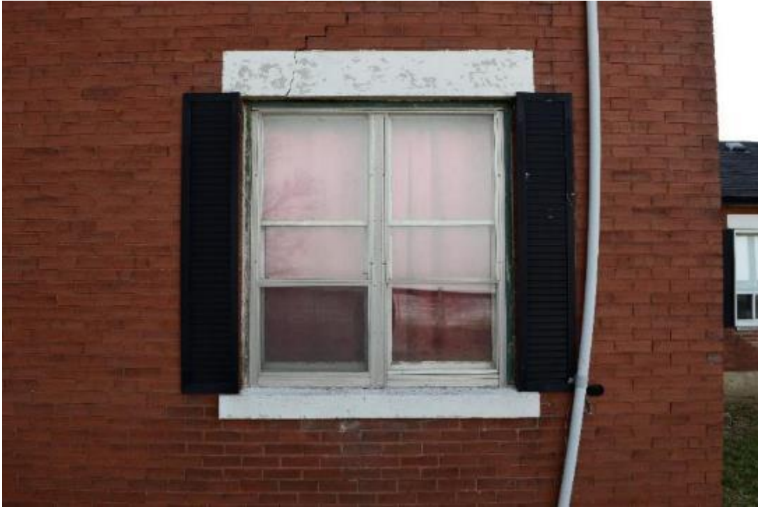
Image 18: Typical original window with later external aluminum storm. Note crack in brick and cement lintel. Southwest corner.
