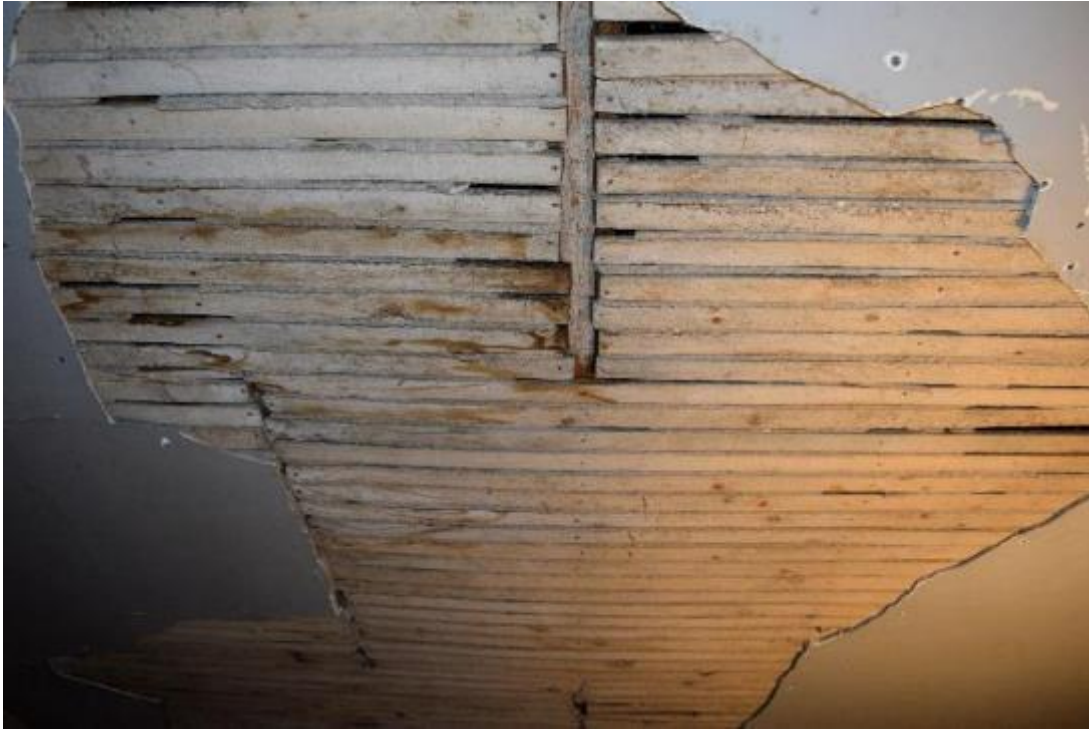
Image 38: Exposed cut lath, typical of that used in wall and ceiling construction.
