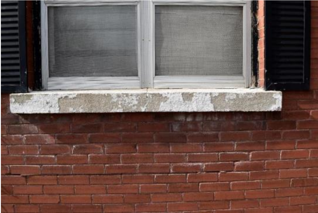
Image 24: Water damage and settlement associated with windows on front façade. Note crack in sill and staining indicative of water damage on brick under sill.
