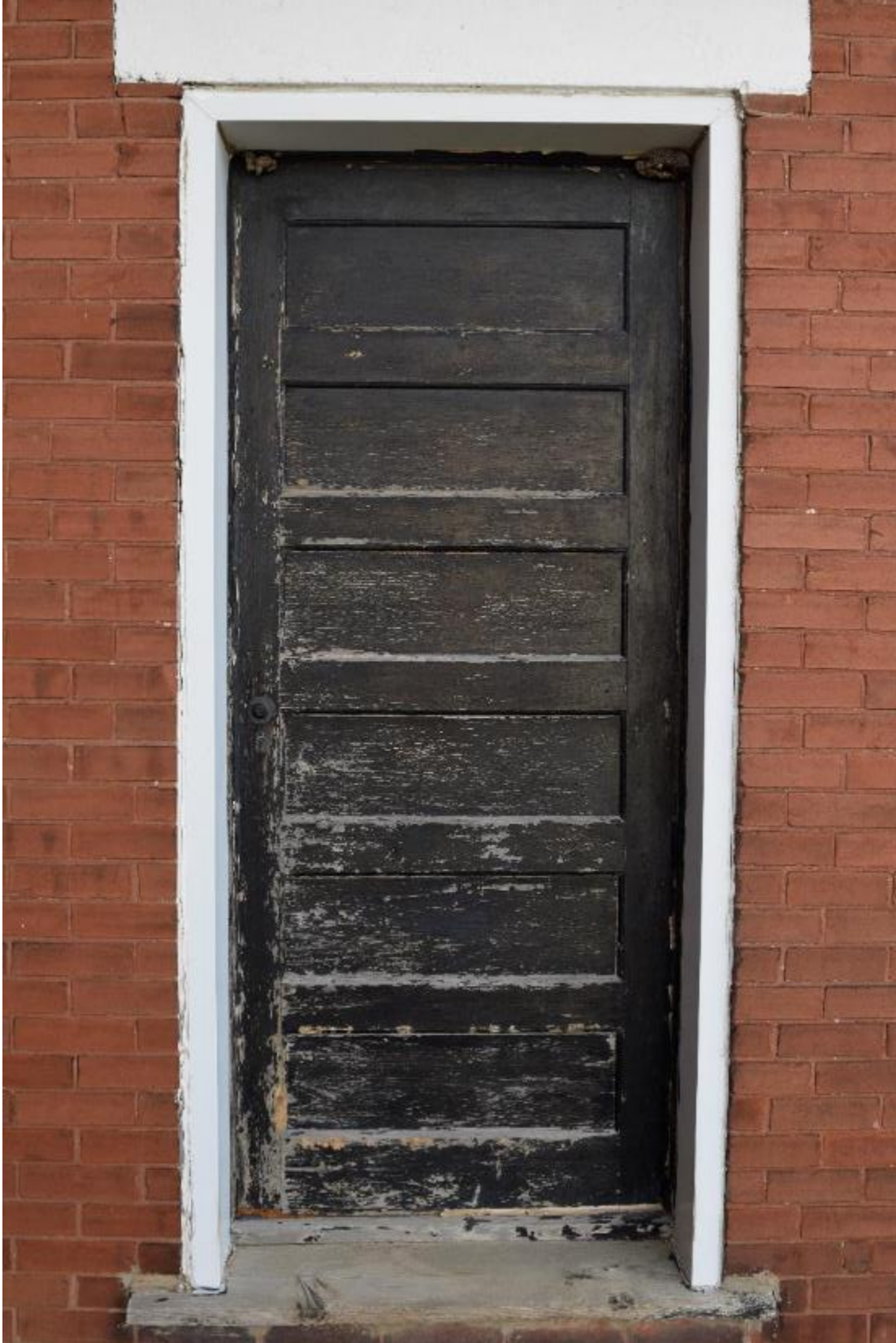
Image 30: Typical six panel non-operable door of rear addition.
