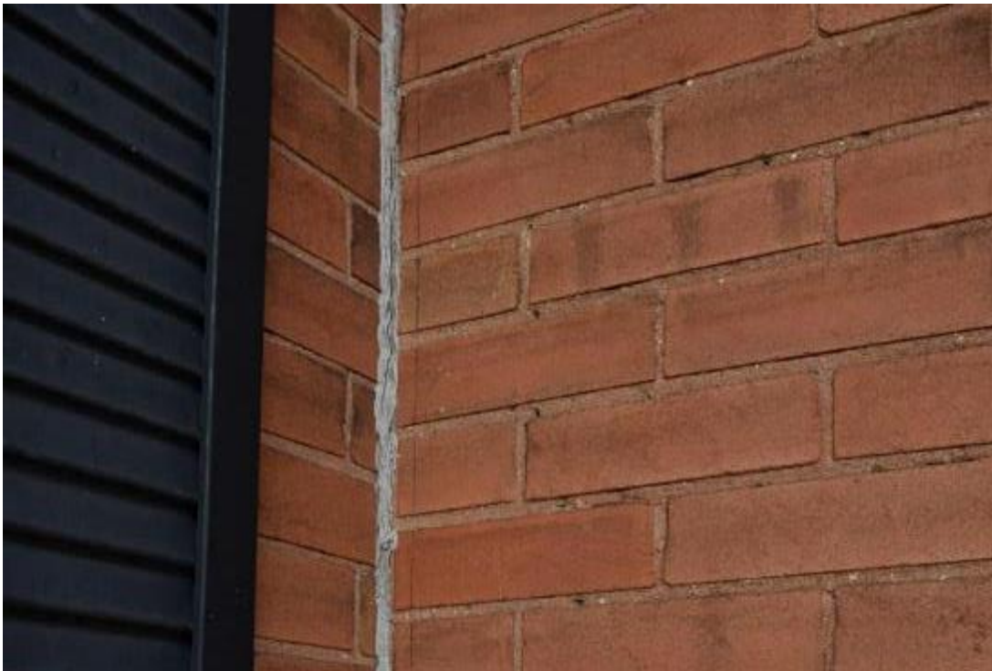
Image 25: Seam between main house and rear addition, brick courses do not align.
