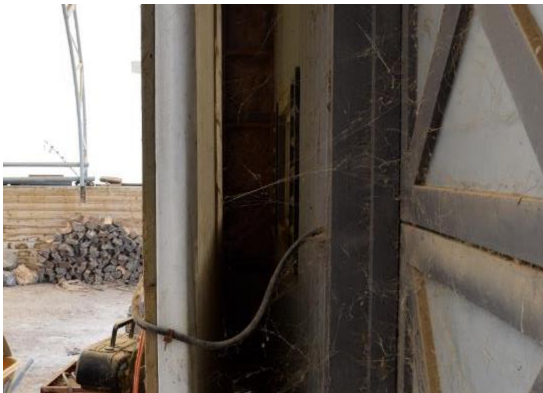
Image 108: Separation between fabric Quonset hut and 1998 horse stable.
