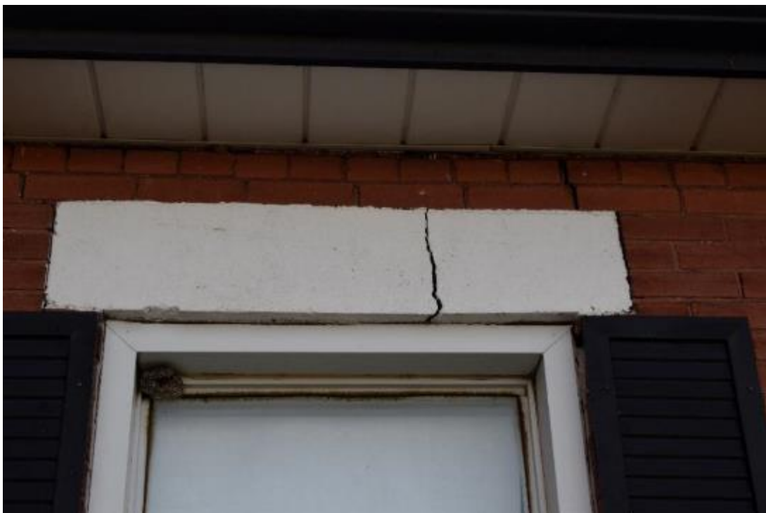
Image 19: Structural damage to second storey cast concrete lintel. This damage is typical of structural openings.
