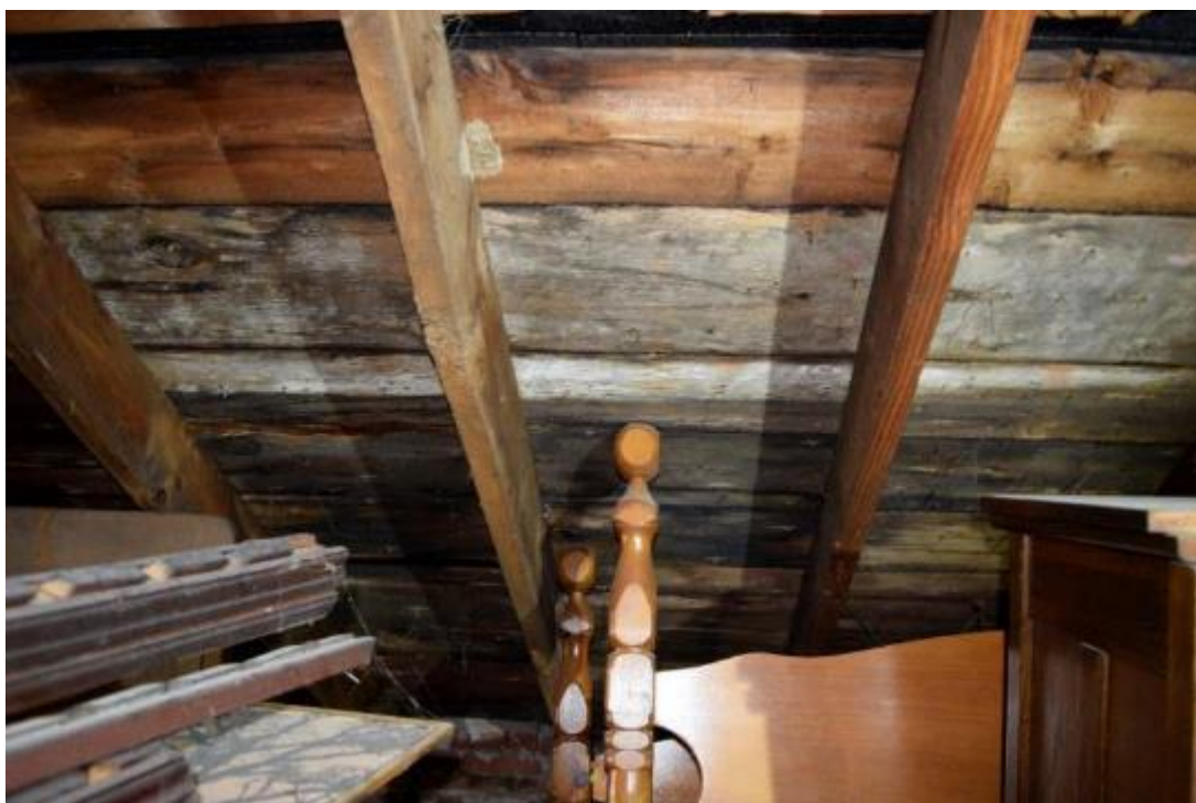
Image 62: Example of discolouration of roof decking indicative of water infiltration.
