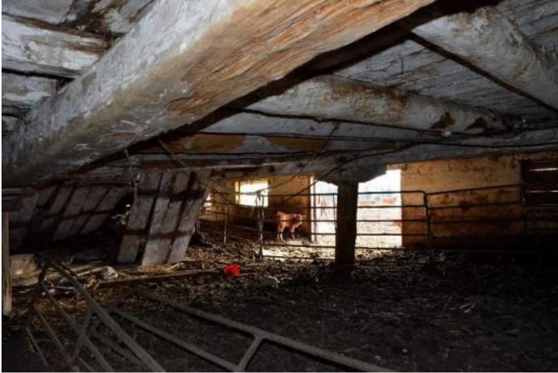
Image 93: Lower level of timber frame barn, suffering from structural collapse.
