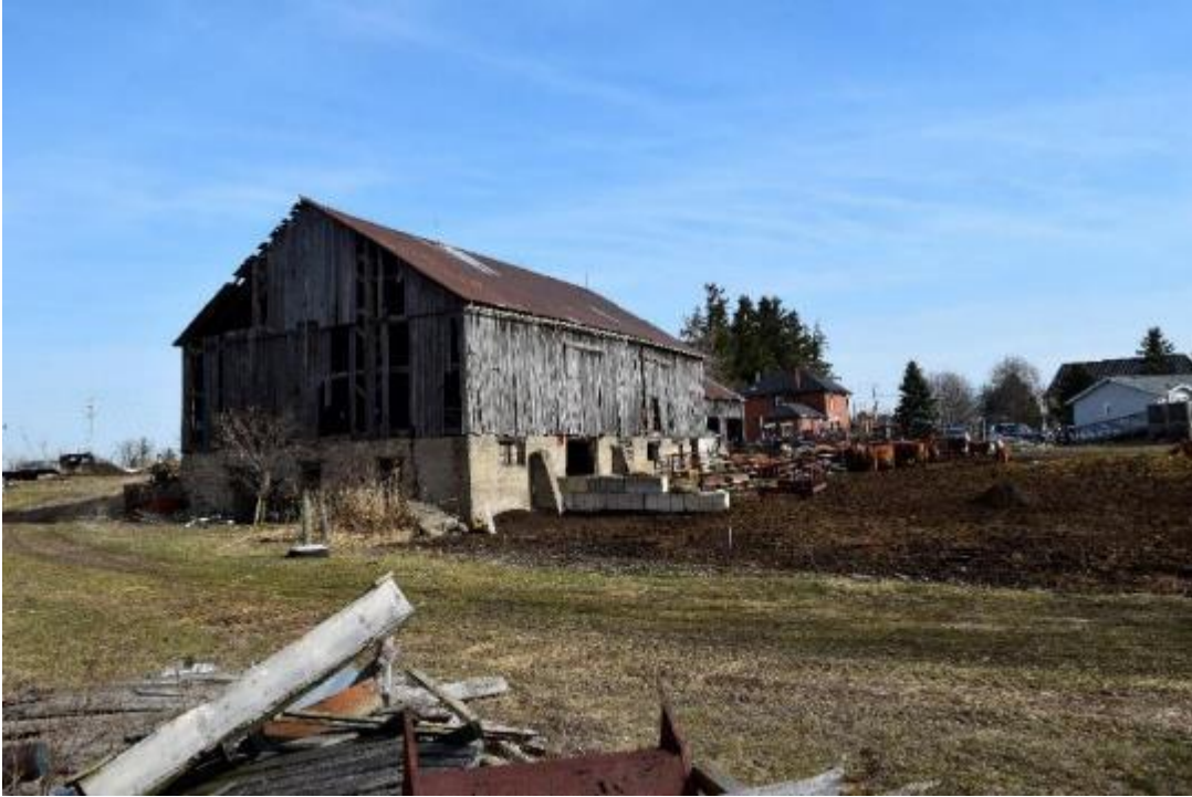
Image 87: Timber frame barn with field stone foundation and later concrete repair and buttress, facing north.
