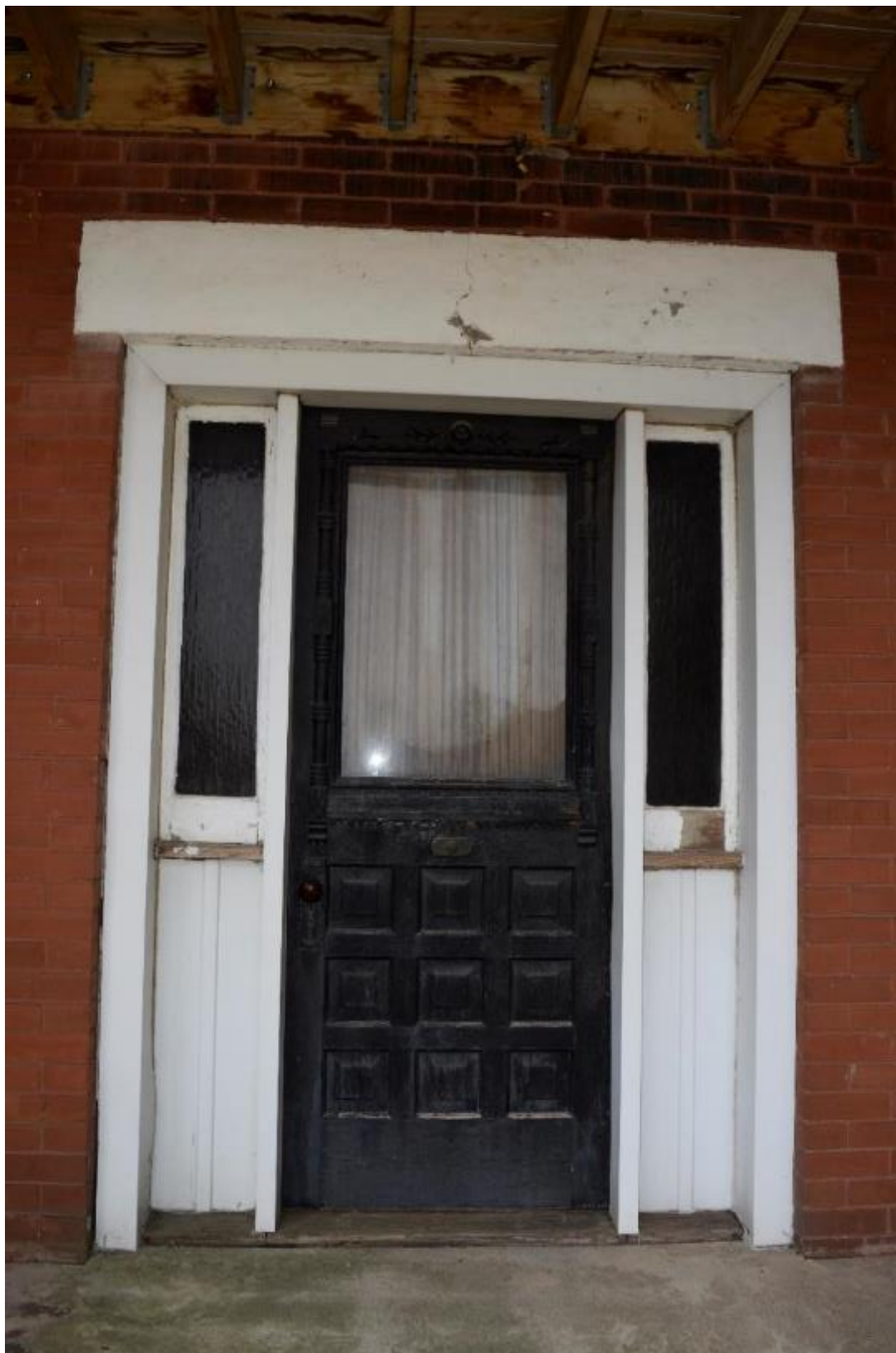
Image 21: Front door and sidelights. Note split in concrete lintel.
