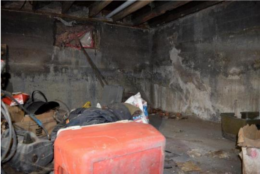
Image 69: Poured concrete foundation in northwest corner of home, note extent of water staining indicating seasonal flooding of basement. Light colour represents high water mark.
