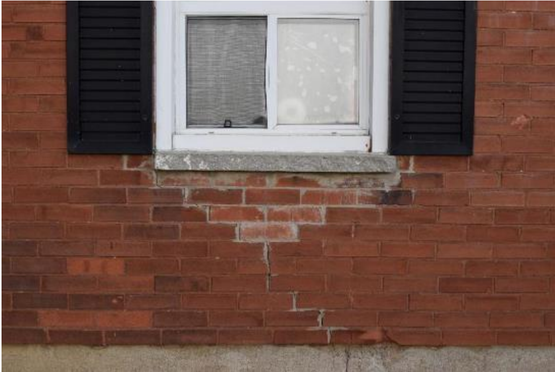
Image 22: Typical repair of damage to structural openings, Note use of new sill material and crack continuing into foundation.
