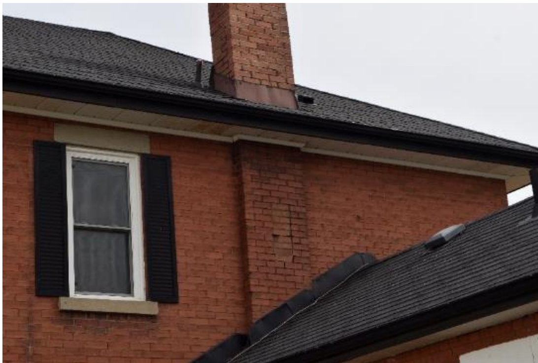
Image 28: Damage to and repair of extant chimney. Note rust streaks on soffit indicating underlying water damage.
