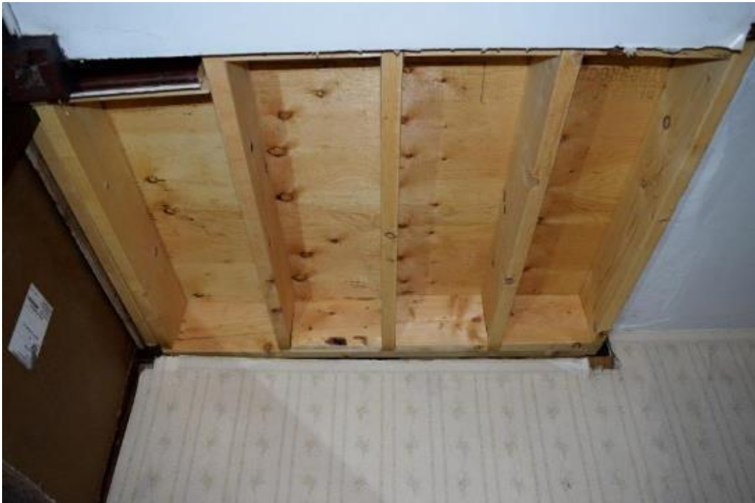
Image 43: Exposed framing installed when main stairs were removed.
