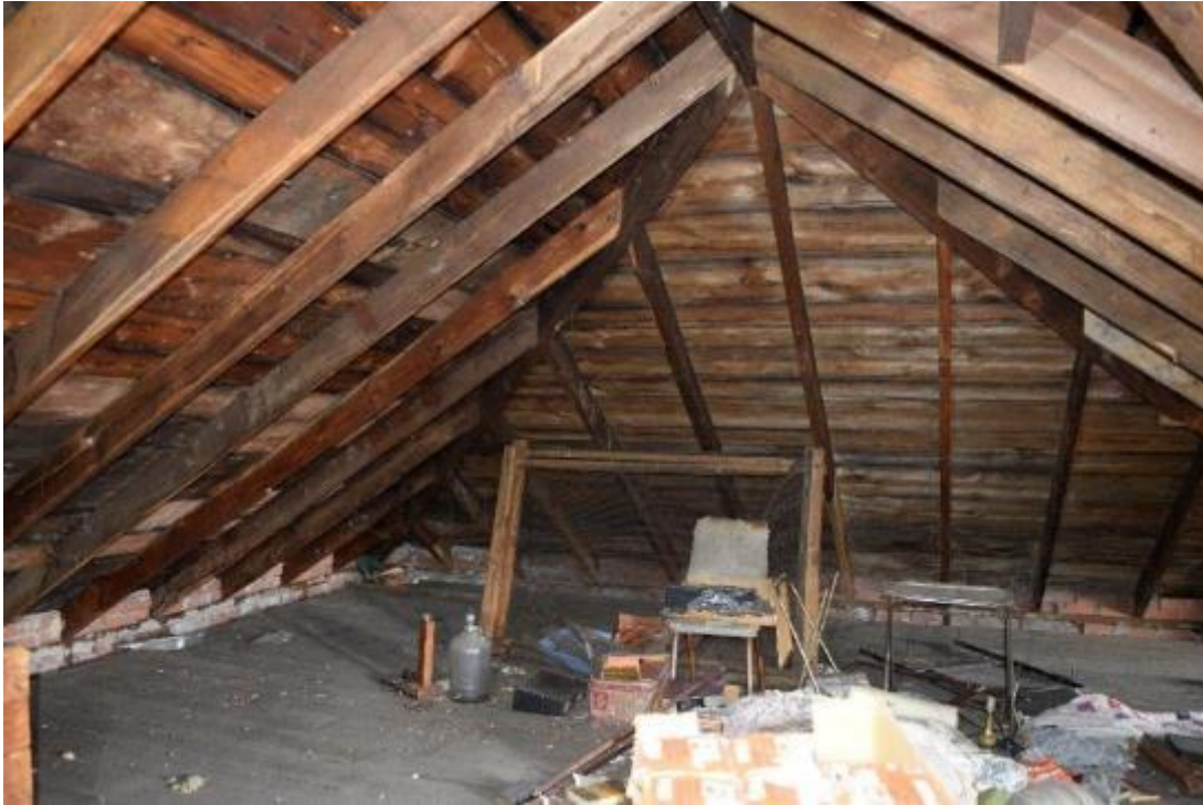
Image 59: Attic space with exposed rafters and roof boards.
