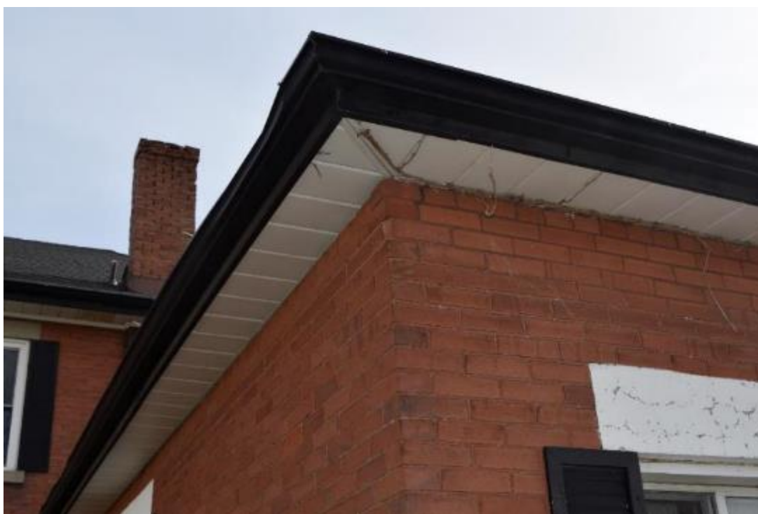
Image 29: Typical aluminum fascia, soffit and eavestrough. Note chimney in left quadrant of image.
