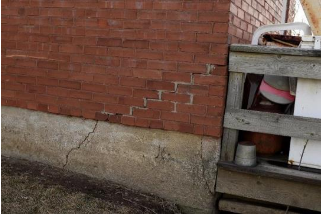
Image 26: Cracks in cement foundation continuing into brick veneer of rear addition.
