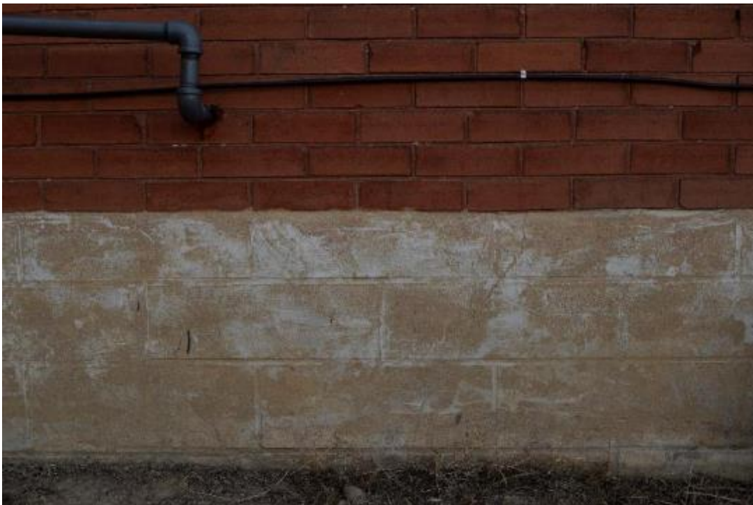
Image 23: Tooled finish of poured concrete foundation.
