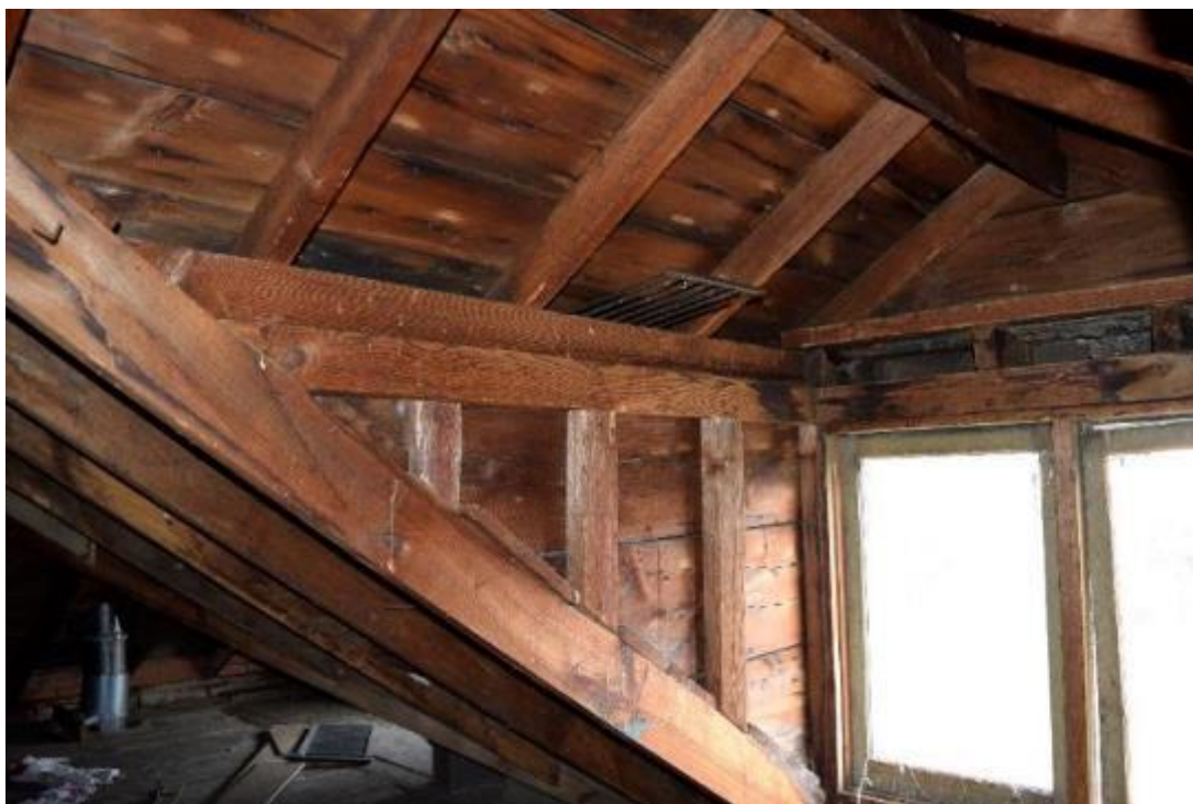
Image 61: Center gable dormer with original wood one light casement windows.
