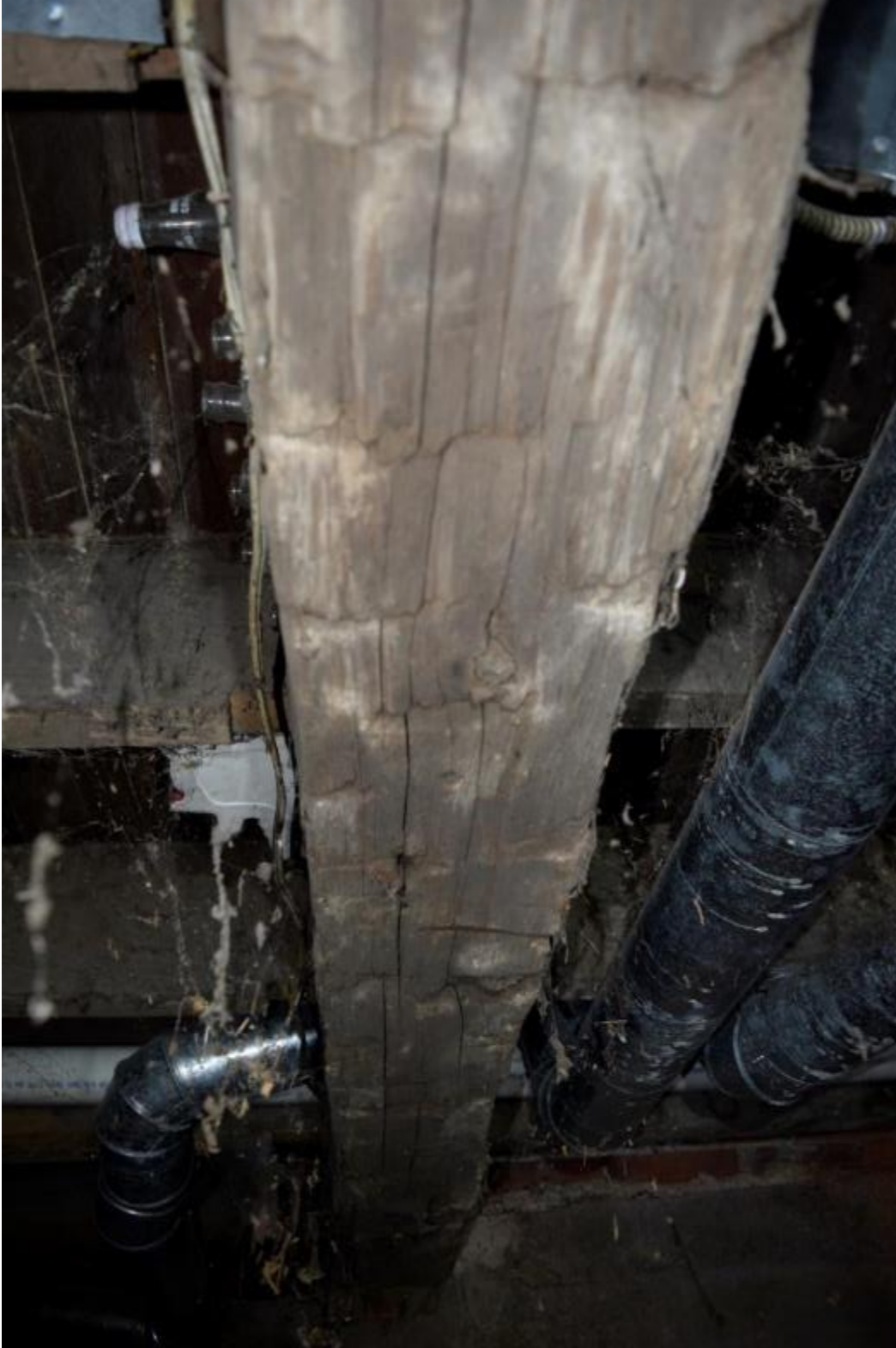
Image 71: Example of hand-hewn support beam, likely an example of repurposed salvaged material.
