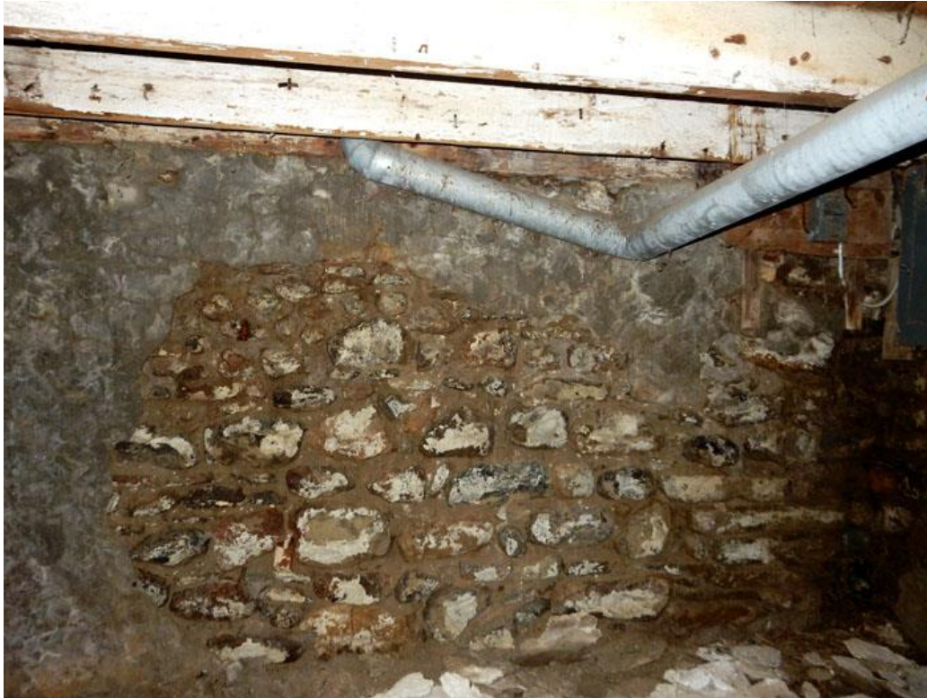
Fig. 22 – Basement Rubble Stone Wall
