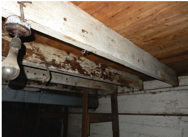
Figure 28: Basement Post & Beam Construction, LDW
