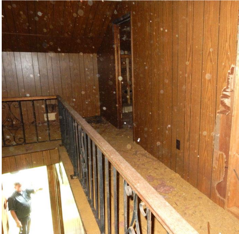
Fig. 26 – Second Floor Landing from Staircase, Beaverboard Cladding
