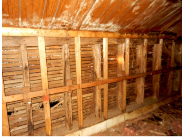
Figure 24: Sawn Lath under Modern Framing in Upstairs Space, LDW
