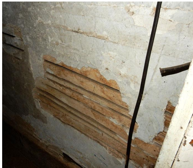
Figure 23: Hand Split Lath at Entrance to Basement, LDW
