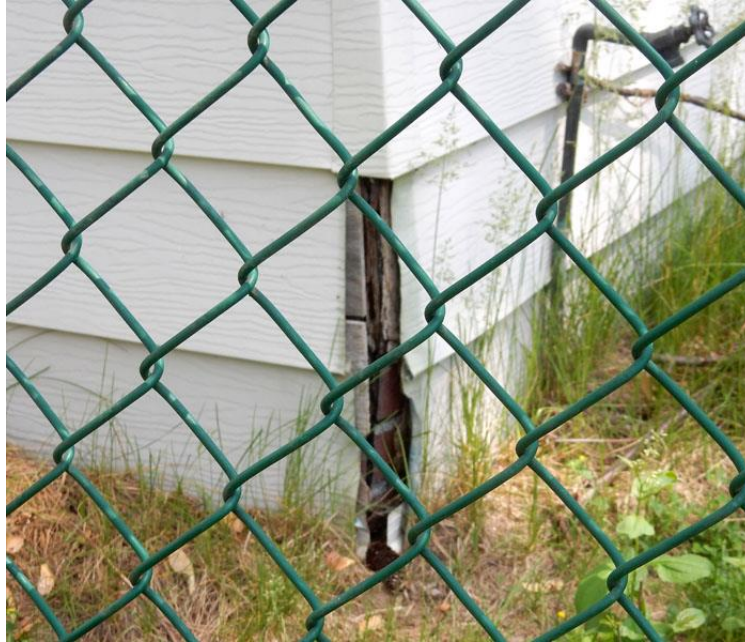
Figure 18: Elliott House, Detail, Insullbrick & Possible Clapboard Cladding
