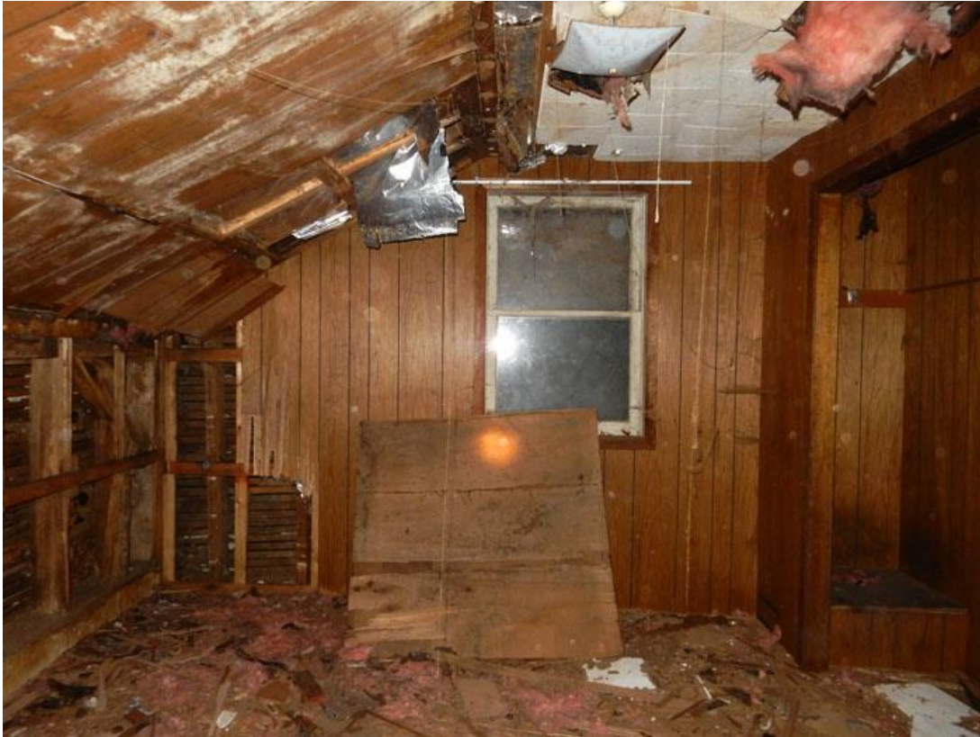
Fig. 25 – Second Floor Beaver Board Cladding
