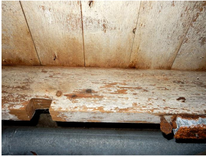
Figure 27: Basement with Post & Beam Construction & Main Floor Pine Flooring, LDW
