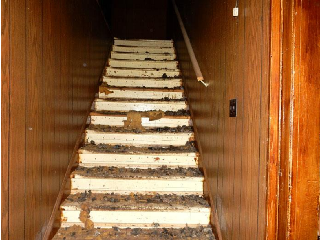
Fig. 9 – Interior, Entrance Vestibule with Boxed Staircase and Beaverboard Walls
