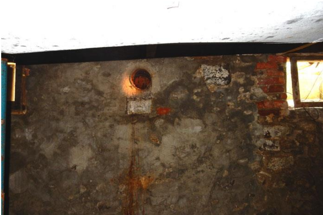
Fig. 18 – Basement Rubble Stone Foundation Walls with Stove Hole
