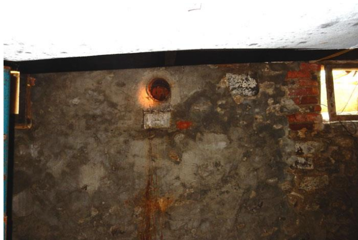
Figure 26: Stove Hole in Rubble Stone Basement, LDW
