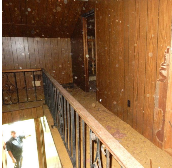
Figure 29: Second Floor Hallway with Beaver Board Walls, LDW
