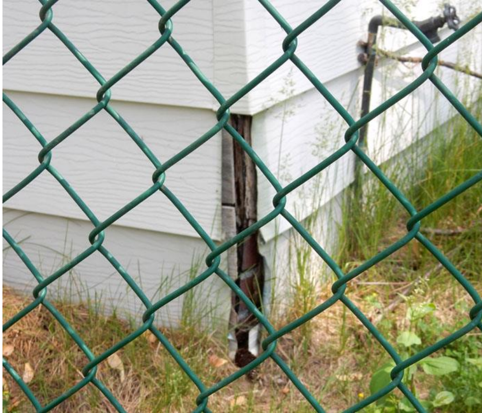
Fig. 8 – Detail, Insulbrick and Vinyl Siding
