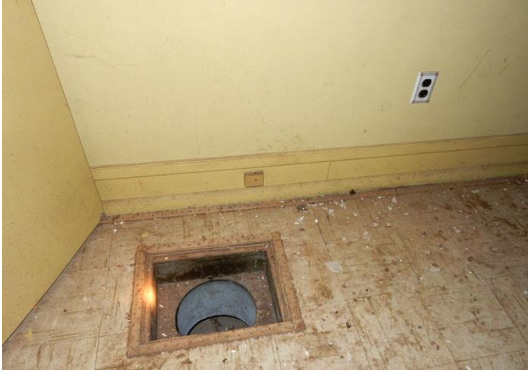
Fig. 12, Chase for Stove Flue Pipe
