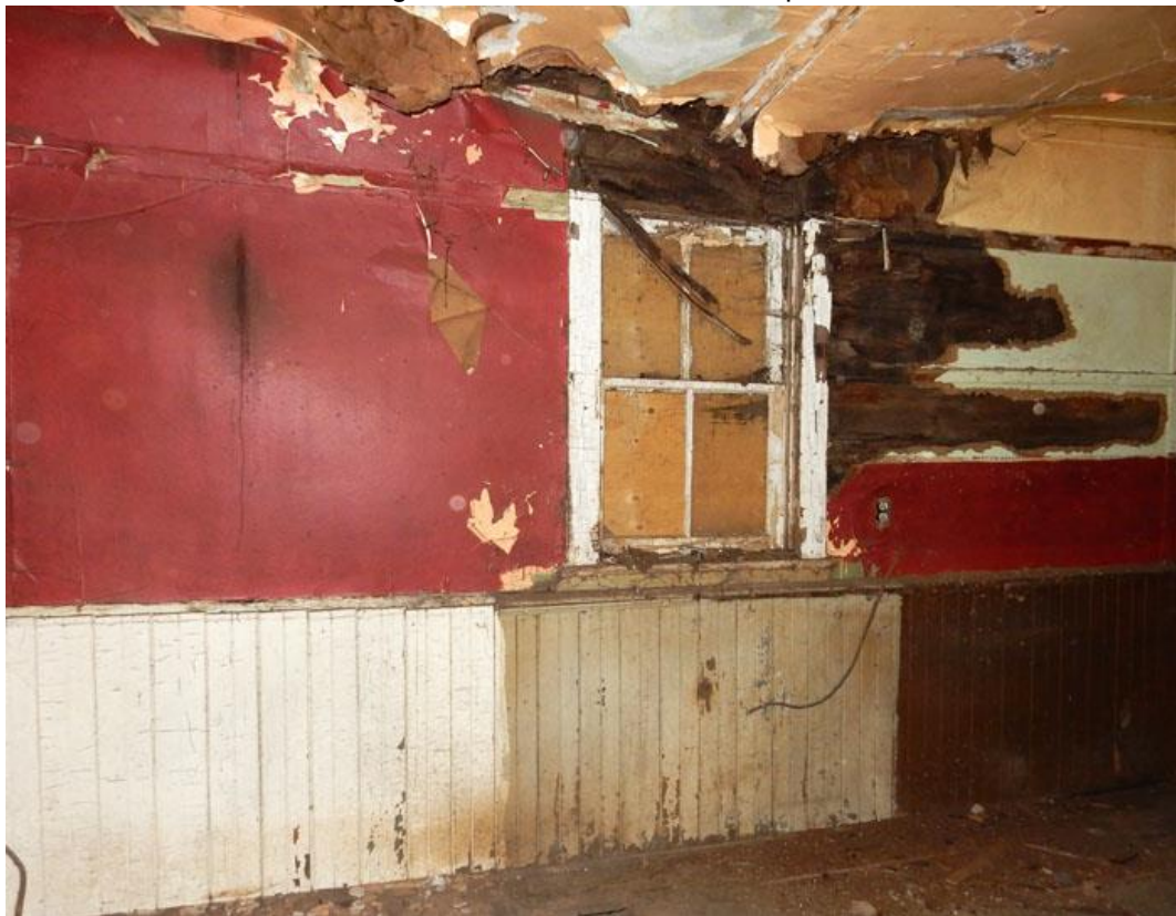
Fig. 13 – Rear of House, Wainscoting in Possible Kitchen Area
