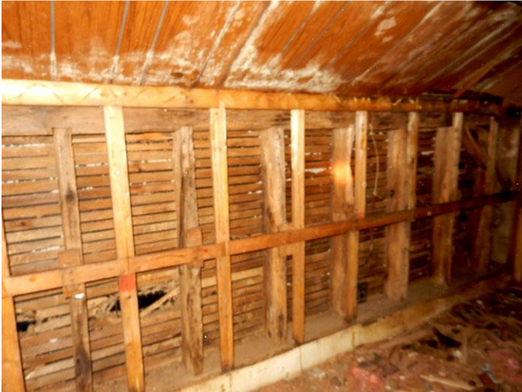
Fig. 24 – Second Floor – Sawn Lath and Posts
