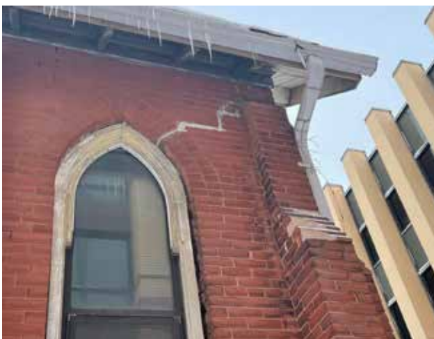
Fig. 5.15. Typical condition at window openings: structural cracks and incompatible repairs.
