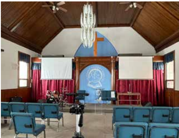
Fig. 5.23. Main floor interior, wood paneling and ceiling are in good condition. Floors are covered in carpet.
