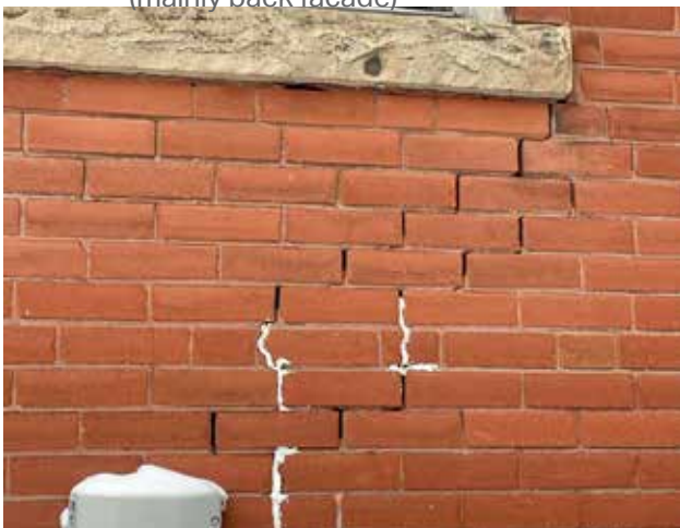
Fig. 5.3. General condition of brick throughout, displaying signs of deterioration, structural cracks, open joints and incompatible repairs.
