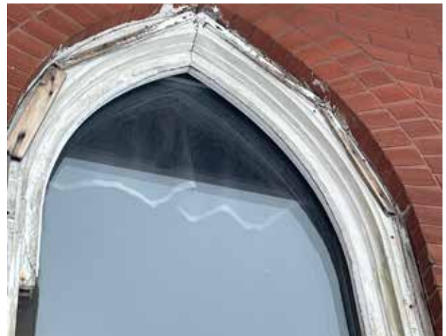
Fig. 5.17. Original wood window frames in fair to poor condition. Windows have been replaced.
