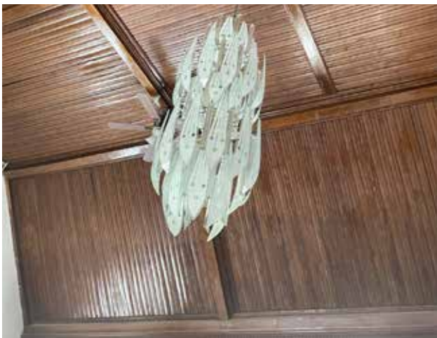
Fig. 5.24. Wood ceiling appears to be in good condition.
