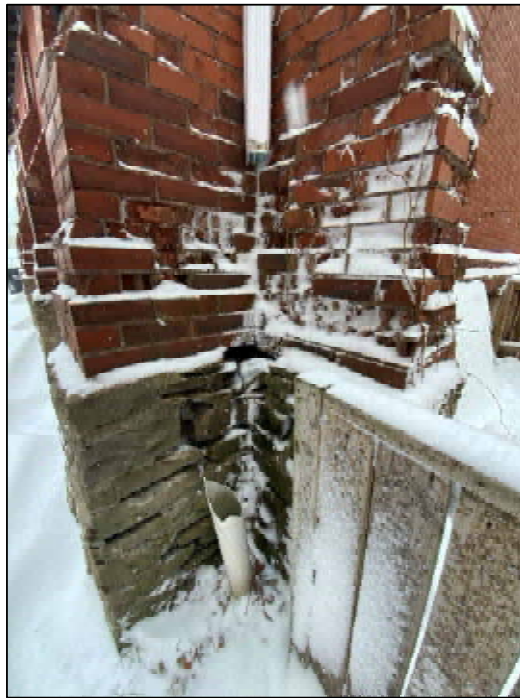
Photograph 12: Open foundation wall at south corner
