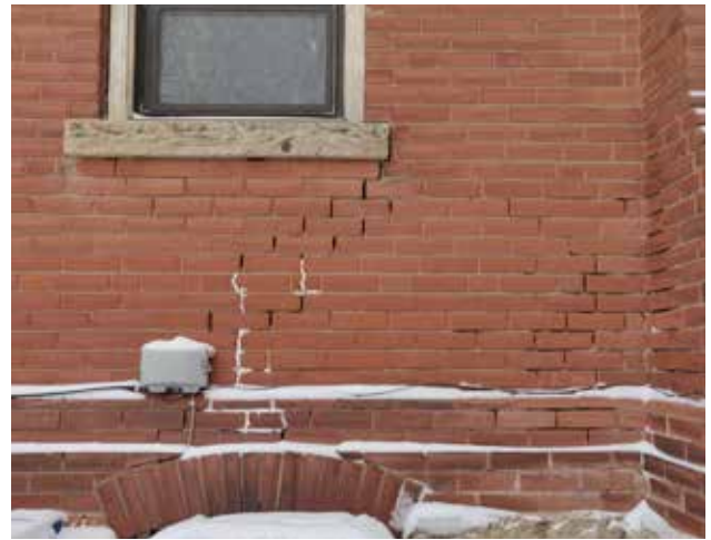
Fig. 5.16. Typical condition at window openings: structural cracks and incompatible repairs.
