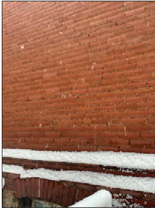
Photograph 8: Open head joints on rear wall
