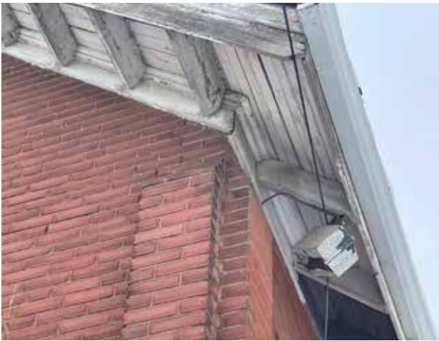
Fig. 5.19. Wood soffits and roof brackets in fair to poor condition.
