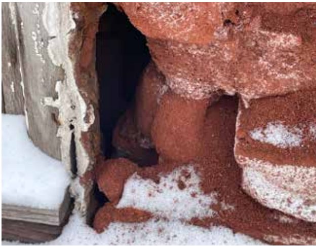
Fig. 5.13. Severe deterioration of masonry at lower portion of front entrance wall.
