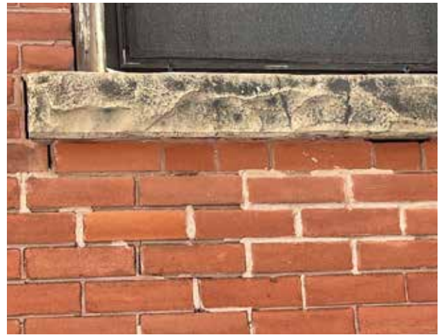
Fig. 5.22. Stone sills are generally in fair condition.
