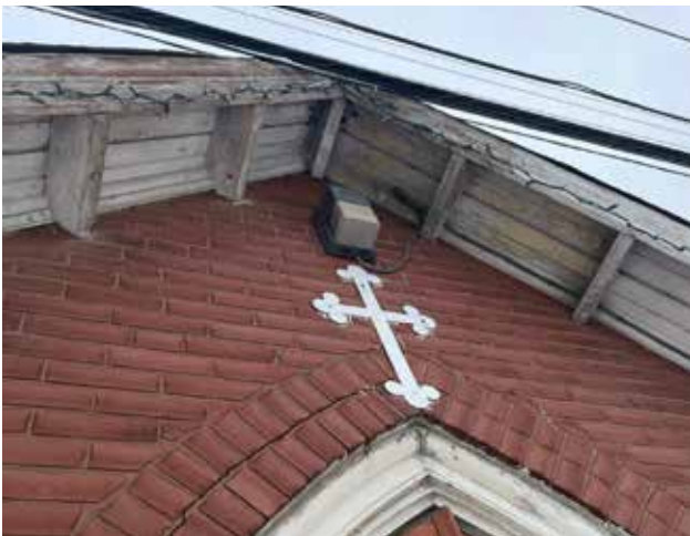
Fig. 5.20. Wood soffits and roof brackets in fair to poor condition.
