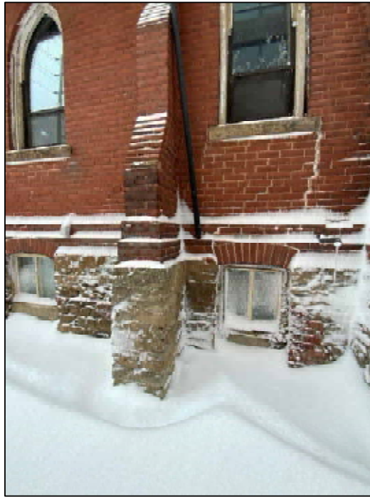
Photograph 7: Typical buttress
