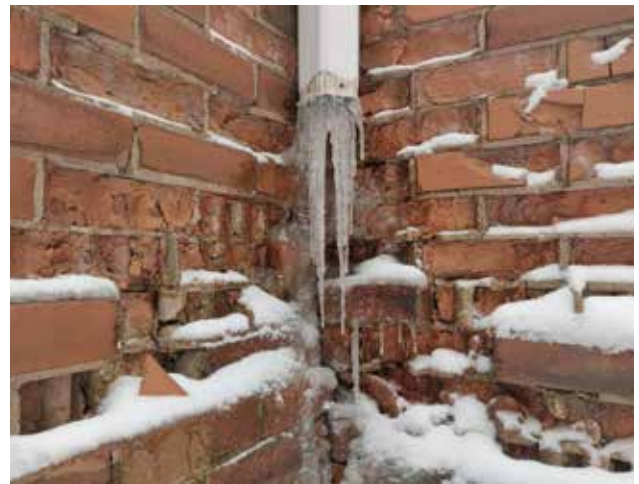
Fig. 5.11. Close-up of inside corner at buttresses: damaged masonry due to water ingress.
