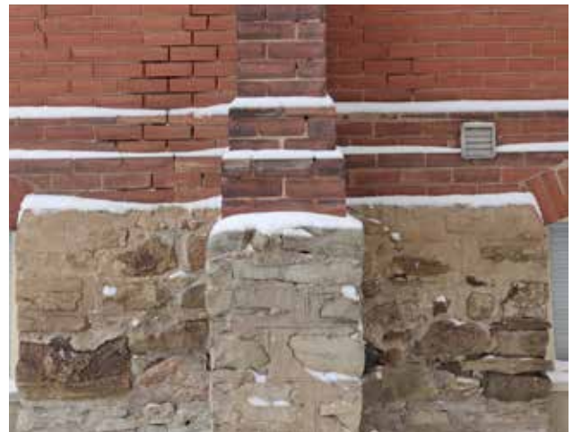
Fig. 5.5. General condition of foundation walls: open joints and incompatible repairs.
