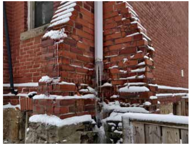
Fig. 5.10. Significant deterioration at buttresses due to water ingress.
