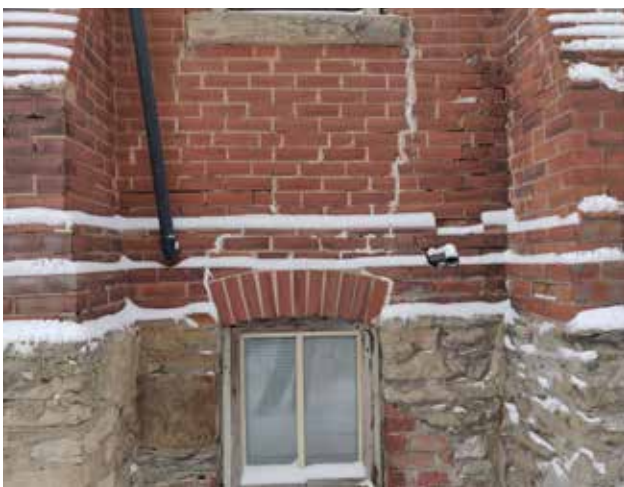
Fig. 5.9. General condition of masonry condition at inside corners. Deteriorated mortar, structural cracks, and incompatible repairs.
