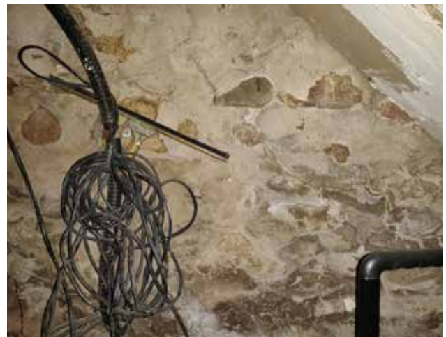
Fig. 5.6. Foundation walls interior face visible in the basement.
