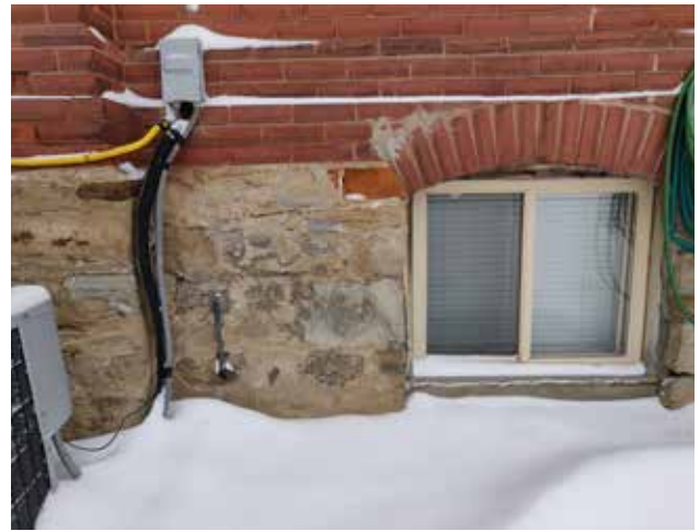
Fig. 5.4. Foundation walls at basement window: incompatible repairs and spalling.
