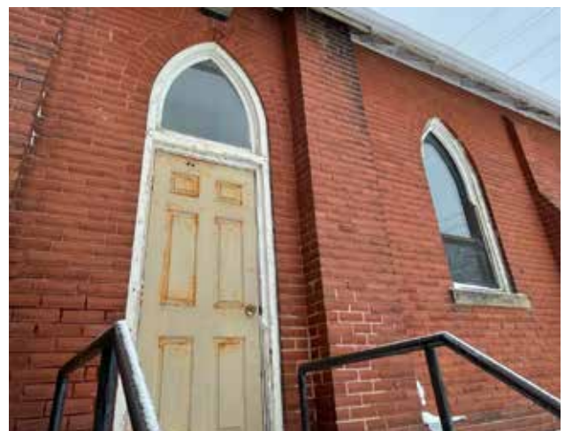
Fig. 5.18. Side entrance door appears to be replaced and in fair condition.
