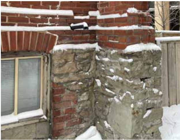
Fig. 5.7. Incompatible repairs of foundation walls and open joints.
