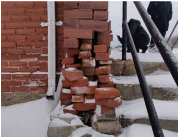
Fig. 5.14. Front buttress partially collapsed.
