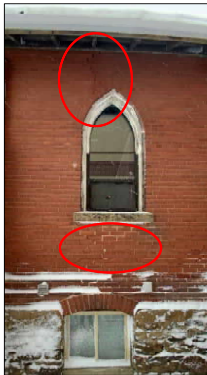
Photograph 9: Cracking above and below sidewall window opening (typical)
