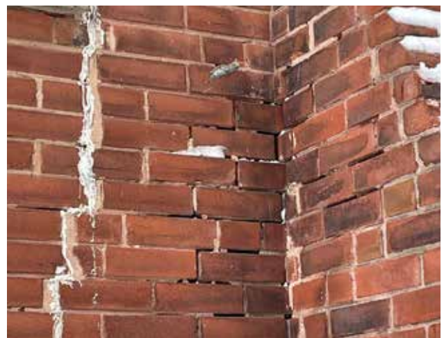
Fig. 5.12. General condition at inside corners: open joints, deteriorated mortar, incompatible repairs.
