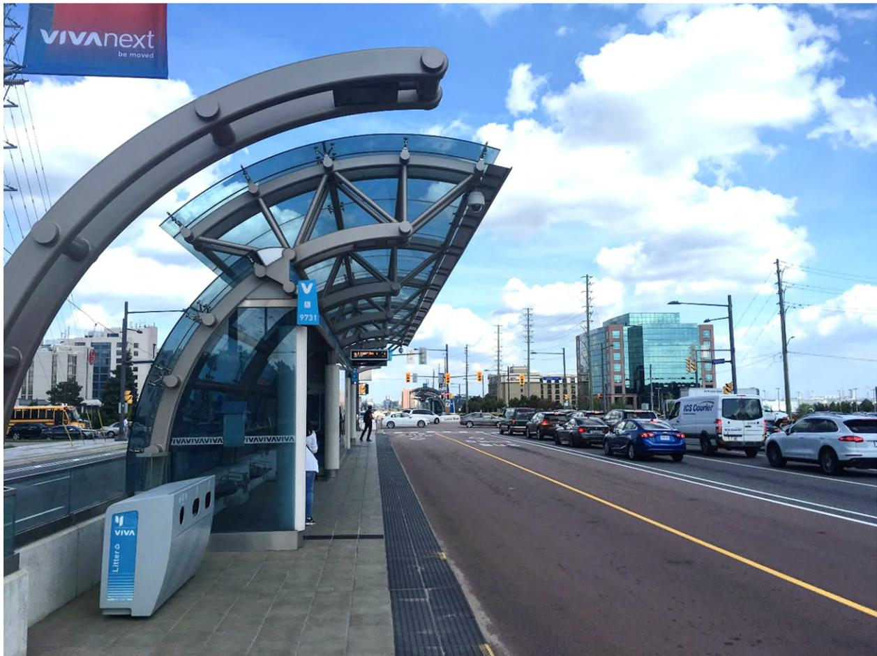
Figure 8: A street with centre-median bus-only lanes to allow transit to operate faster and more reliably (Credit: Matt Pinder)
