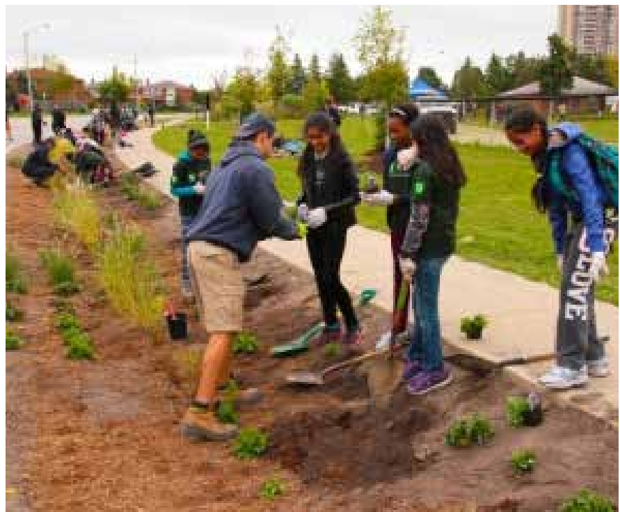
Fig. 100 Retrofitted Roadside Biofiltration Swale, Brampton
