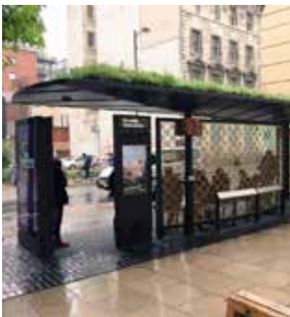
Fig. 89 Bus Shelter Green Roof, Manchester, UK
