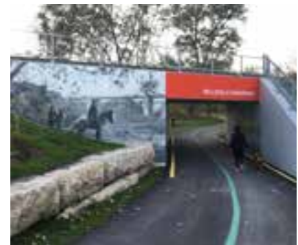
Fig. 138 Pedestrian Rail Underpass, Lower Don, Toronto, ON
