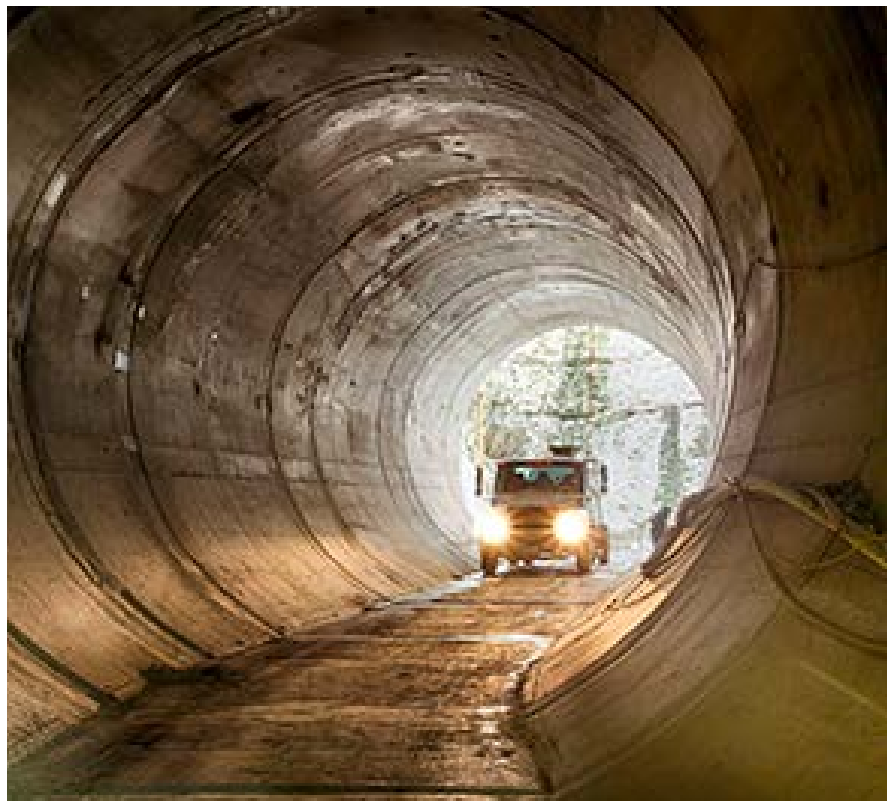
Fig. 40 Waller Creek tunnel during construction. (Photo: City of Austin)
