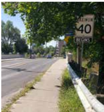
Fig. 22 Sidewalk at Church Street Bridge
