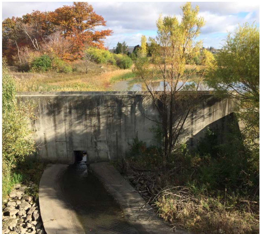
Fig. 6 Edgeley Pond and Park Existing Control Structure
