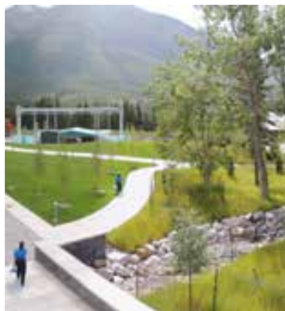
Fig. 101 Integrated Bioswale, Banff Centre for the Arts, Banff, BC
