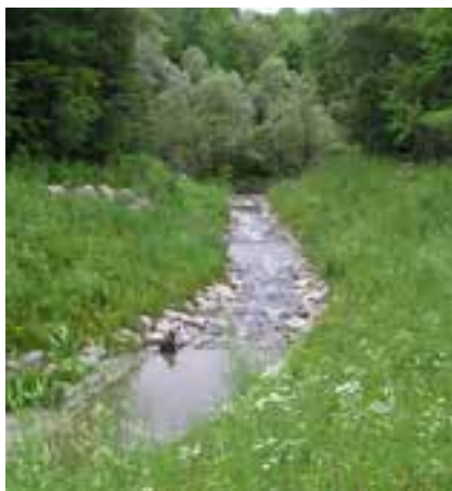
Fig. 95 Riffle structures, Morningside Creek, ON
