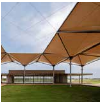
Fig. 103 Rainwater Harvesting Canopy, Rio Olympics, Rua Arquitetos, 2016
