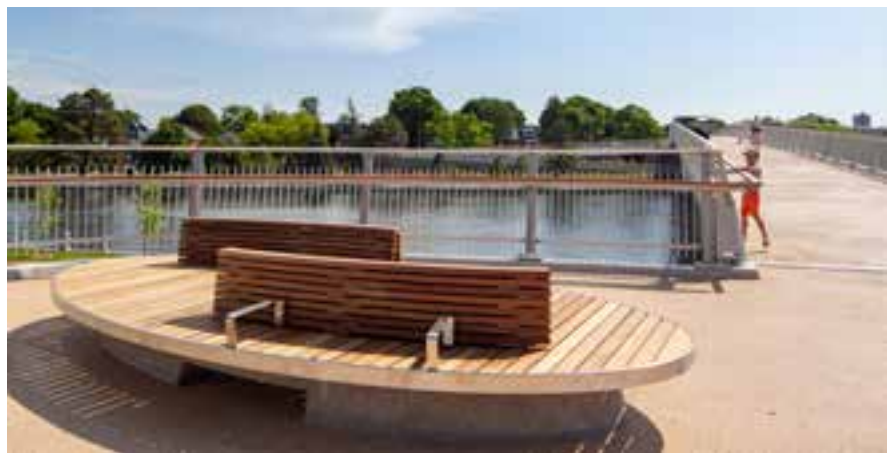
Fig. 193 Bridge Lookout, Flora Footbridge, Ottawa, ON
