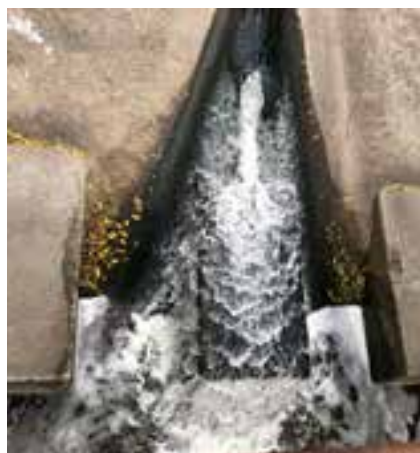
Fig. 31 Bypass Channel Weir at CN Rail Bridge
