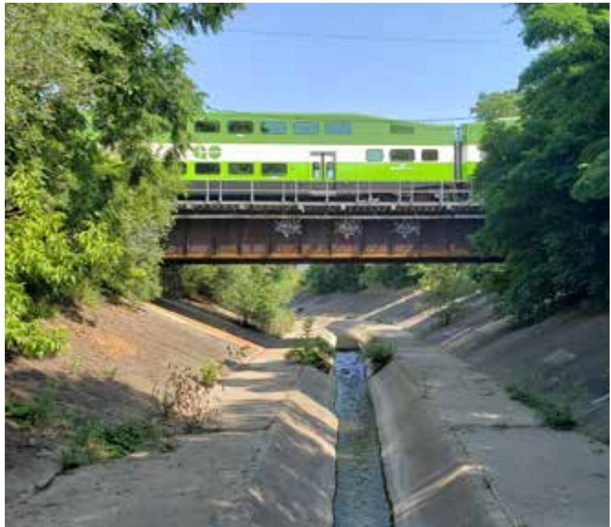
Fig. 20 CN / GO rail bridge over the Etobicoke Creek
