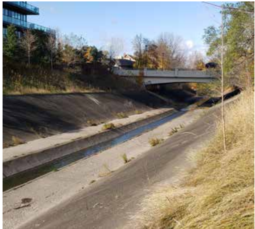
Fig. 45 Etobicoke Creek bypass channel looking toward the Queen Street Bridge
