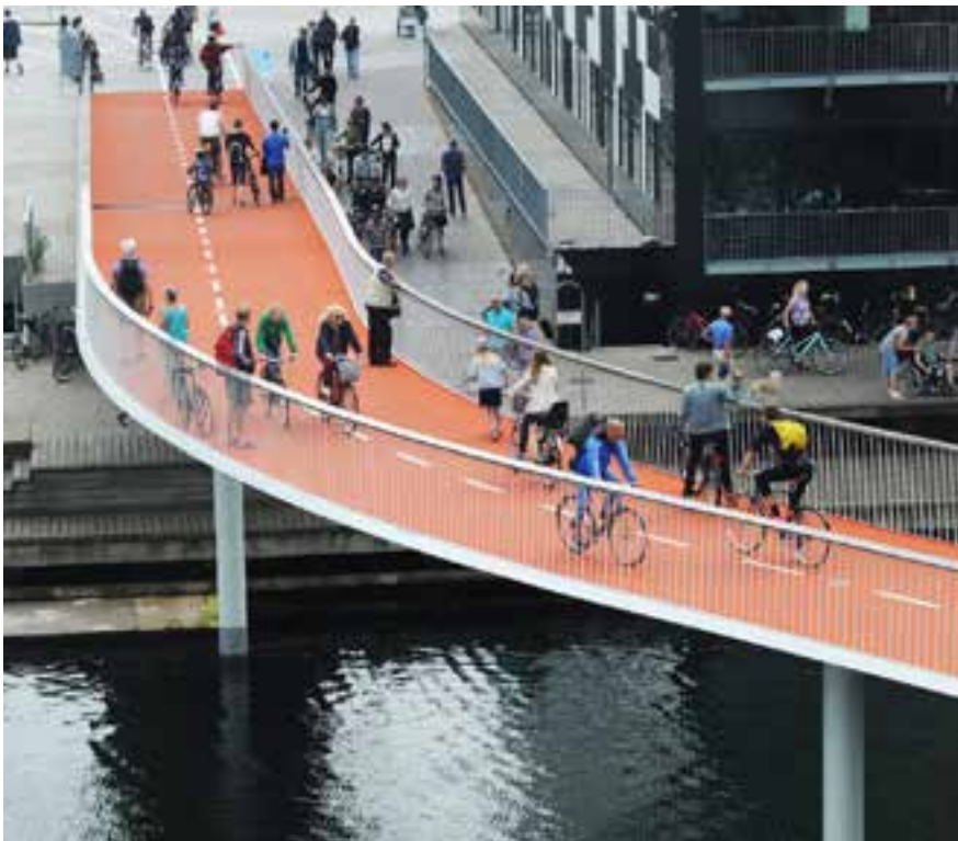
Fig. 91 Bicycle Snake Bridge , Copenhagen
