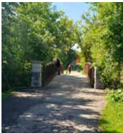
Fig. 48 Pedestrian Bridge In Duggan Park
