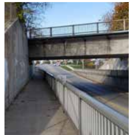
Fig. 18 Centre Street Rail Underpass
