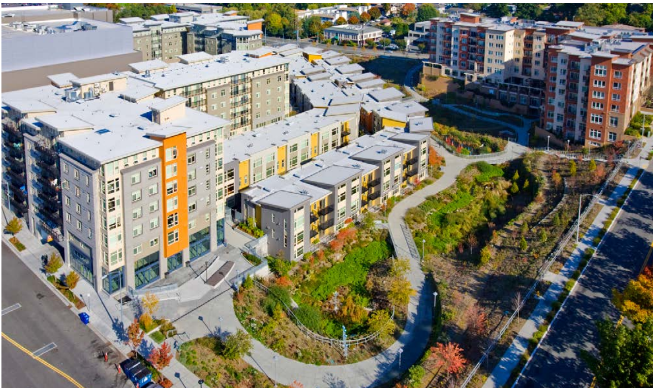
Fig. 17 Thornton Creek Water Quality Channel. Photo: SvR Design.
