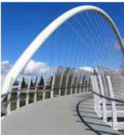
Fig. 185 Griffiths Pedestrian Bridge, Burnaby, BC
