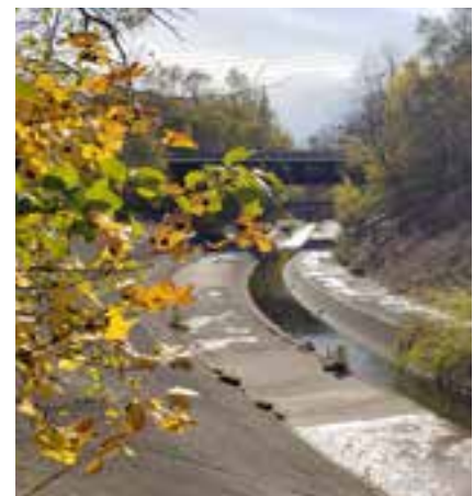
Fig. 4 Bypass Channel north of the CN Rail Bridge
