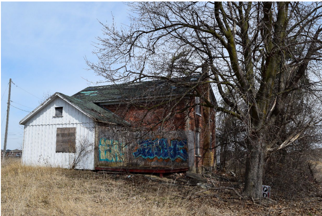
Image 6: West face of Clark/McClure House, note plywood hording is concealing a structural opening that will need to be included on architectural plans
