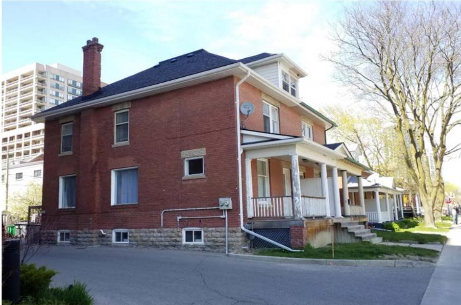
West facade of 22 John Street, taken from the southwest. Stone lintels and sills are visible on the windows. A cut stone finish is present at the base of the building, behind it the foundations are rubble stone.
