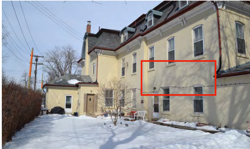
The east portion displays a significant bulging of the exterior brick wall at the second floor level, above the original extent of the one-storey "running bond" (clip-bond) brick construction, above which a second floor with exterior common bond brick walls was constructed.
