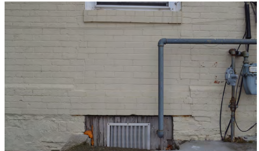
Alterations made to the ground floor windows at main elevation, where previous doorway rough openings were infilled with new brick, at removed veranda, showing a disruption in the original brick chamfer at building's base. New brick sills are additionally typical at these alterations.
