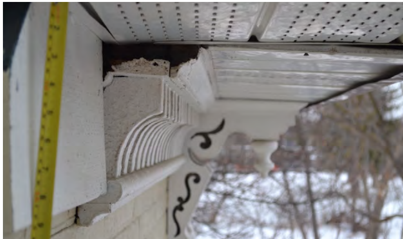
Detail view of the wood cornice at eave of mansard roof, showing missing section of dentils along the main elevation, and new (typical) non-compatible soffit material.
