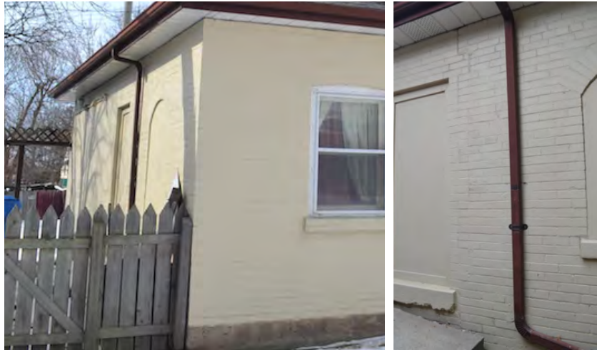
(left) Showing one-storey brick c.1925 extension east elevation, with detail at (right) showing the continuous joint line between infilled doorway and window which differentiates the brick bond construction types: running bond on left, toward the south elevation; and inconsistent common bond at right, toward the main elevation.
