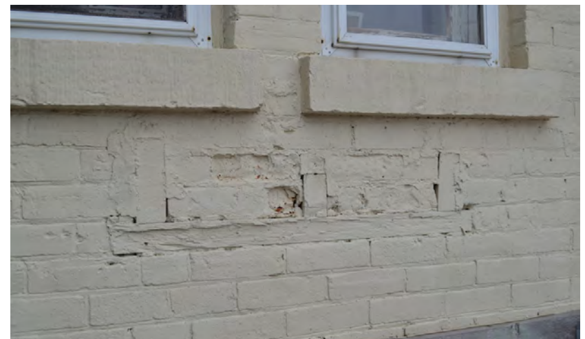
Remnants of wood bracketed structure with iron cresting at paired window of third floor (attic), main elevation. The condition also exists along the Elizabeth Street North elevation.
