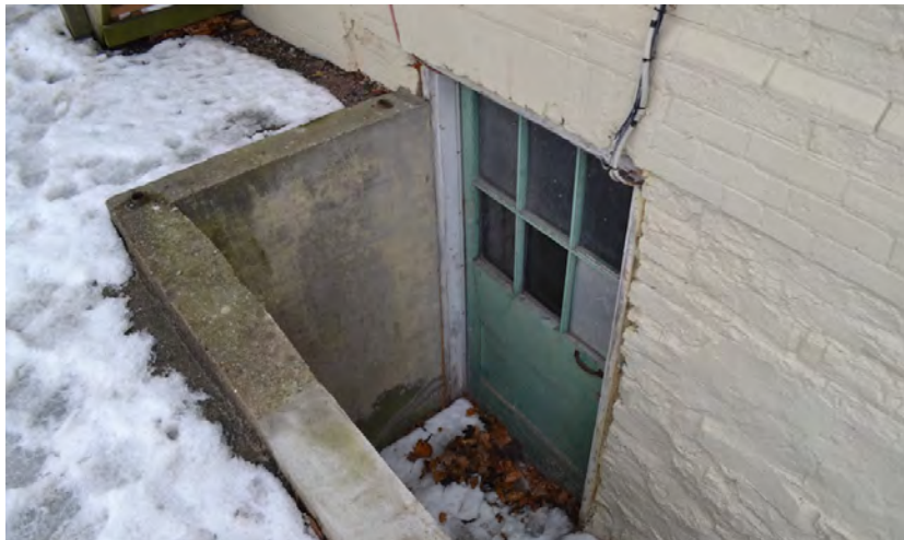
Basement entrance at main elevation, showing extent of brick infill at rubble stone foundations.
