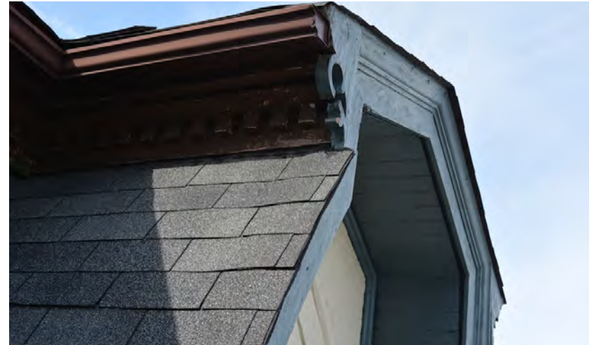
Detail view of typical convex mansard dormer trim detail with bracket; note the original wood soffit is intact (view of main elevation)
