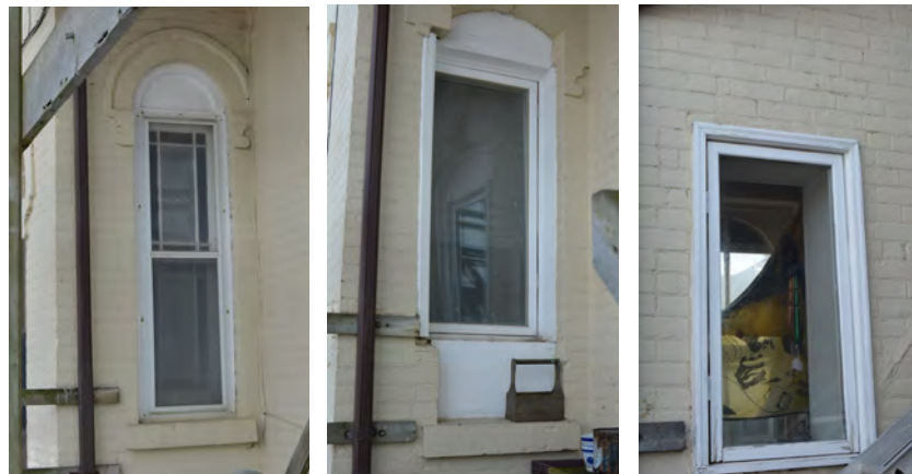
View of the south elevation windows and non-original door at east portion. This area has seen alterations in its fenestration, as shown by brickwork investigations (there was likely a door previously situated at area highlighted red).
