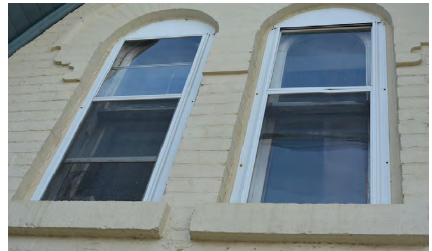
Detail view of typical stone sill, with minor chips; showing condition at main (north) elevation, third floor paired windows.
