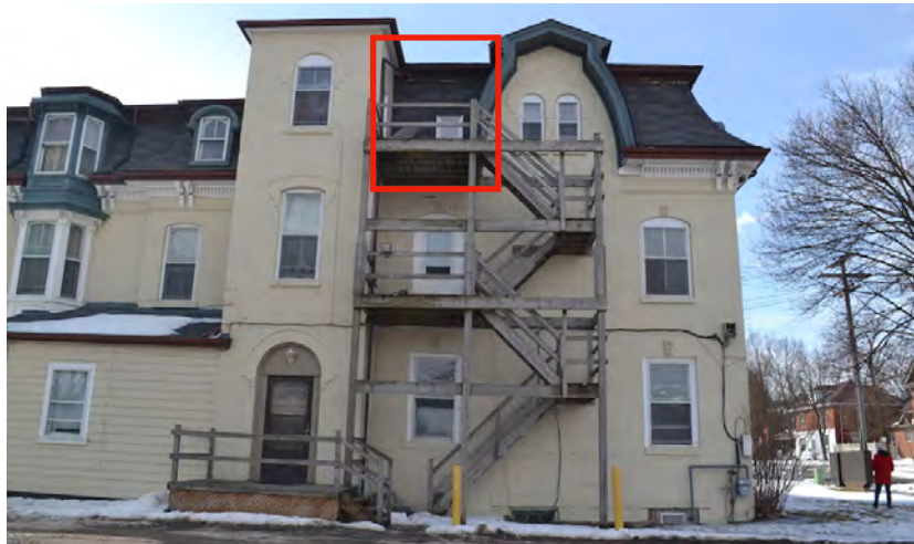
View of main elevation, showing area where mansard roof removed, highlighted red, today replaced with elevation of asphalt finish.
