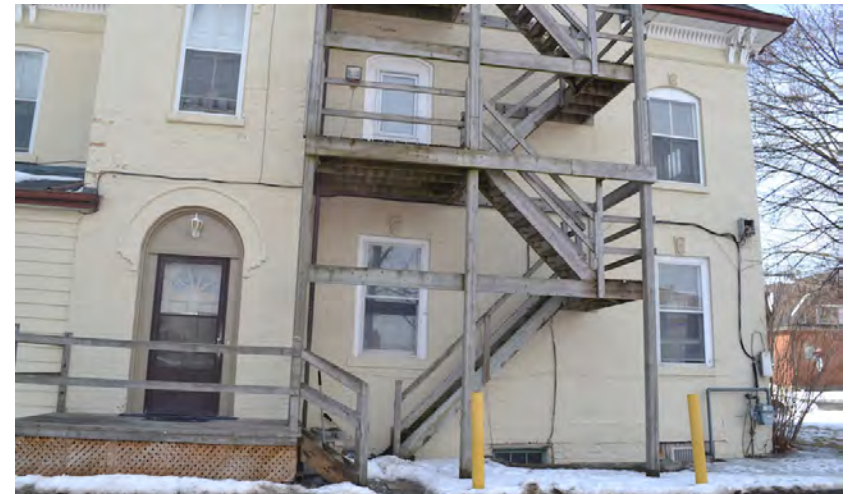
View of the main elevation, showing the non-original door at the base of tower; the two non-original windows at ground floor of west portion (replacing original doors); the original 2/2 sash windows at tower and west portion; and altered window at fire escape that retains its wood trim moulding at brick.
