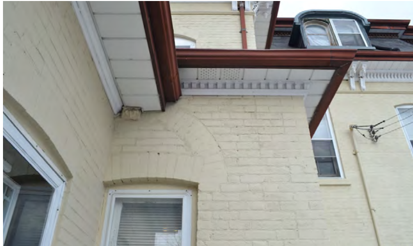
Obstructed brick voussoir and flower-themed keystone combination at ground floor window, where c.1911 extension abuts the original one-storey south extension the (rear) Elizabeth Street North elevation.
