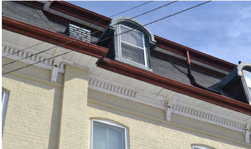
View of south elevation at east portion, showing continuous concave mansard roof profile and typical hooded dormer window; typical missing wood dentils and bracket at cornice
