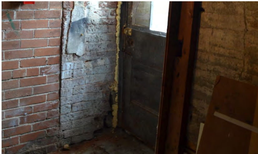
Basement entrance at main elevation, view from interior, showing extent of brick infill at rubble stone foundations, with new adjacent brick interior partition wall.
