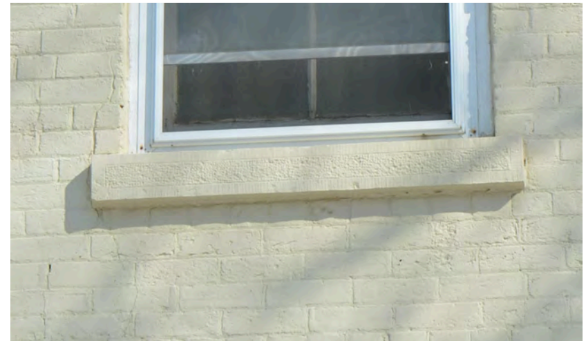
Detail view of punched sill, typical of second floor at east portion, as well as two units found at ground floor of c.1911 extension (west and south elevations).
