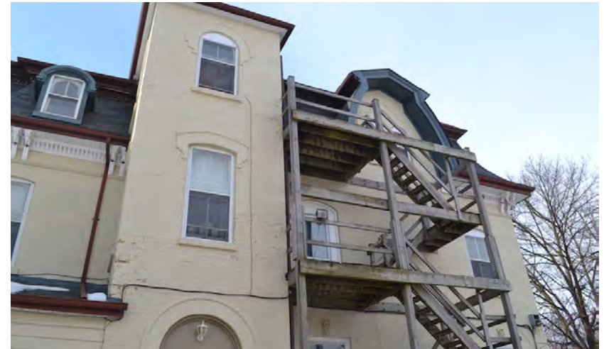
Chipped and cracked bricks at voussoir dripstone moulding of second floor window; Localized areas of deteriorated brick at tower elevations to be further investigated; non-sympathetic wood fire-escape to be removed, and adjacent masonry investigated.
