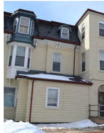
(left) View of north extension, existing condition showing non-sympathetic wood cladding and new window unit. (right) Archival documentation showing original design of north extension, c.1900, as extension of original veranda.
