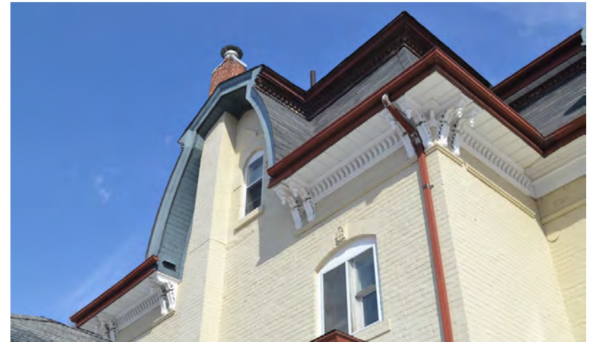
Chimney obstructing previously paired window with combined brick voussoirs at third floor (attic) of west portion, along the Elizabeth Street North elevation; Showing altered window rough opening and non-sympathetic contemporary window at second floor, above original south extension.
