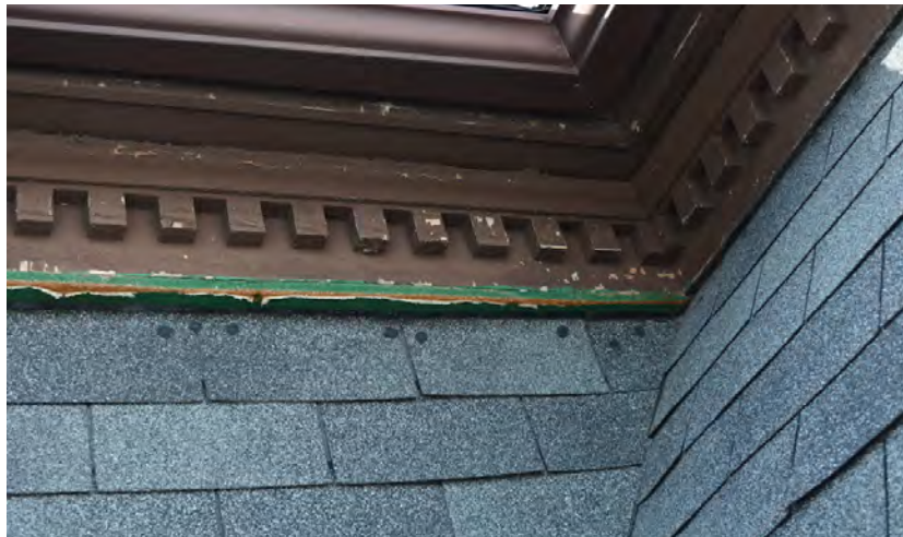
Detail view of main elevation, where convex mansard dormer meets the new asphalt elevation; showing typical wood cornice with dentils.
