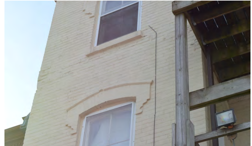
Detail view of brick deterioration at main (north) elevation tower, typical localized condition at the tower, and chipped brick dripstone at second floor voussoir; showing area between second and third floors.
