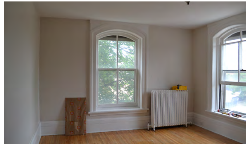
Interior wood casing trims and sills largely remain throughout, and appear in good condition. View of interior showing North and West elevation, second floor windows of the west portion.
