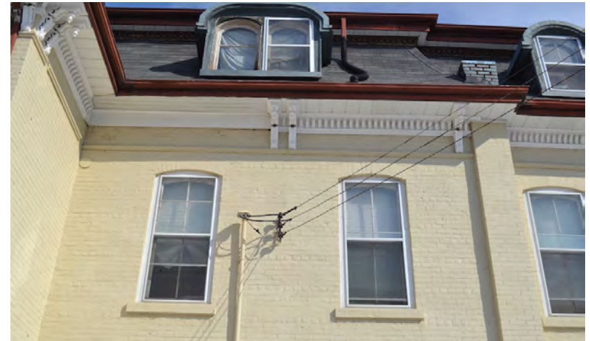
View of south elevation, showing the a-typical dormer type which consists of paired windows; typical missing section of dentils at wood cornice.
