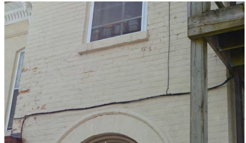
Detail view of brick deterioration at main (north) elevation tower, typical localized condition at the tower, showing area between ground and second floors.
