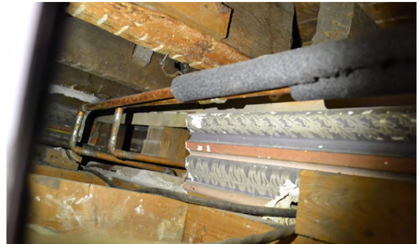
Partial remnants of the presumed original painted plaster crown mouldings remain tucked away within the new drop-ceiling of west portion adjacent staircase.
