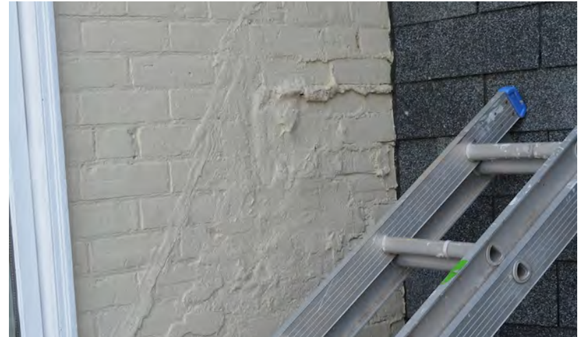
Remnants of removed mansard roof section visible at adjacent tower brick elevation (main elevation).
