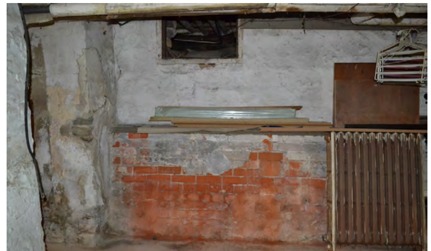
East portion main elevation foundation wall, view from interior, showing opening within original rubble stone foundation at left, and the continuous brick buttress.
