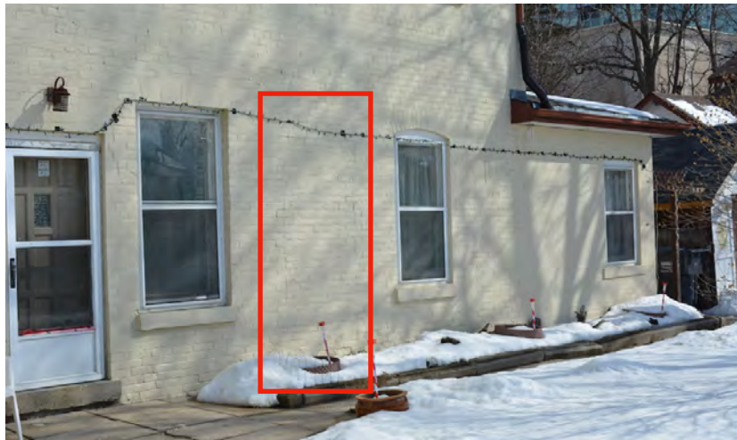
View of the south elevation windows and non-original door at east portion. This area has seen alterations in its fenestration, as shown by brickwork investigations (there was likely a door previously situated at area highlighted red).
