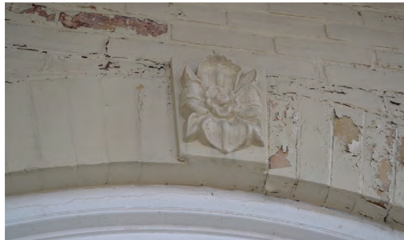
Paint flaking throughout; showing second floor window at main elevation, west portion, and characteristic flower-themed keystone set within segmental arch.
