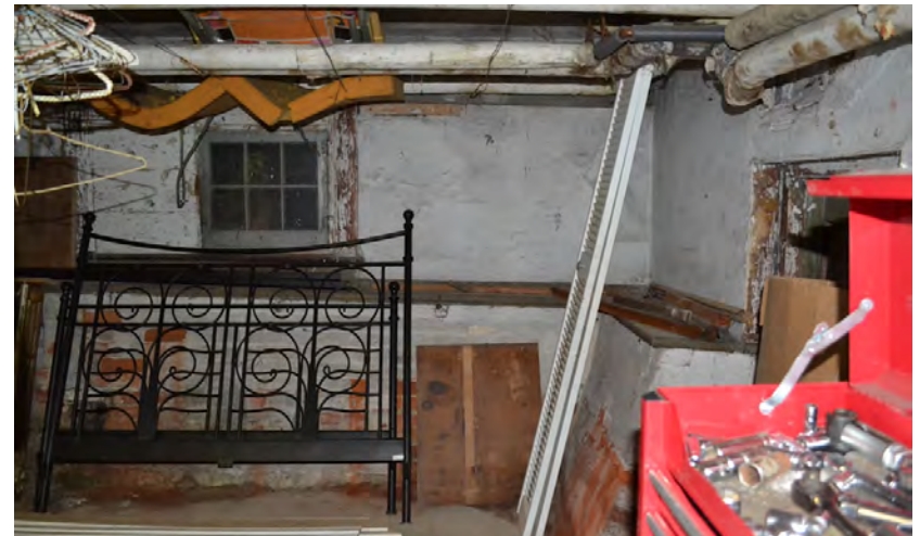
Original six-pane window at basement level of east portion, no longer with access to its adjacent exterior space (at main elevation).
