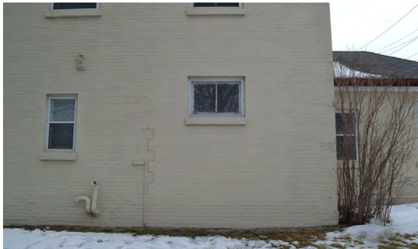
Non-sympathetic contemporary window at West elevation, at the location of an original one-storey bay window (since removed) showing recent non-sympathetic repointing repairs at joint line between original and non-original brick of infill at removed one-storey bay window.
