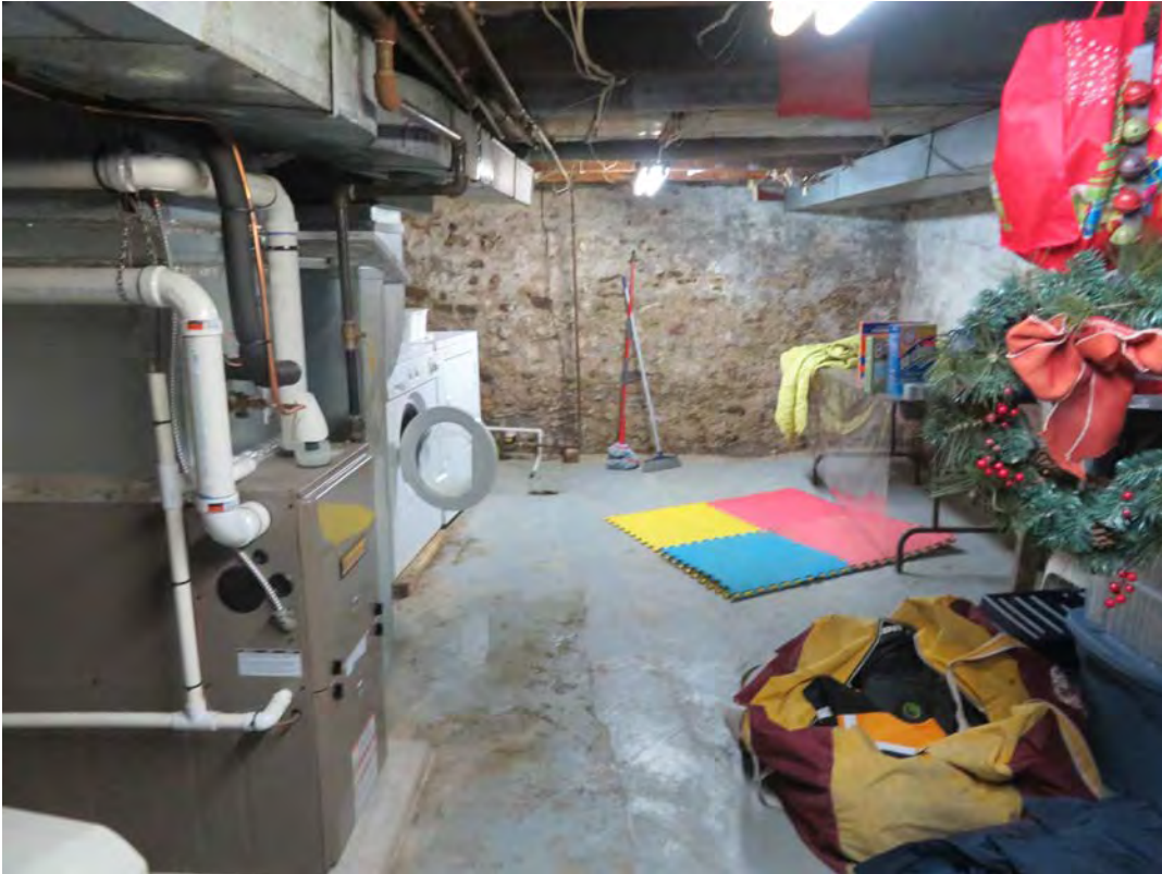
BASEMENT FURNACE ROOM – rubble stone foundation & full basement in this area
