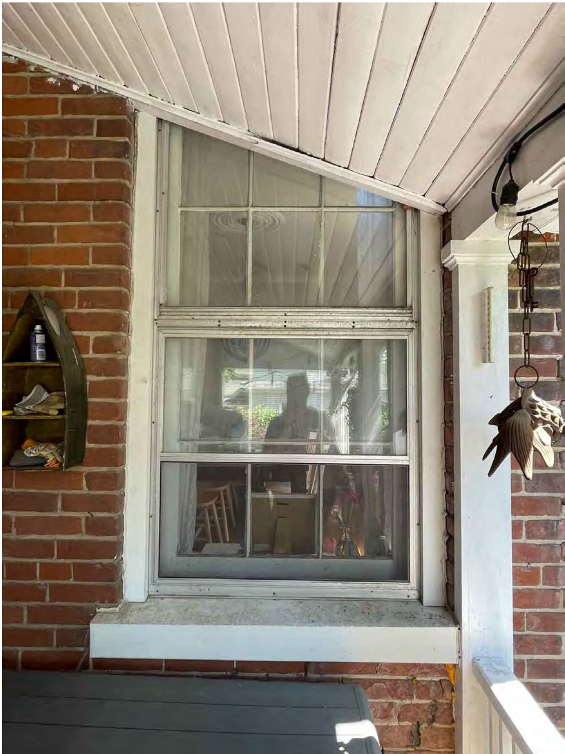
SIDE PORCH – the roof overlaps a window indicating that the porch was probably an early addition built in the late 19 th or 20 th century
