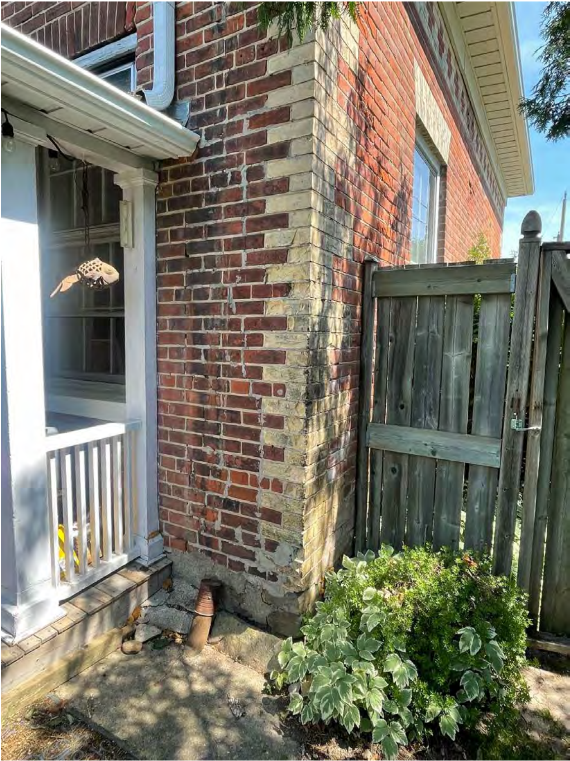
BACK CORNER – some open mortar joints and spalling of the buff brick
