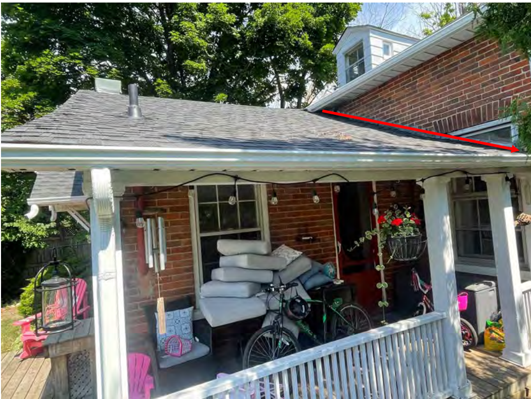
SIDE PORCH – the gable roof of the tail section extends over the porch and overlaps one of the windows
