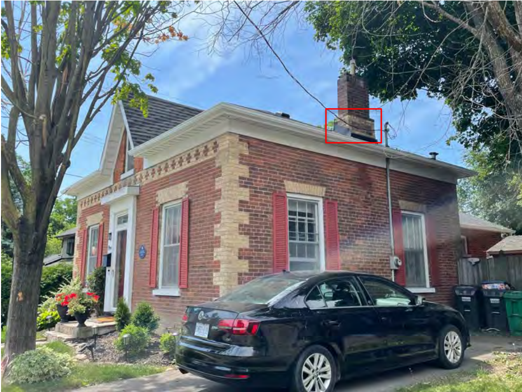
DRIVEWAY ELEVATION – 1.5-storey, 3 by 2 bay dwelling with a one storey tail at the back – the roofline of the addition is lower and the footprint is narrower – there is a chimney on this elevation
