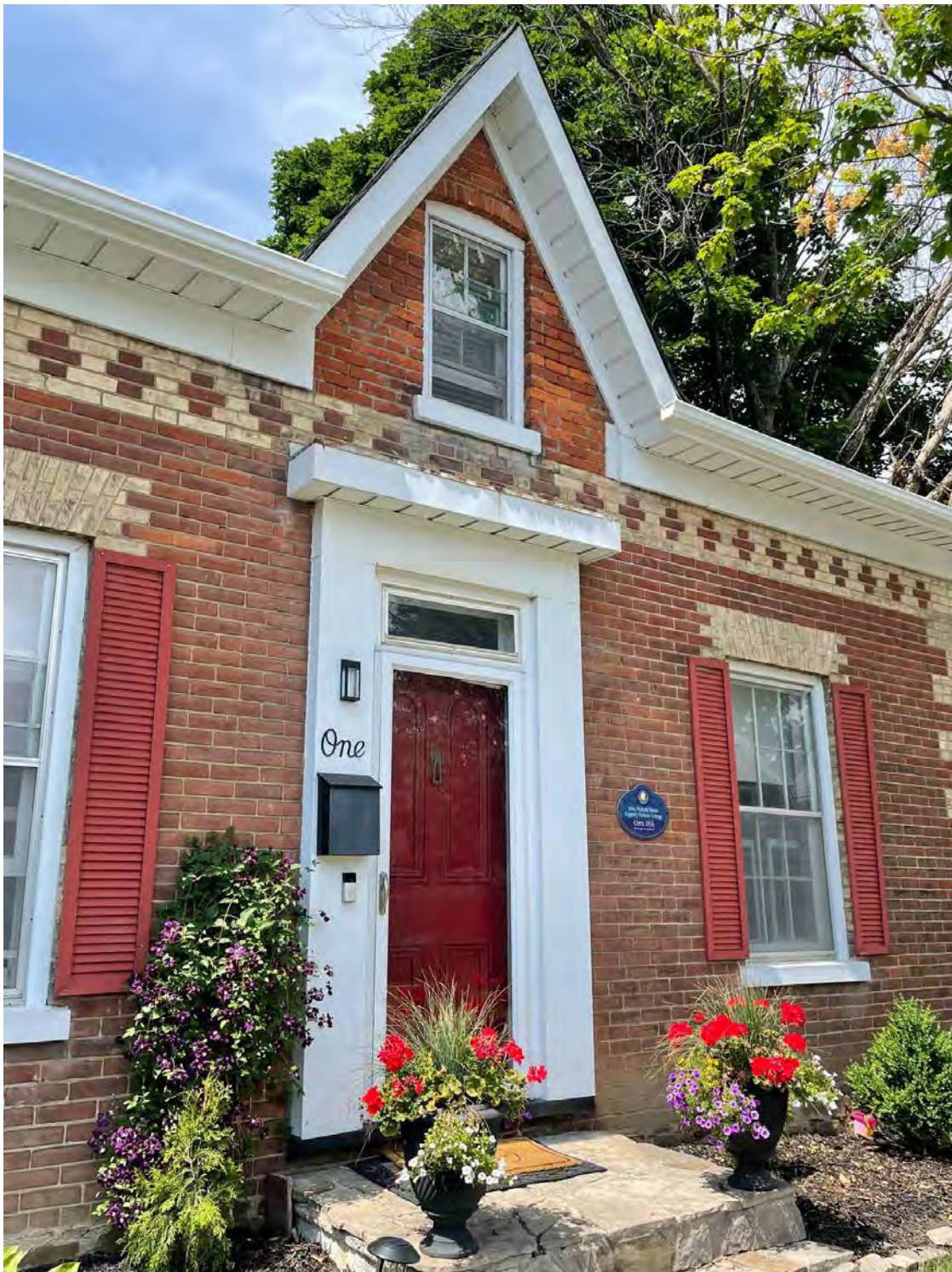
FRONT GABLE – the front gable appears to be a later alteration, possibly done in the late 19 th or early 20 th century – the door frame has been clad with aluminum, perhaps on top of original wood components – the soffits and fascia are aluminum, perhaps with original wood components beneath
