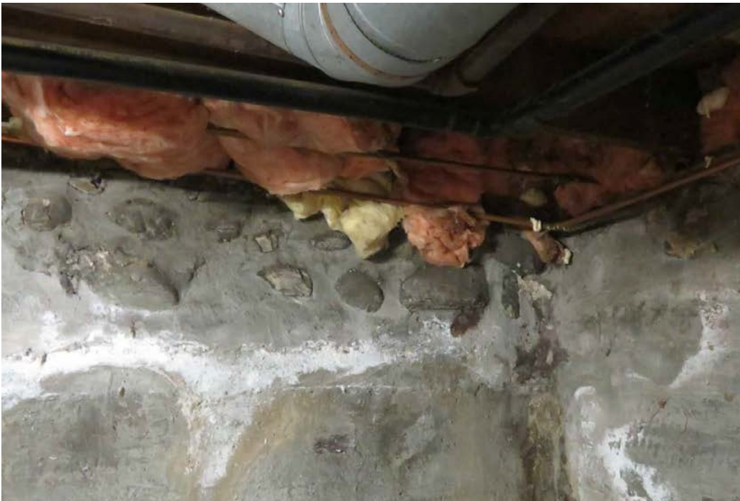
BASEMENT – rubble and concrete below the rear section – originally a crawl space that was later excavated and underpinned
