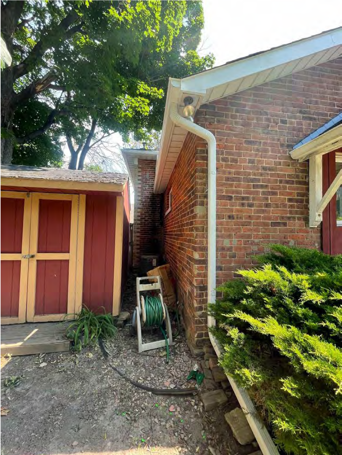
BACK CORNER ON THE DRIVEWAY SIDE – the addition is constructed of red brick without the buff brick detailing of the front – the shed is a modern frame structure
