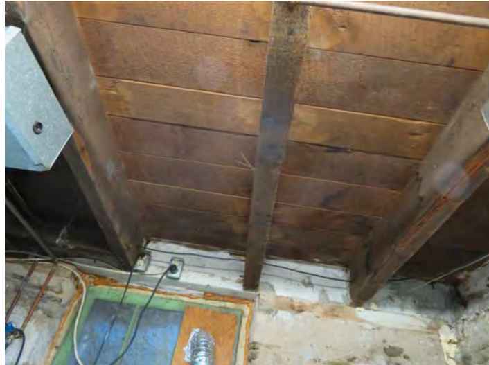
FLOOR FRAMING - circular sawn lumber & wide spacing of the joists are consistent with a mid-19 th century date of construction
