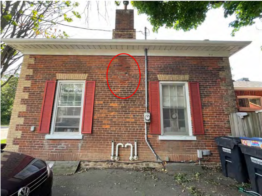
DRIVEWAY SIDE ELEVATION – note the wide overhang of the roof – note the spalling of the brick below the chimney – there is a basement below and two windows above grade on this elevation - note the rubble stone foundation
