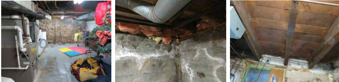
c. 1850s RUBBLE STONE FOUNDATION (left) c. 1920s or 1930s CONCRETE UNERPINNING (center) c.1850s floor framing (right)
