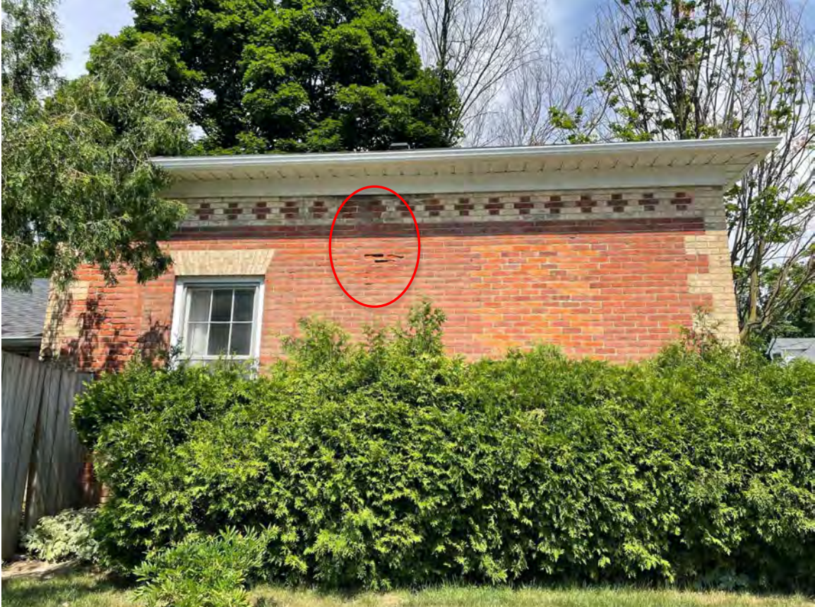
DAVID STREET ELEVATION – note spalled area of brick indicating that there may have been a chimney above, similar to the other side elevation – note the bricked in window
