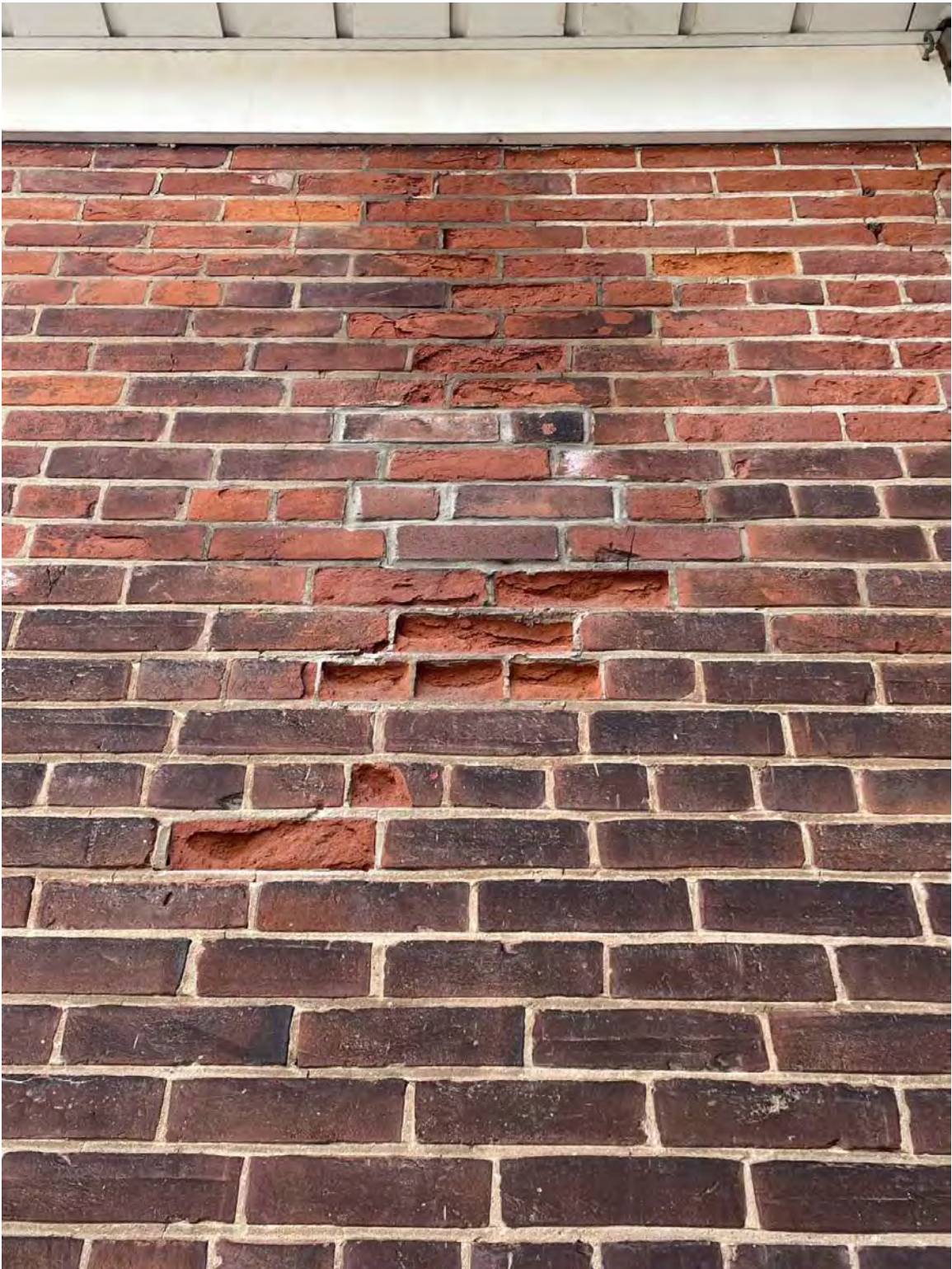
DRIVEWAY SIDE ELEVATION – detail of spalled brick noted above
