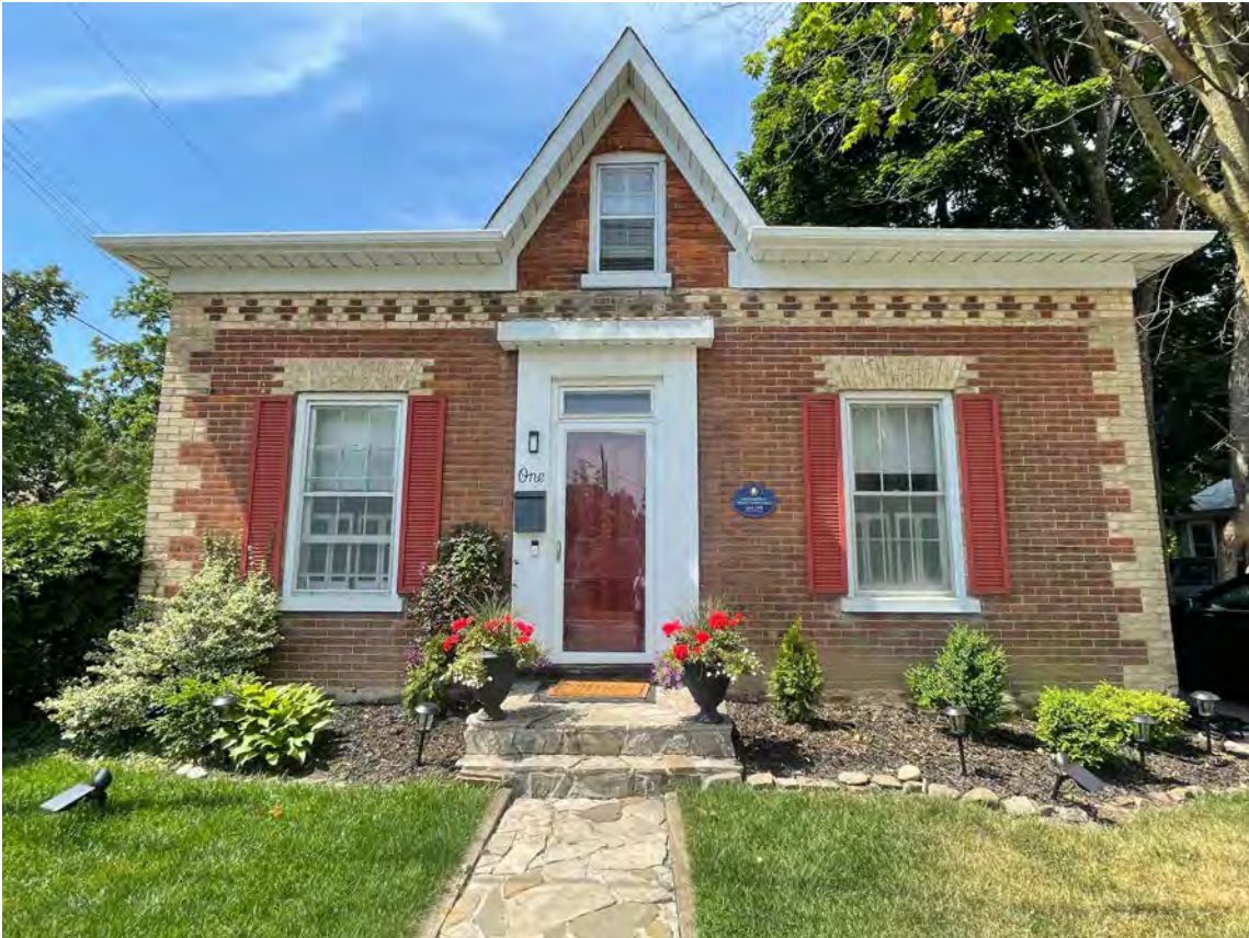
ISABELLA STREET ELEVATION – 3 bay, 1.5-storey 'Ontario Cottage' with a hip roof that was modified at the front for a gable – note the dichromatic brickwork that employs buff brick for corner quoins, frieze and window lintels. The windows are 6 over 6 wood sash.
