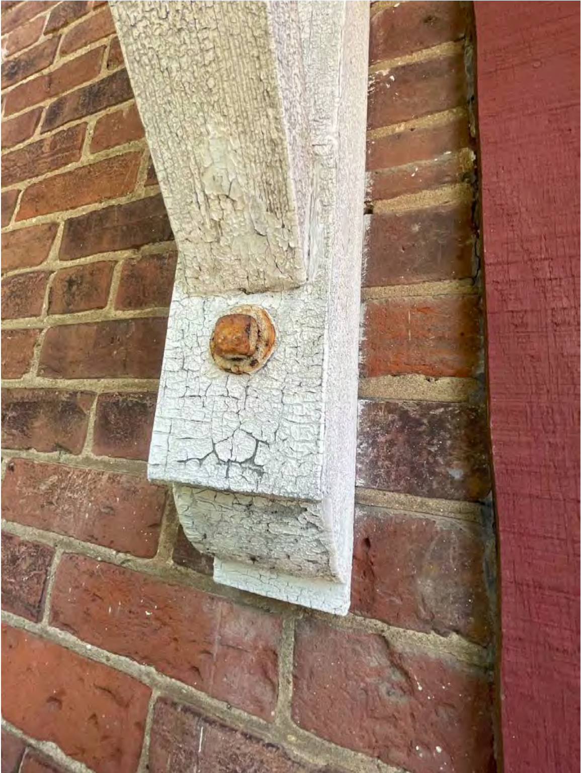
BACK DOOR – detail of the metal bolt that anchors the wood bracket into the masonry
