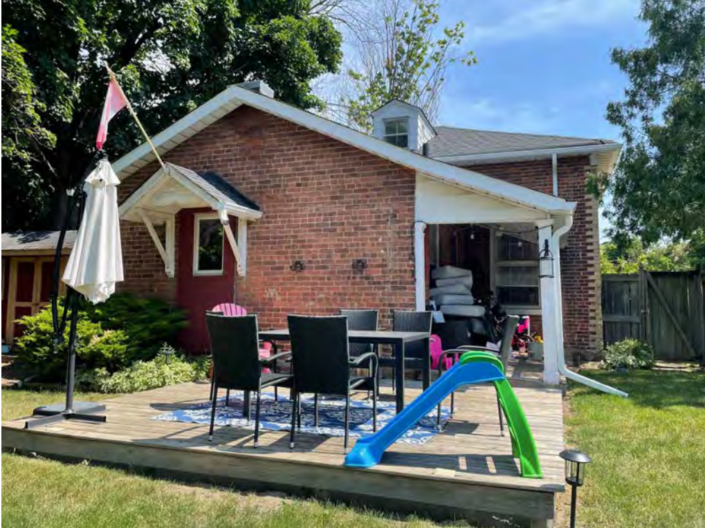
REAR ELEVATION – the rear tail section has a gable roof that extends over a porch on the David Street side – the roof of the porch overlaps a window on the rear elevation of the main portion of the house
