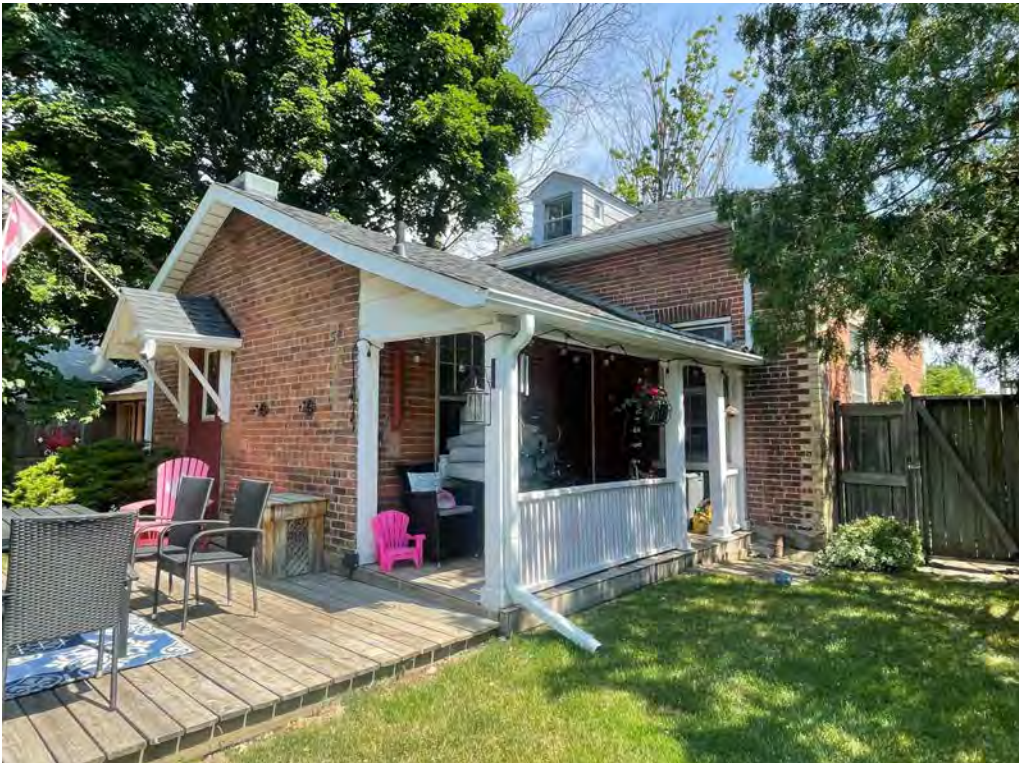
REAR ELEVATION – the 1917 Fire Insurance Plan shows a porch in this location but the wood posts and railings are probably more recent – there is a small dormer above that also seems to be a fairly recent alteration
