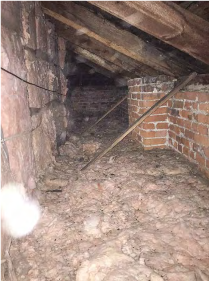
ATTIC – unfinished area under the eaves on the David Street side – the base of a chimney is visible, confirming that there was originally a matching chimney on this side
