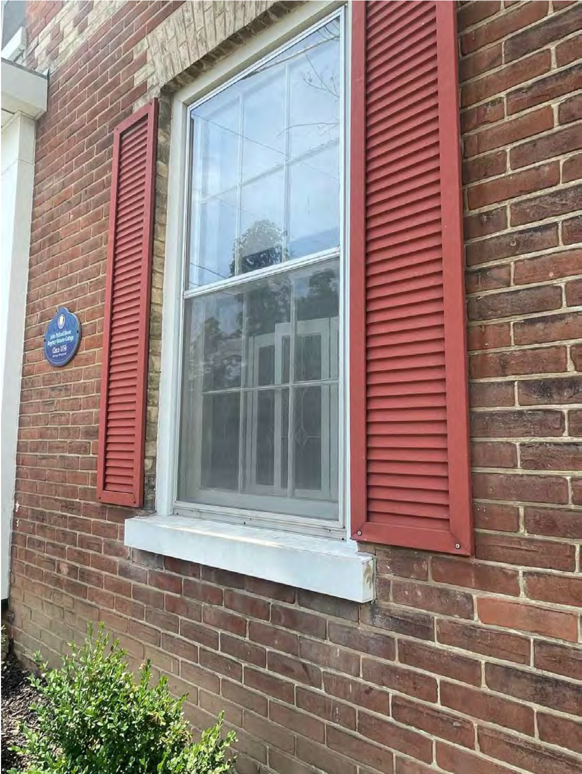
WINDOWS – wood sash windows with slender muntin bars are probably original – the sills have been covered with aluminum and may be wood beneath – the aluminum shutters are recent
