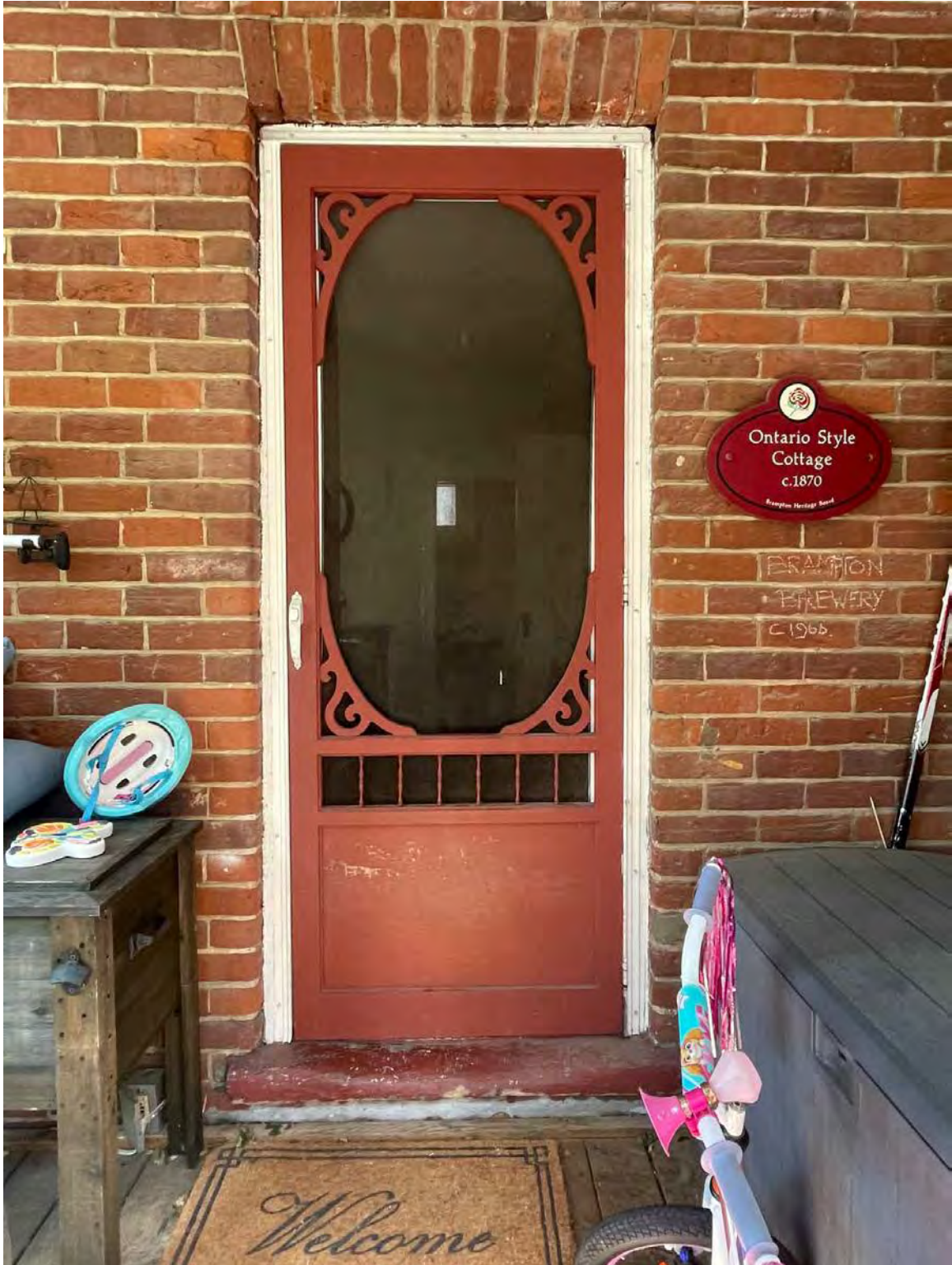
SIDE DOOR – the opening has a flat brick arch
