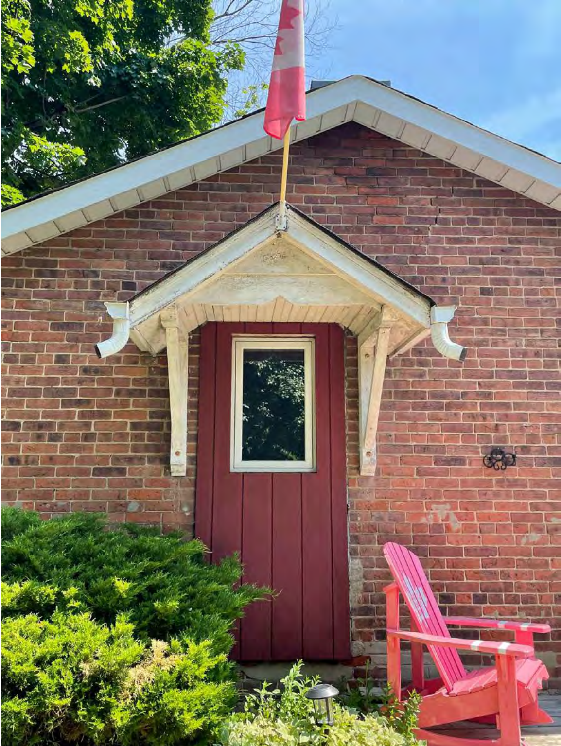
REAR ELEVATION – a back door has been recently blocked up with wood framing and cladding and converted to a window – it has a wooden roof above that is bolted into the masonry – given the Arts & Crafts influenced style of this feature and its simple construction, it probably dates from the 1920s or 30s.
