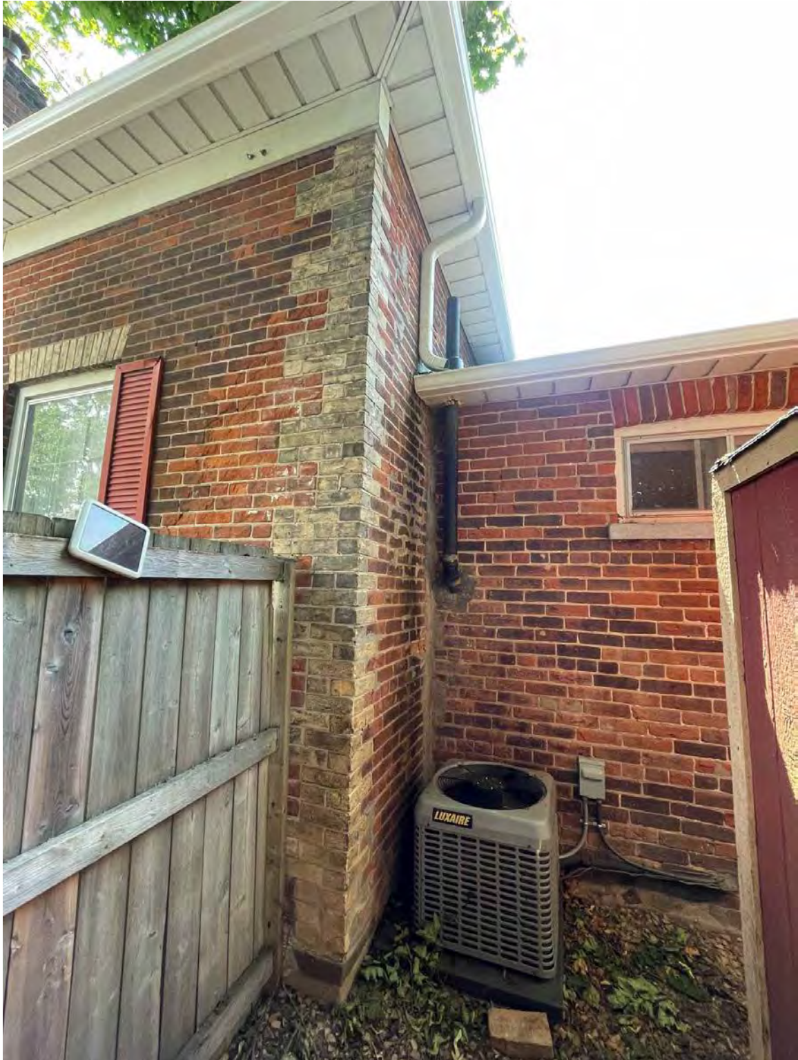
TRANSITION TO THE REAR SECTION – note the buff brick quoin detail – the addition is double-brick construction, note the different bond pattern of the addition that has a row of headers every 8 th row – note the rubble stone foundation – the tail may be original or was an early addition built in the late 19 th or early 20 th century – the masonry openings have segmental brick arches
