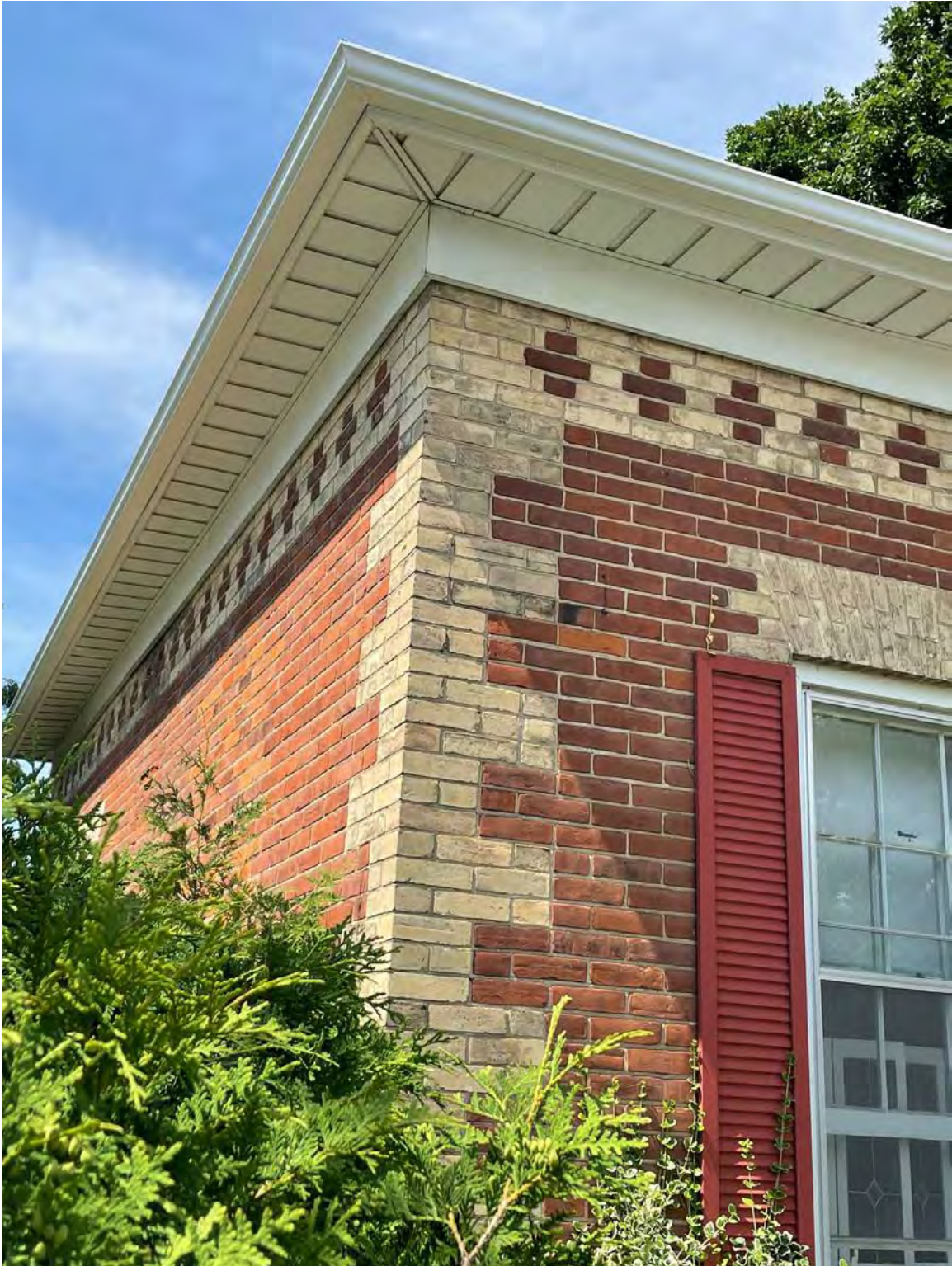
DI-CHROMATIC BRICK – red brick with buff brick quoins, window arches, and frieze – triple brick construction; a double layer of brick with headers and a third layer in running bond on top – the window arches are flat
