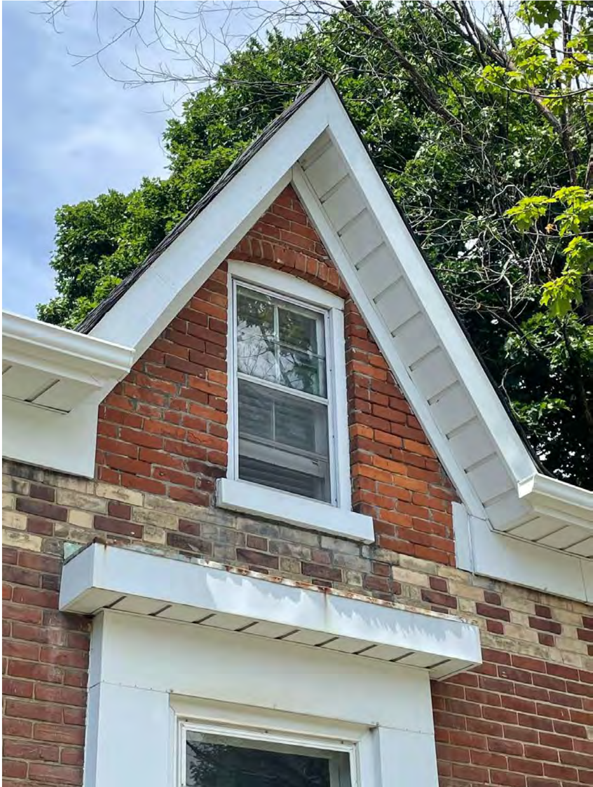
FRONT GABLE – the front gable is an early addition to give additional space on the 2 nd floor – probably done in the late 19 th or early 20 th century – the window in the gable has a shallow segmental arch in red brick
