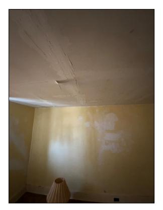
Photograph 2: Previously repaired ceiling damage
