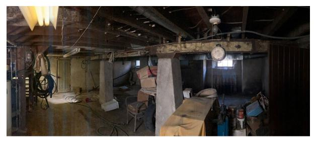
Plate 22: Basement main area showing the machine cut summer beam and concrete pilasters
