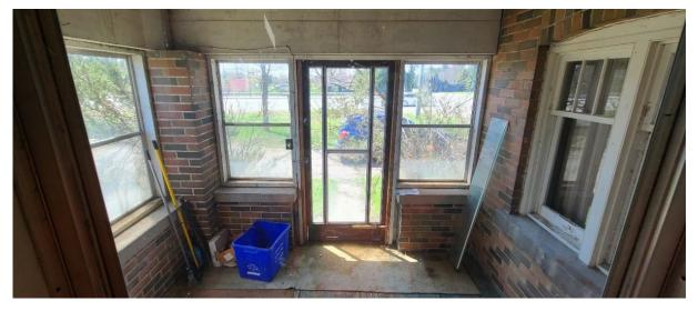
Plate 7: View of enclosed porch with mix of one-over-one windows and three over one segmentally arched windows with double course brick youssoirs
