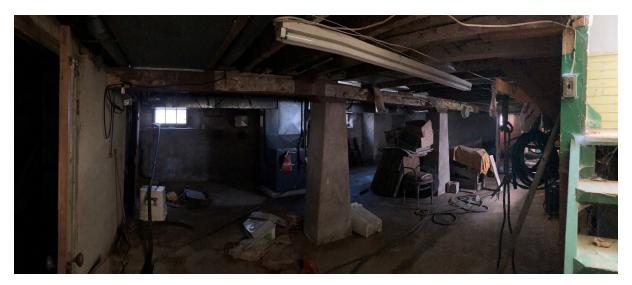
Plate 21: Basement main area including summer beams and concrete pilasters
