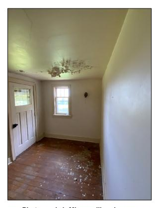
Photograph 1: Minor ceiling damage
