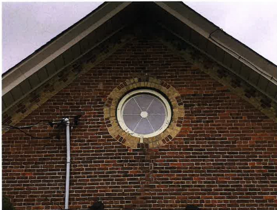
Image 2: Detail of the bullseye window and dichromatic brick pattern under the gable eaves.
