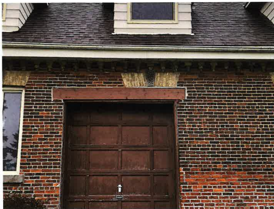
Image 7: View of the garage door on the north elevation of the schoolhouse, note the remnant buff brick lintel with keystone from the former window opening.
