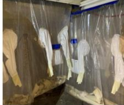
Photo 2: Representative picture of work area during Type 2 (Glove bag) abatement of Aircell pipe insulation – Basement.
