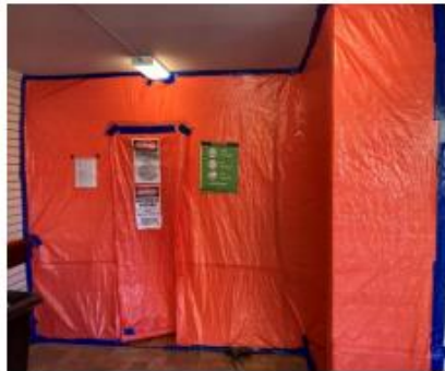
Photo 1: Clear Asbestos warning signage at entrance of Project Area.
