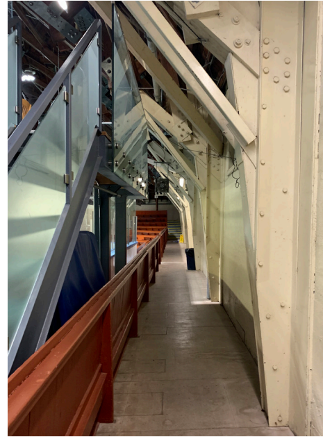
View of interior where new addition is to be located Source: ATA Architects, 2022
