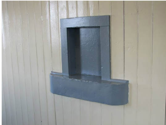
Surviving ticket wicket on west side main hallway.
