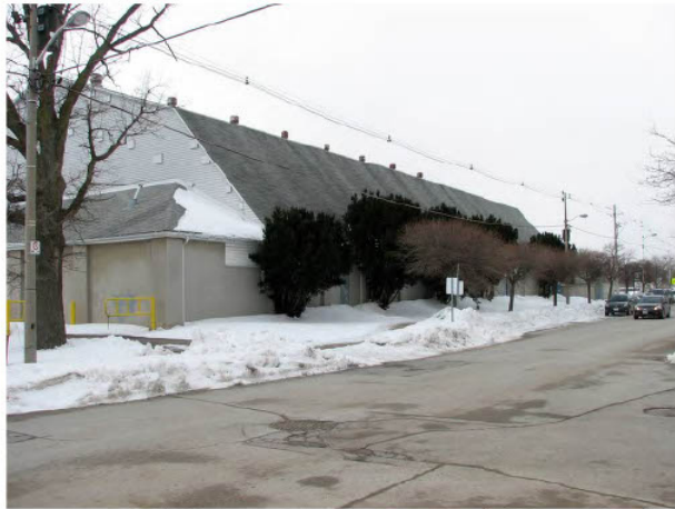
View of east façade, abutting Elliott Street. Image shows landscaping elements flanking the sidewalk and series of roof vents at ridge of roof.
