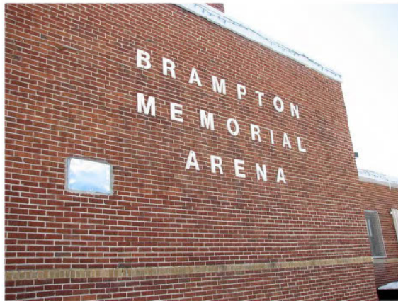
Detail of frontispiece on front façade with original "Brampton Memorial Arena" lettering. Every effort should be made to retain this detail. If letters are replaced in future, the 1950s era typeface and form must be replicated. Alterations that would result in new openings being cut into the masonry walls should be avoided. Masonry repairs should only be made using compatible mortar mix, taking care to match original colour and mortar profile.
