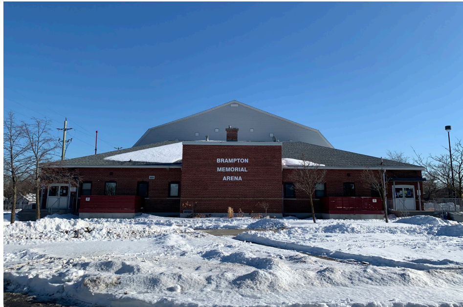
View of the Front of Brampton Memorial Arena Source: ATA Architects, 2022
