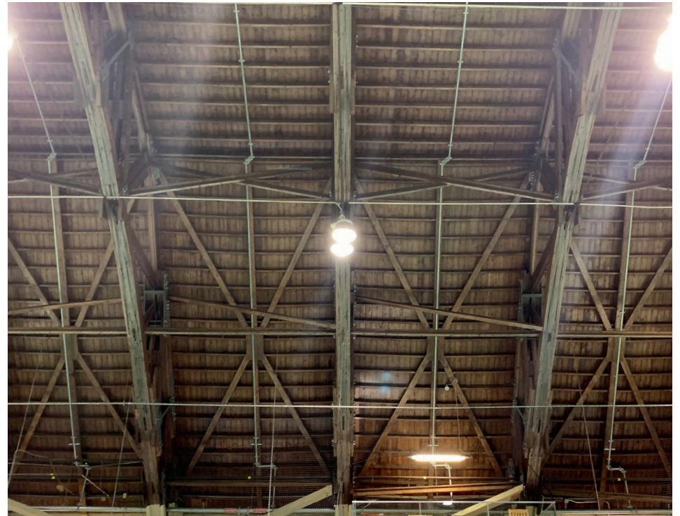
Roof structure in the Brampton Memorial Arena
