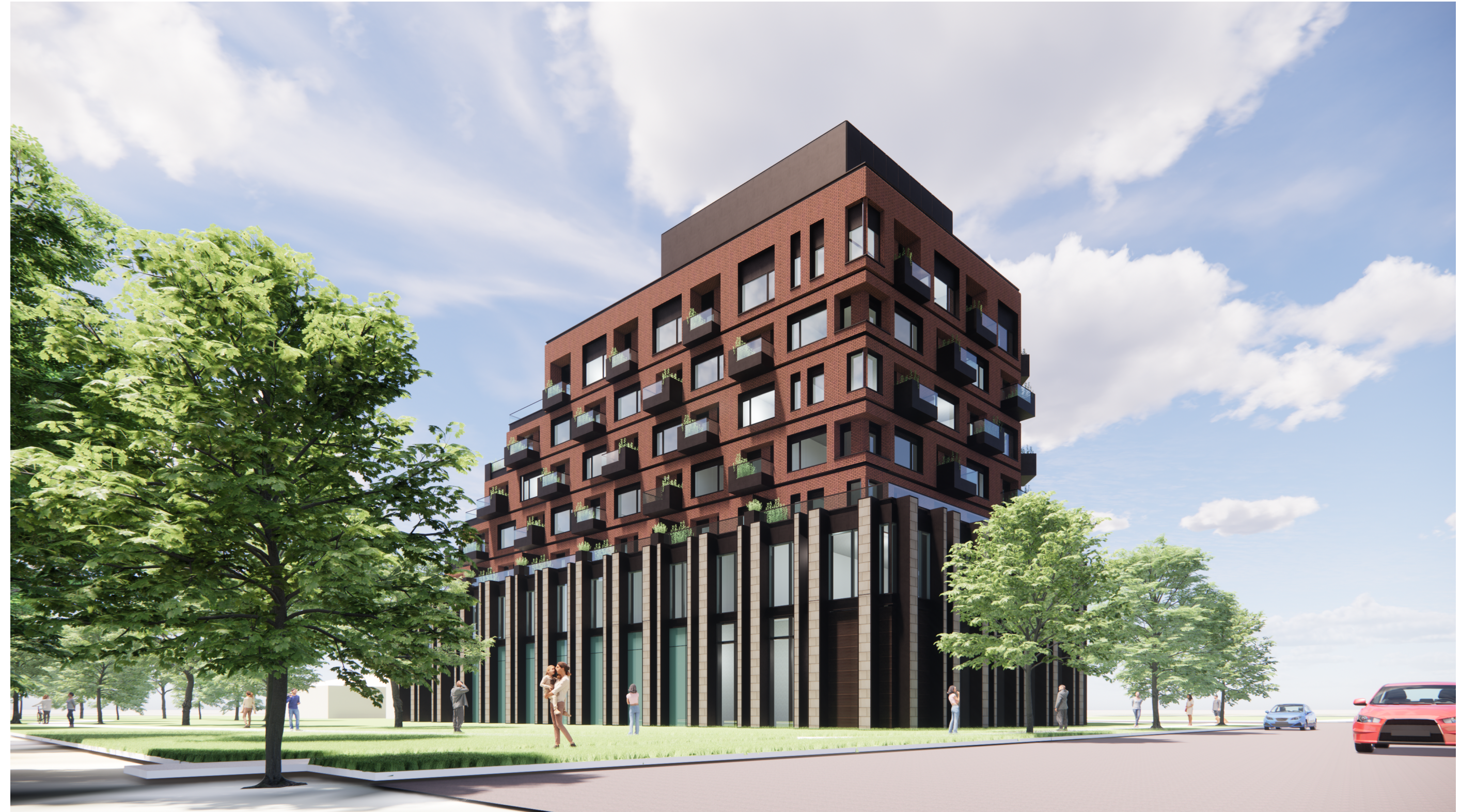
VIEW FROM BRAMALEA ROAD LOOKING WEST
