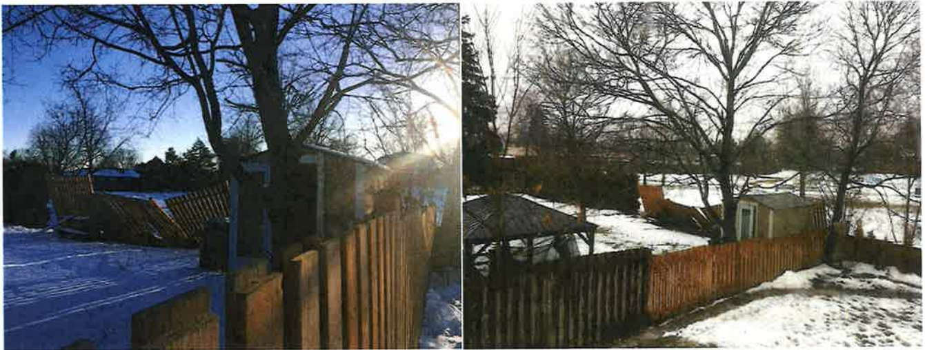
Oversized Fence – no posts, only staked plus zip-tied to chain link fence
