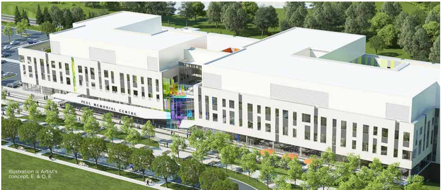
Peel Memorial Phase II expansion
