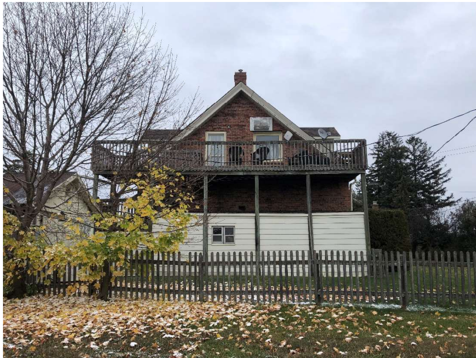
Image 4: View of the rear (west) elevation of the schoolhouse.
