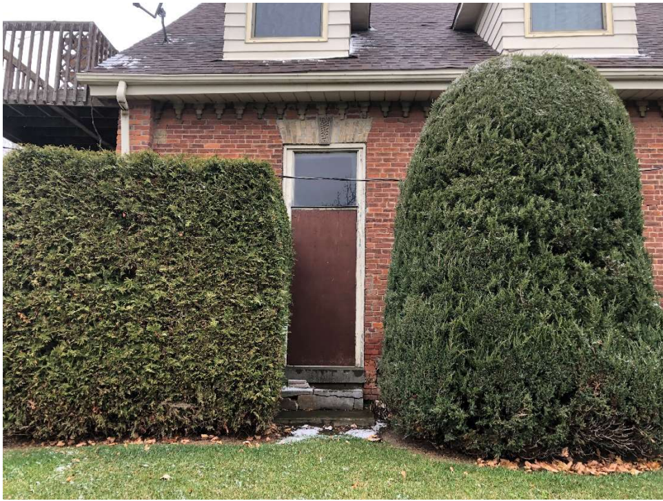
Image 10: View of the door on the south elevation of the schoolhouse.
