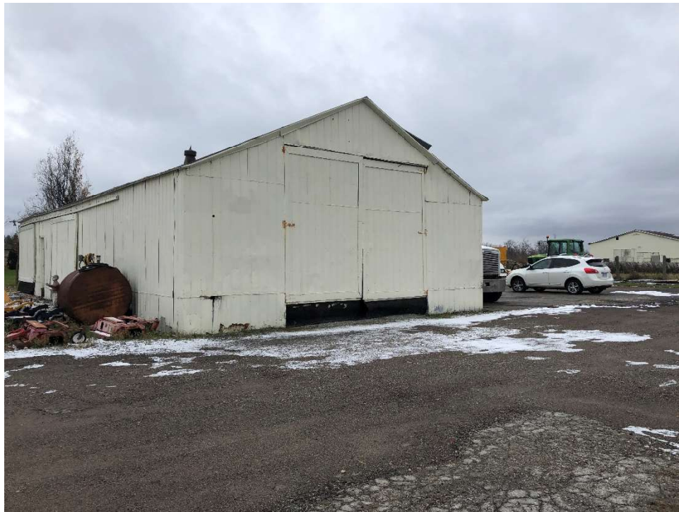
Image 17: View looking southwest towards the eastmost farm building.
