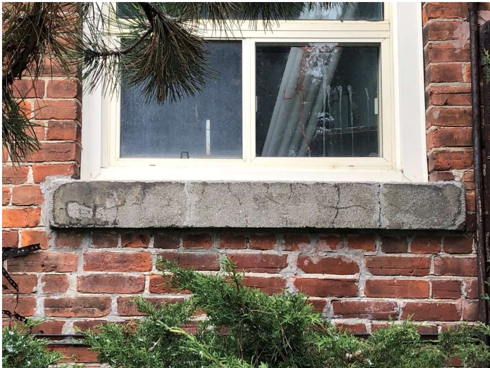
Image 11: Detail of a concrete lintel on the south elevation of the schoolhouse.
