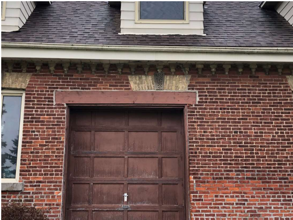
Image 7: View of the garage door on the north elevation of the schoolhouse, note the remnant buff brick lintel with keystone from the former window opening.
