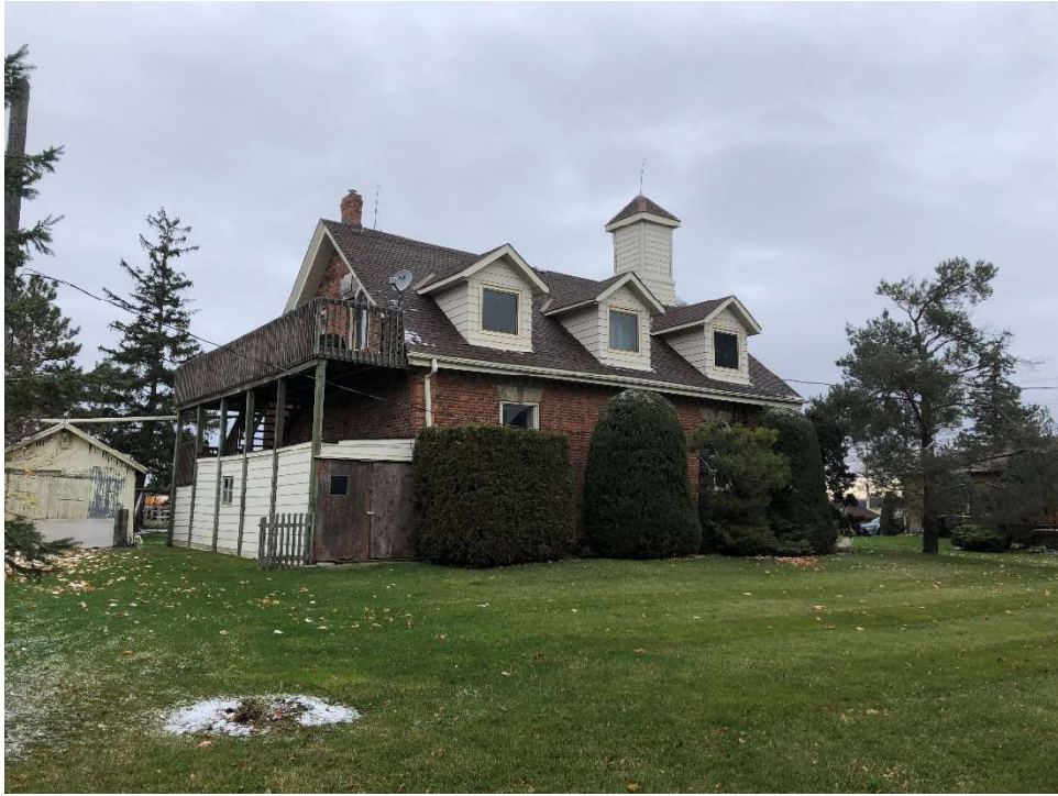
Image 8: View of the rear elevation and south elevation of the schoolhouse.
