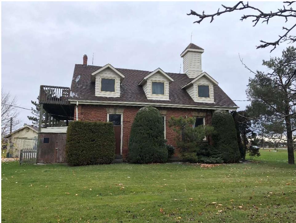
Image 9: View of the south elevation of the schoolhouse.
