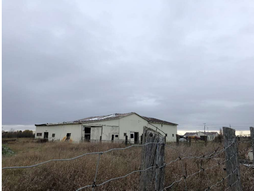
Image 15: View looking northeast towards the westmost farm building.
