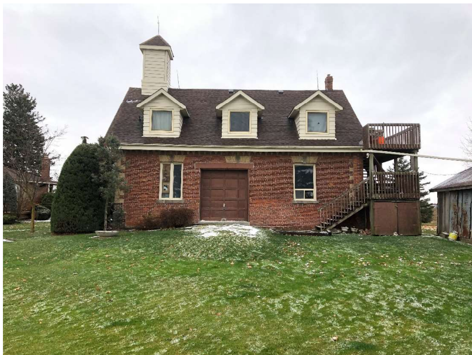
Image 5: View of the north elevation of the schoolhouse.
