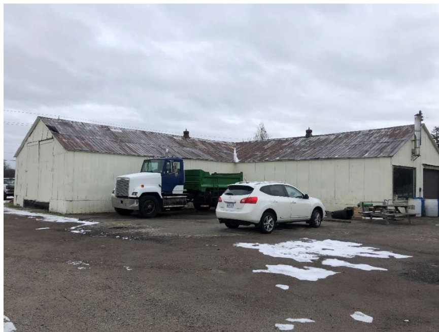
Image 18: View looking southeast towards the eastmost farm building.
