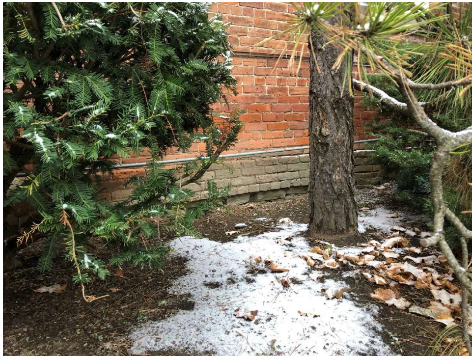
Image 12: View of the foundation from the south elevation.
