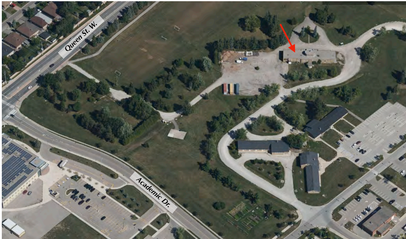
Birds eye view of the subject site, showing its relationship to the institutional buildings west of Academic Drive, the former institutional buildings on the grounds to the east, and 8870 McLaughlin Road South – the Former Administration Building of the ‘Ontario Mental Tubercular Hospital’/‘Former OPP Administrative Building’ (1938) by architect James Henry Craig. This building is located on the upper right hand corner of the image above (and noted by the red arrow).
