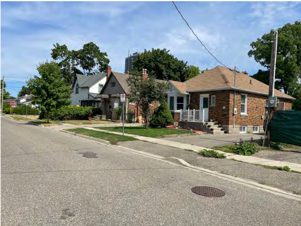
1920s WAR-TIME BUNGALOWS – ROCK-FACED CONCRETE BLOCK FOUNDATIONS SIMILAR TO THE SUBJECT DWELLING
