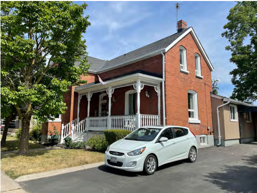
19 TH CENTURY BRICK FARMHOUSE NEXT DOOR
