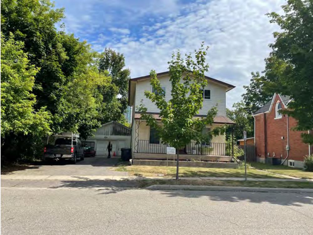
VIEW FROM WEST STREET – 2-STORY DWELLING WITH A SIDE DRIVEWAY & SMALL DETACHED GARAGE
