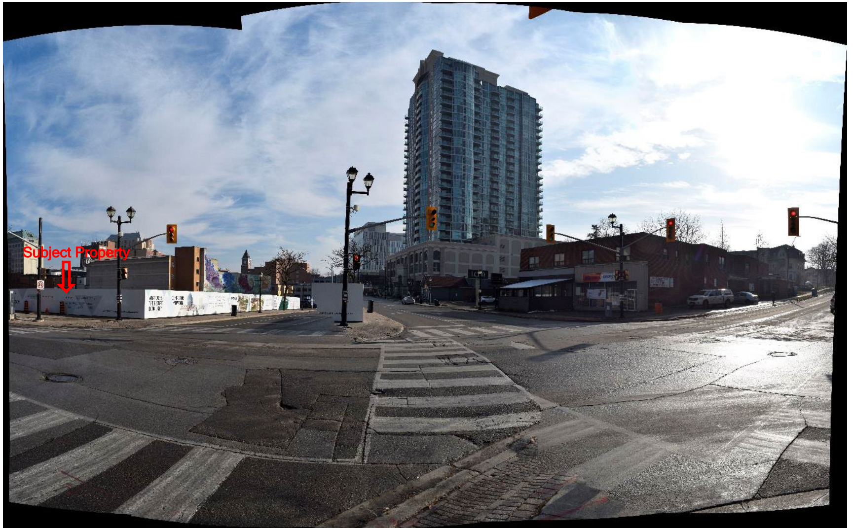
Figure 4: Composite overview of 21 Nelson Street West (as indicated), facing southeast
