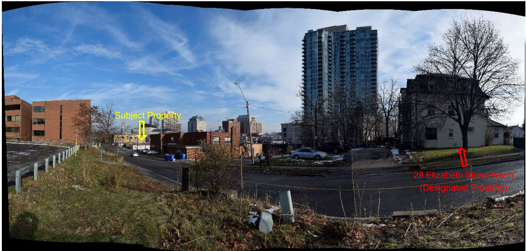
Figure 6: Composite overview of 21 Nelson Street West (as indicated), facing east-northeast
