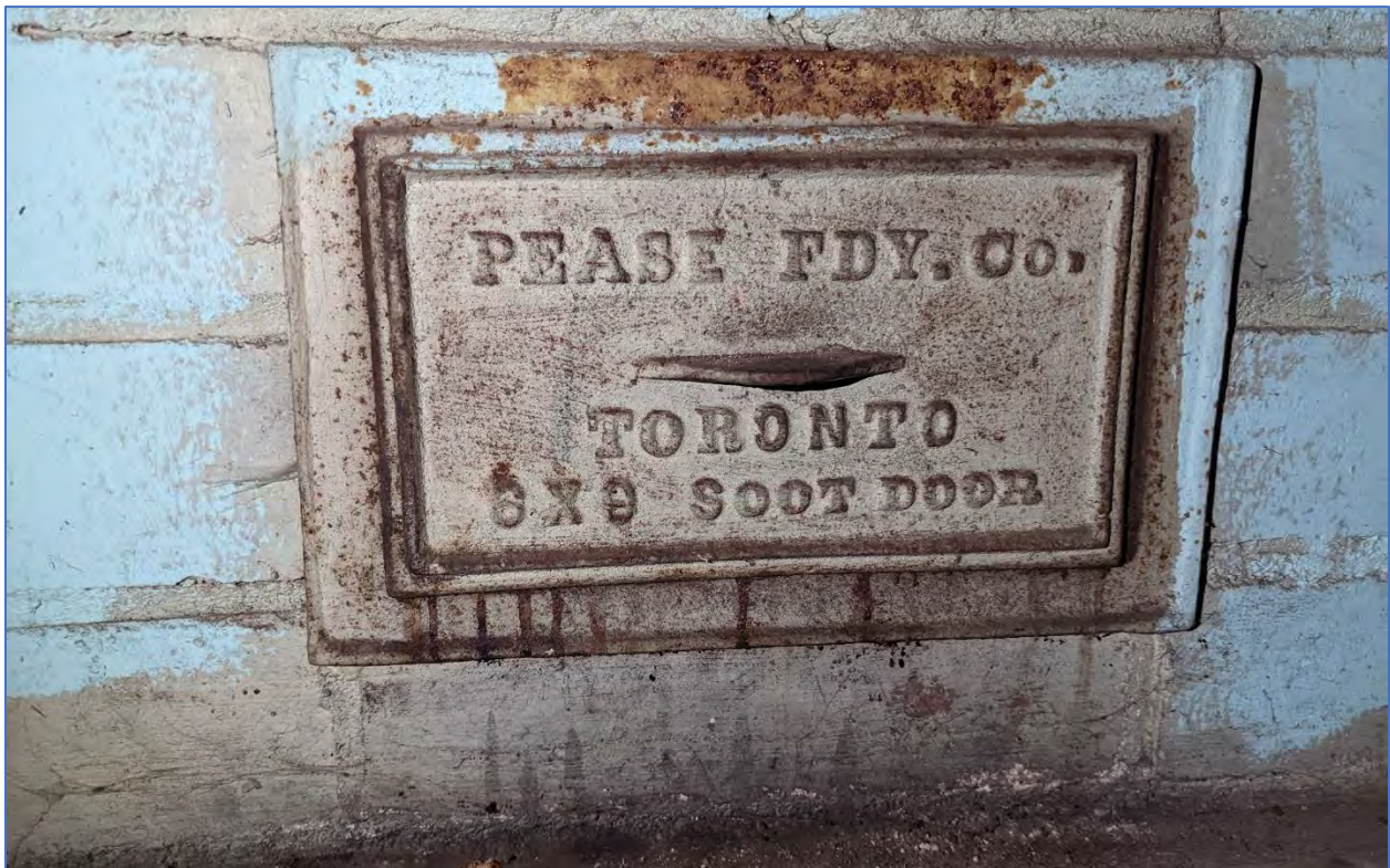
Photo 29: View of soot door on chimney
