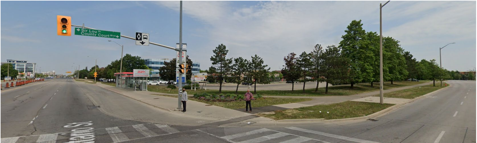
Streetview: Subject Site from Intersection of Hurontario Street and County Court Boulevard
