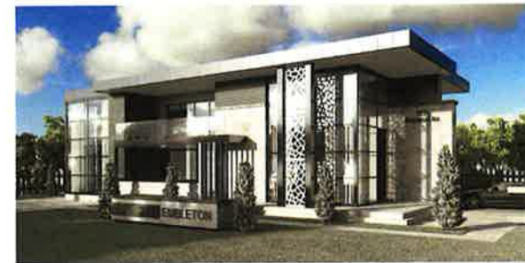
North -West (main) View
