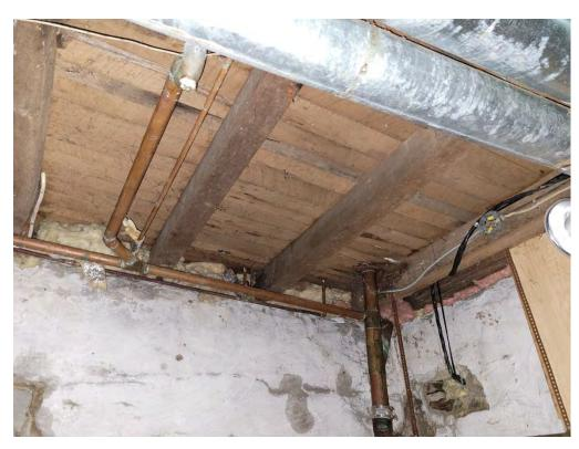
Figure 51: Exposed floor joists with circular sawn marks left in the rough beneath the north extension
