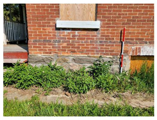
Figure 19: Rubble foundation of the wing and watertable with splayed stretcher
