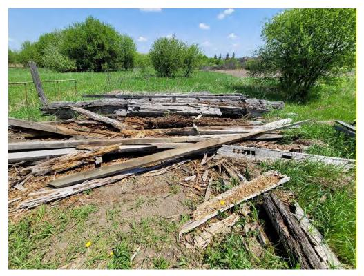
Figure 56: Timber-framing from the demolished gable barn
