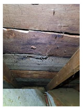
Figure 49:Rough wood sheathing within the attic of the extension
