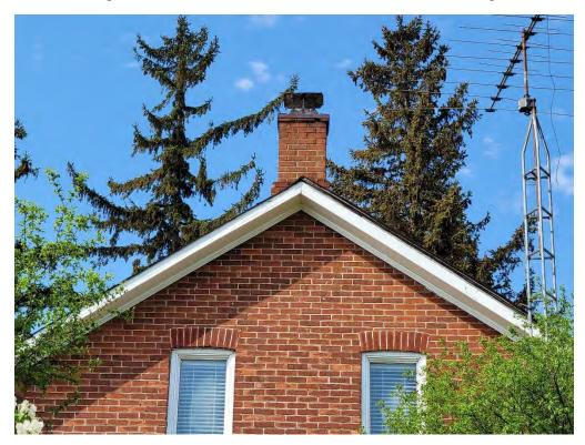
Figure 24: Single-stack brick chimney on the side right centre of the side gable
