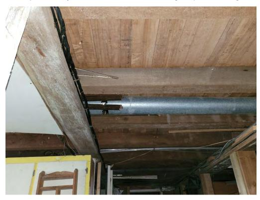
Figure 42: Exposed floor joists with circular sawn marks left in the rough in the side gable portion
