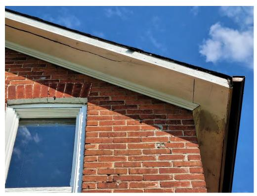
Figure 20: Projecting eaves and verges of the main block wing with plain fascia, soffit, and prefabricated gutter
