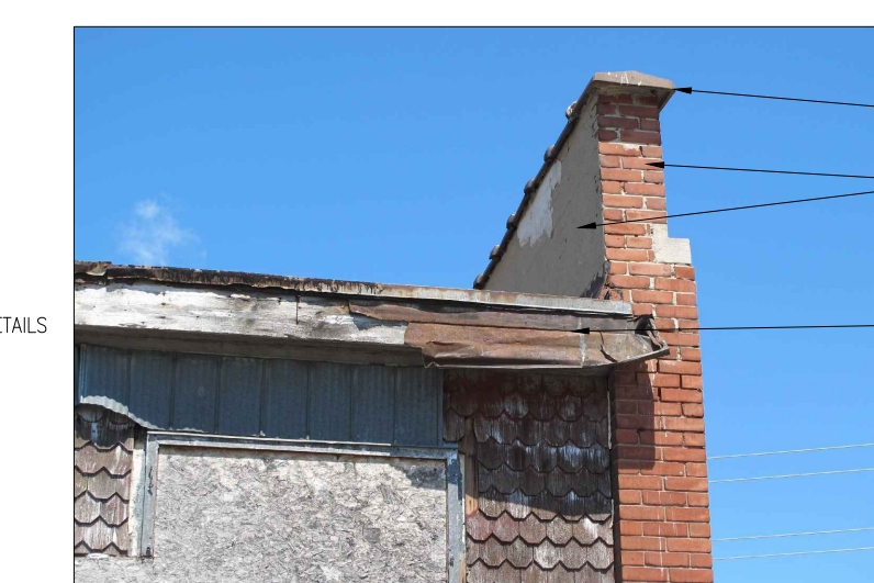
South Facade @ Parapet 3 HA202
