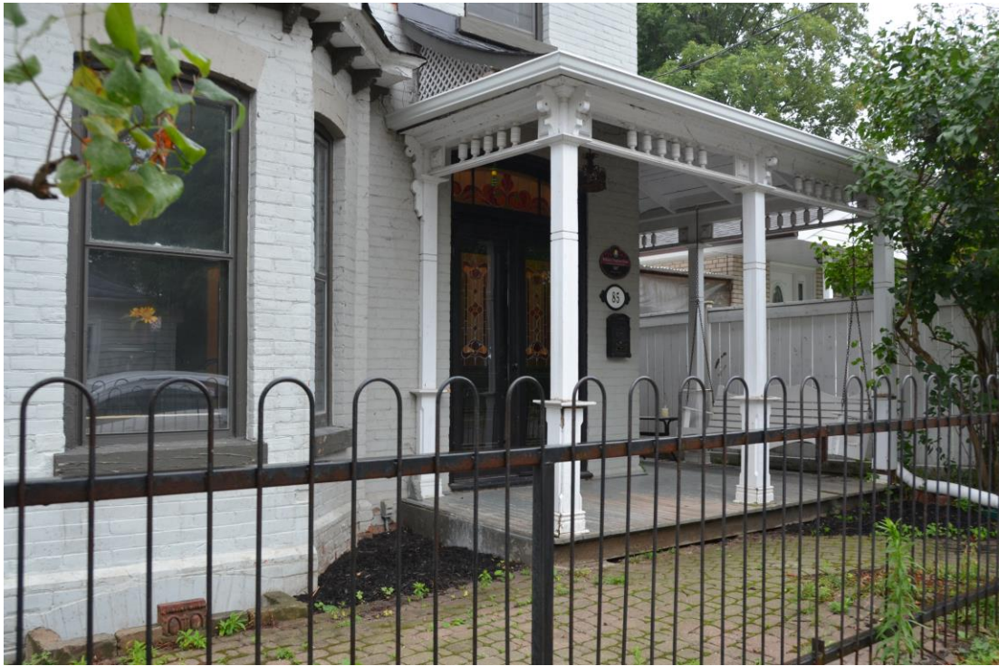
Figure 6: Front porch and details, which wraps partially around the west side (Source: City of Brampton, 2019)
