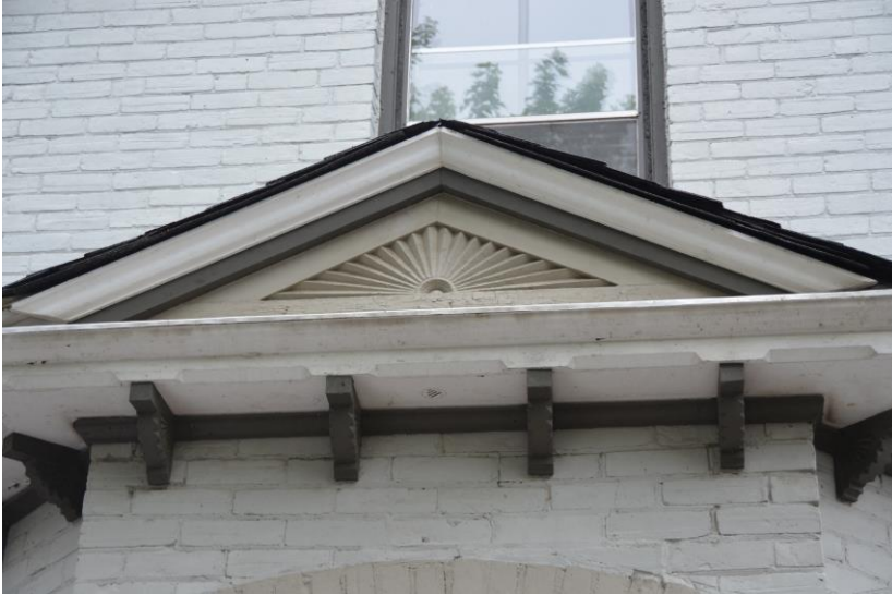
Figure 12: Sunburst detail on gable above bay window, east elevation (Source: City of Brampton, 2019)
