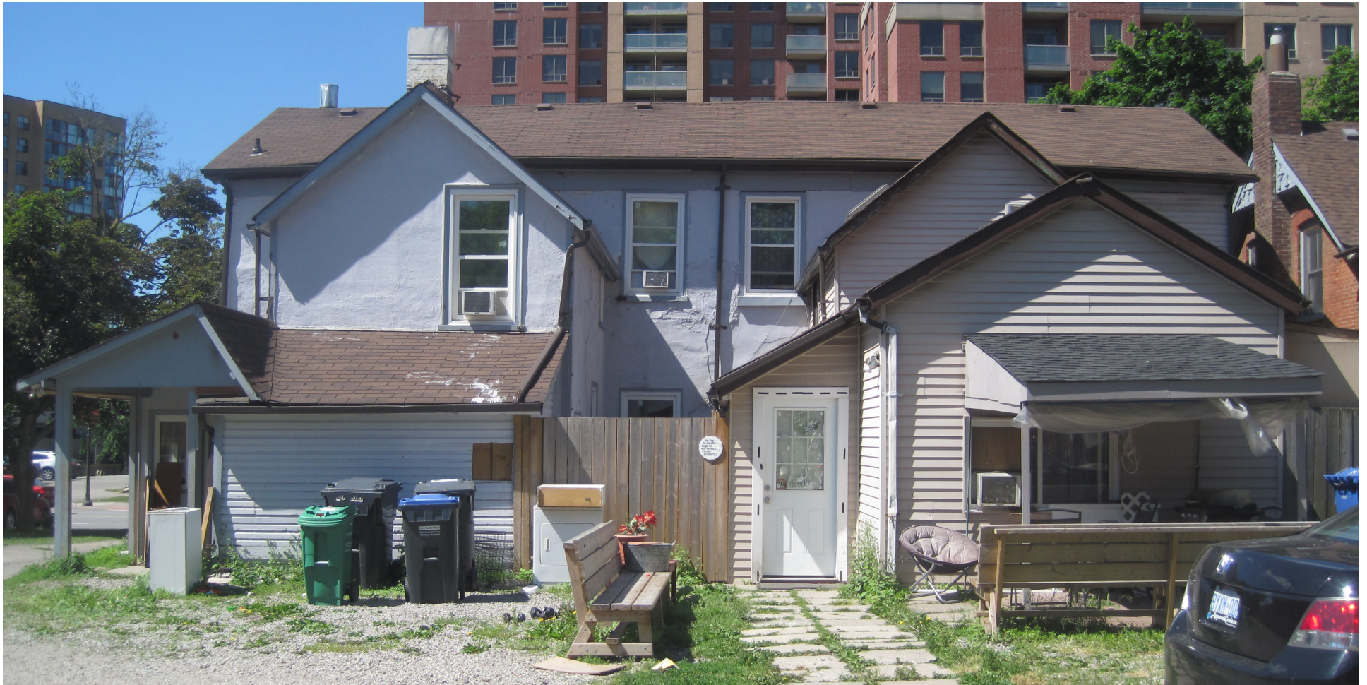
Rear view from East (rear of the lot).
