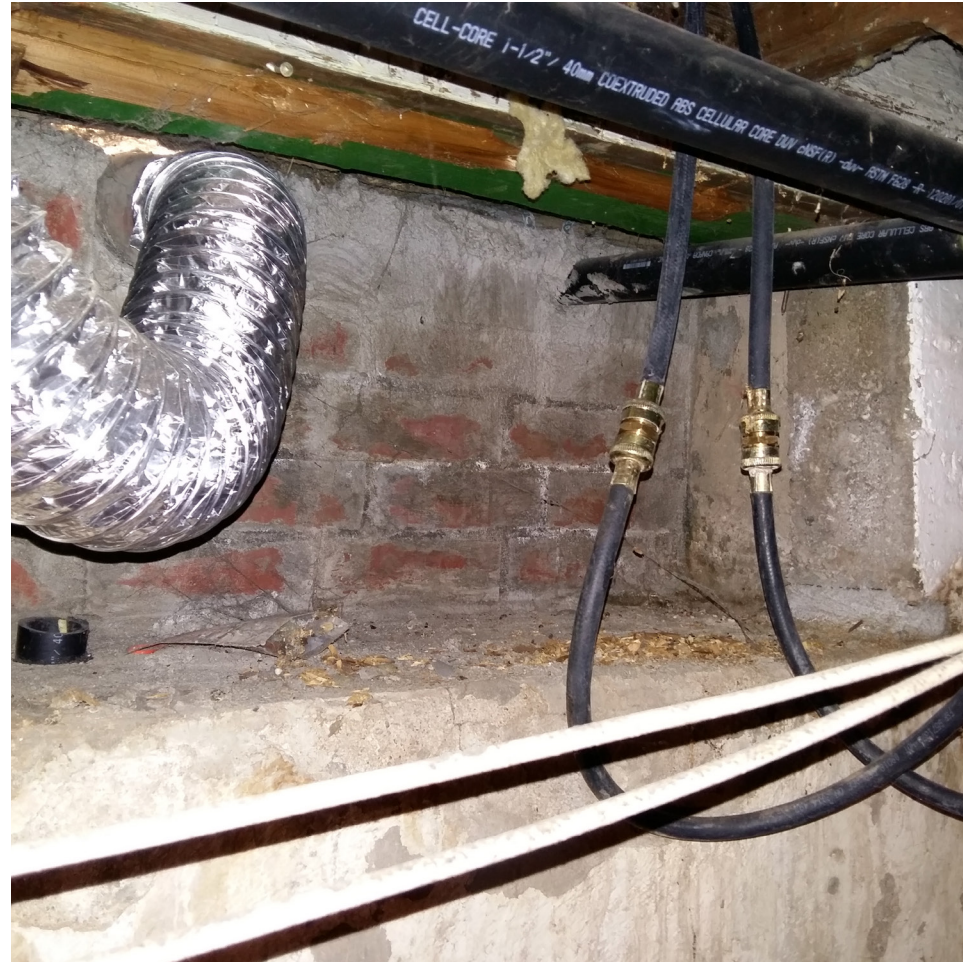
Concrete masonry walls have been built against the inside of the original brick walls.
