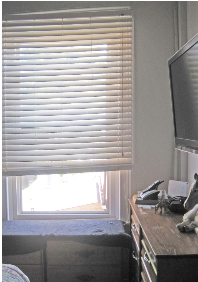
Window and door trims appear to be original in the second floor.
