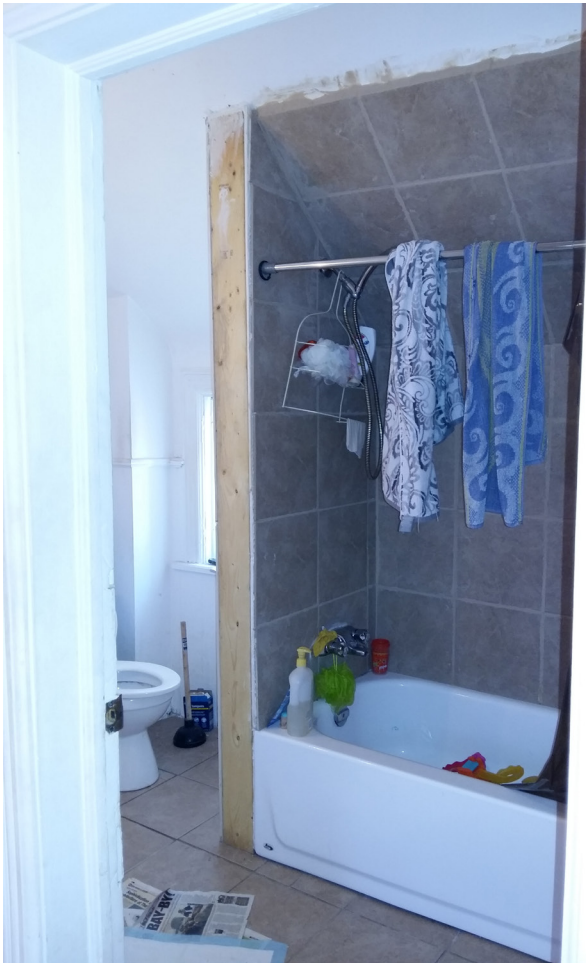
A bathroom is located in the rear addition.
