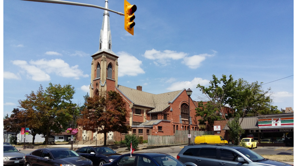
Grace United Church neighbouring the property to the south, a heritage designated property.
