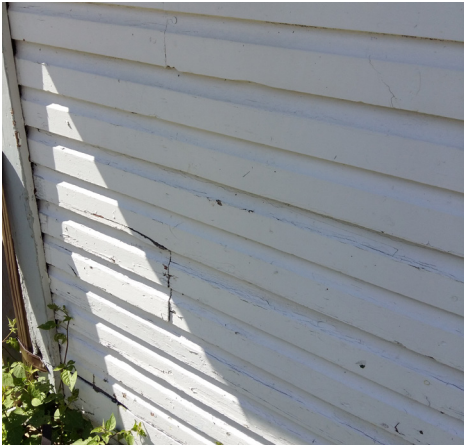
Wood siding at rear 1 storey section of 164 Main Street North
