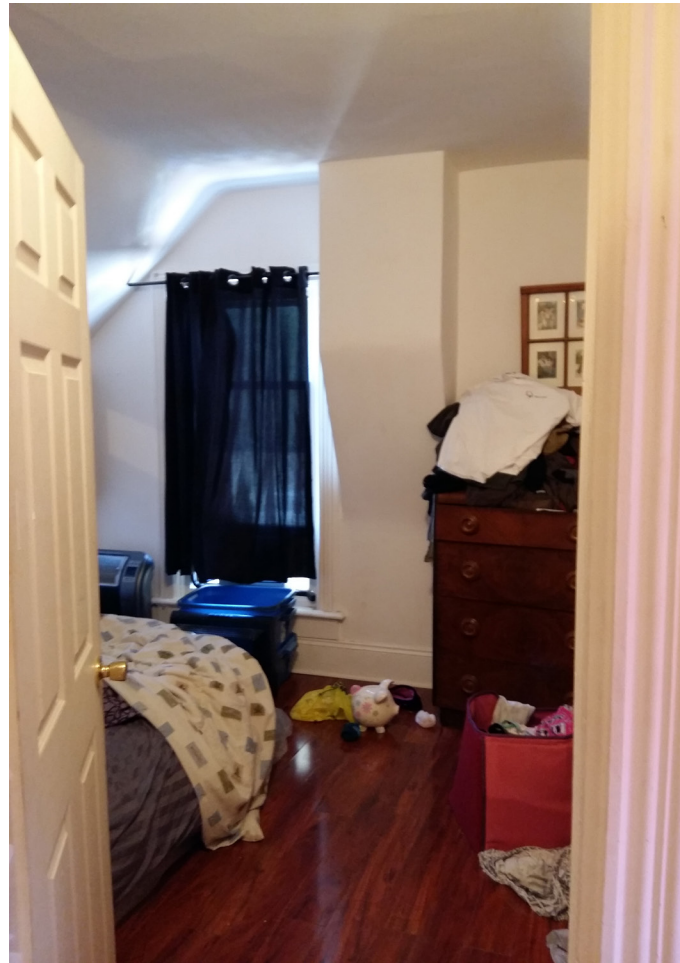
Bedroom in the rear addition of the unit. Trim and baseboards are worth salvaging
