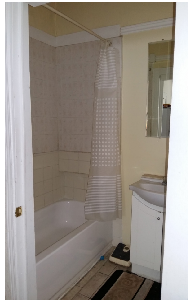
Bathroom located off of the kitchen.
