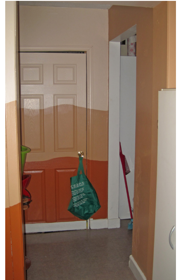
This opening marks the division between the rear addition and the front two storey section.
