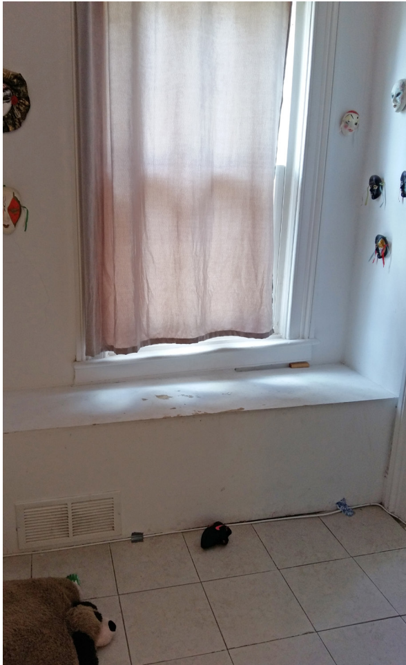
Window seat, appears it may have been put in for ducting given the vent in the lower left corner.
