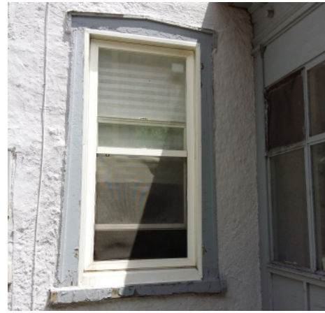
Windows have been changed but the original wood trim was retained
