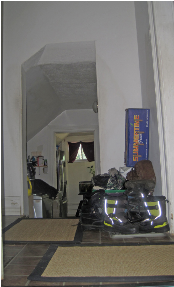
View from the stairs through to the rear addition.
