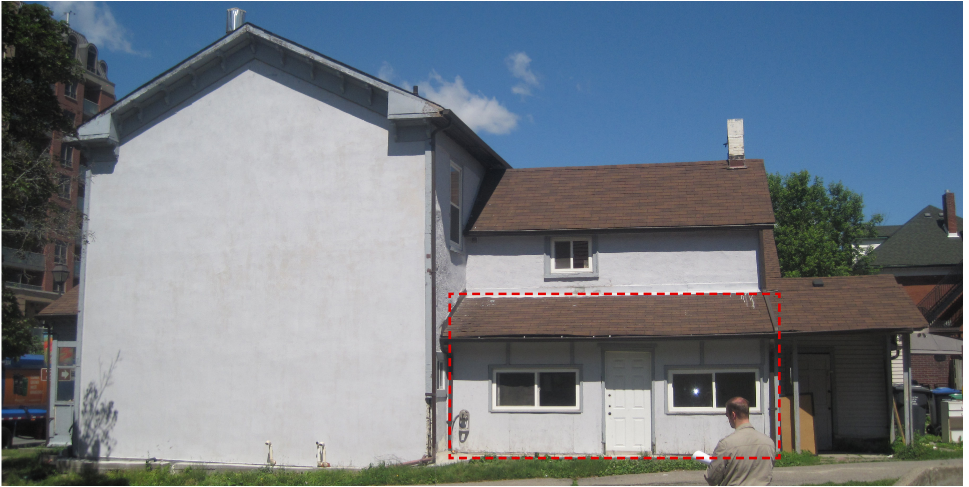
Side view from South. Area marked by red rectangle appears to be a later addition clad in painted particle board. The wall of the one and a half storey section extends down behind this addition.
