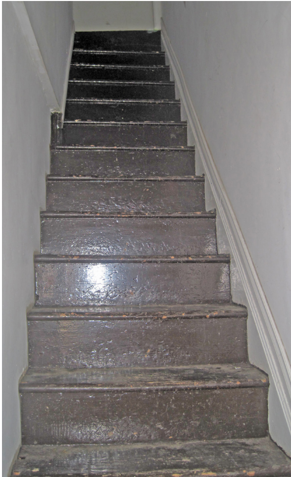
Stairs to the second floor of 166 Main Street.
