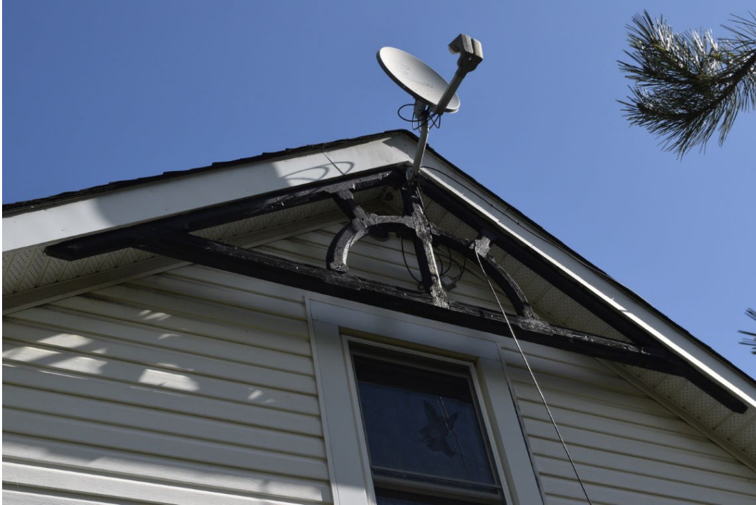
Figure 22: Millwork in gable end of front façade
