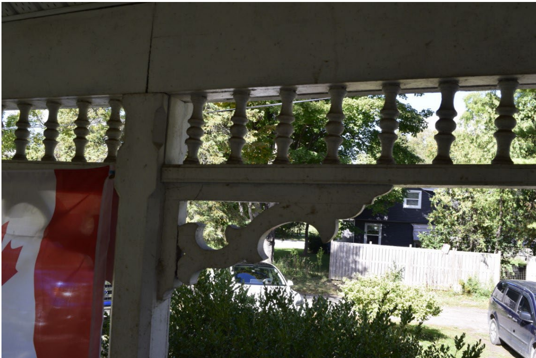
Figure 21: Millwork on north porch
