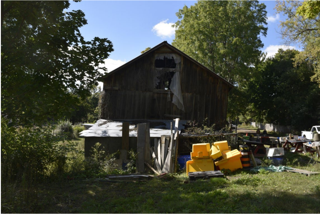
Figure 56: East face of outbuilding facing west
