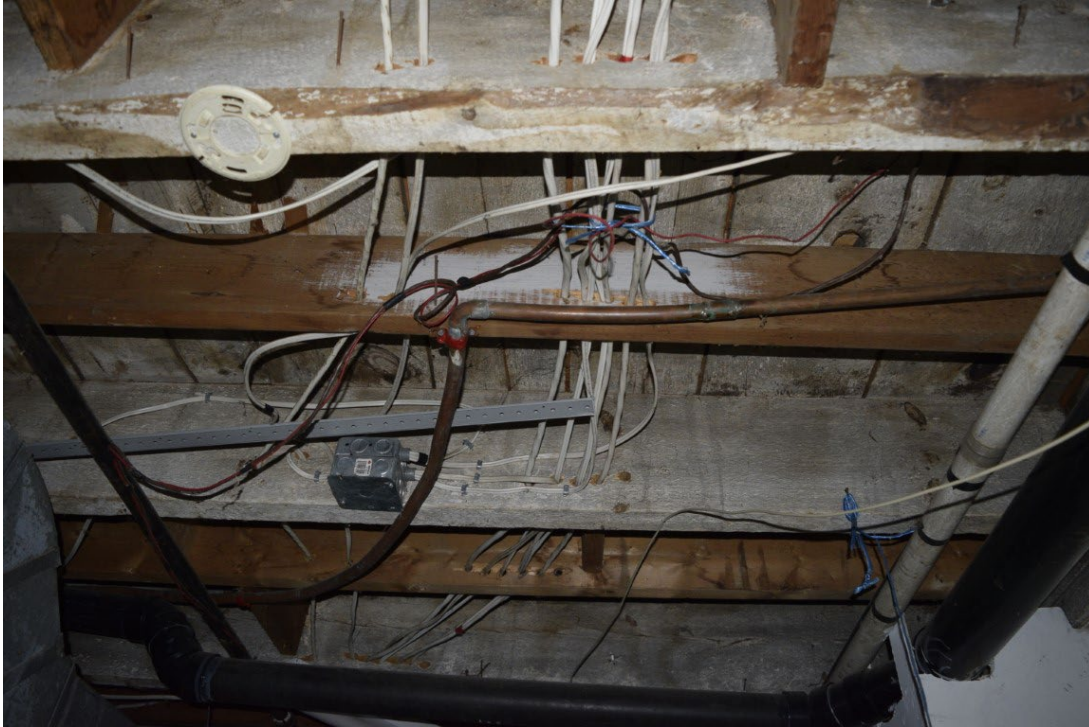
Figure 46: Typical circular sawn floor joists
