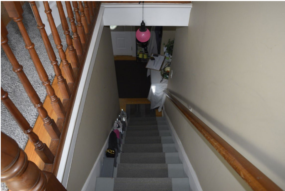
Figure 29: Original stairs in front apartment
