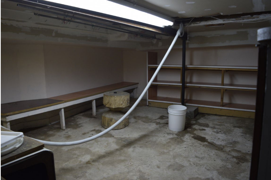
Figure 42: Basement under original portion of rear addition, facing west
