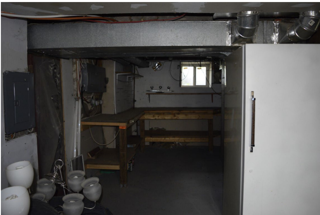
Figure 43: Basement under rear apartment, facing north
