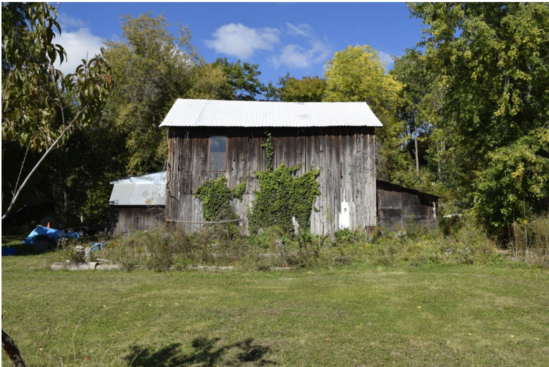
Figure 57: South face of outbuilding facing north
