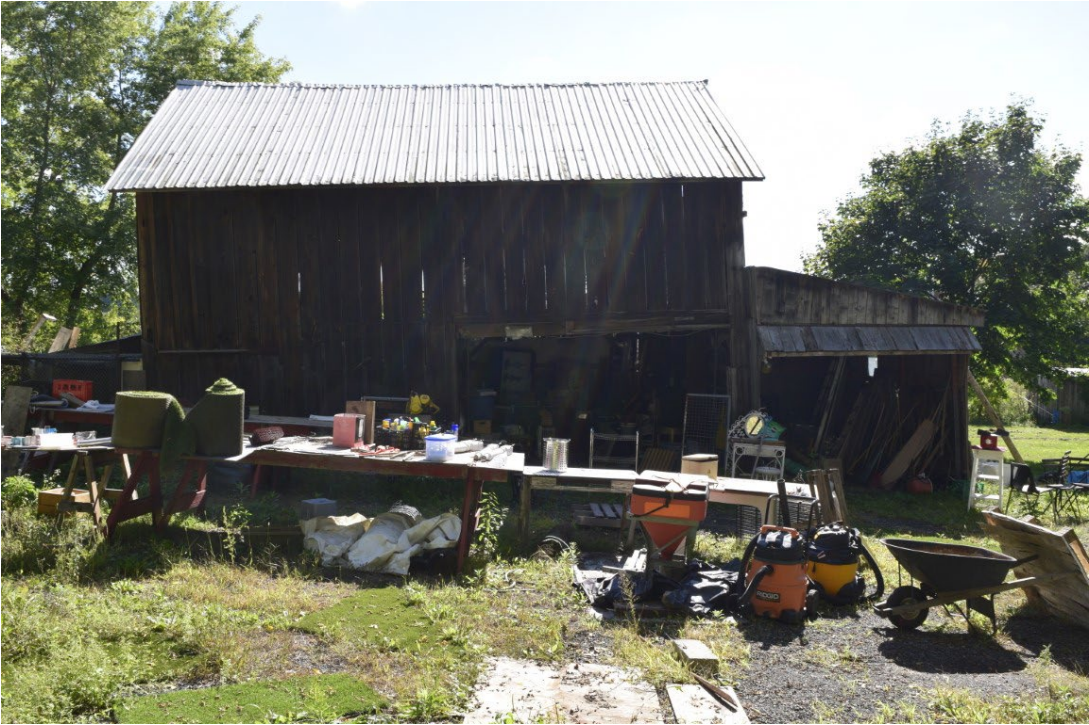
Figure 54: North face of outbuilding, facing south
