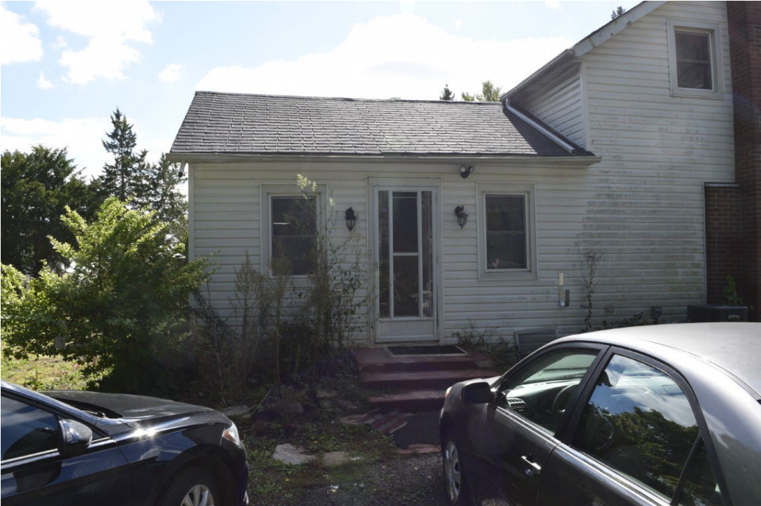
Figure 19: North face of rear addition
