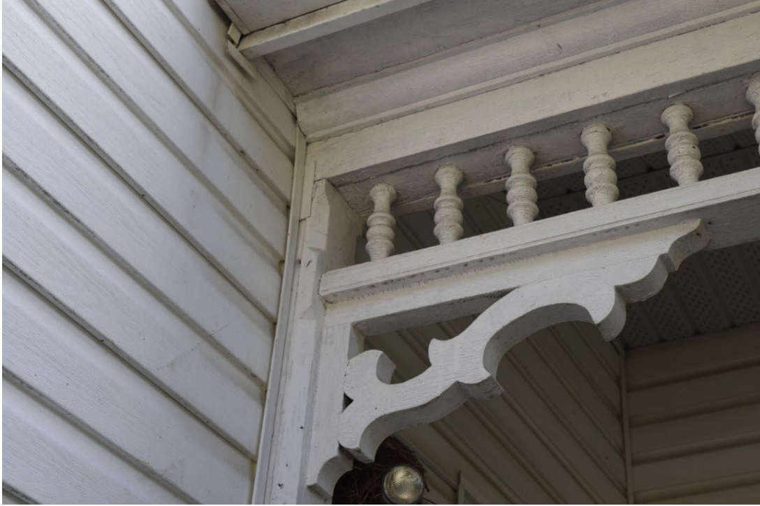
Figure 20: Millwork associated with north porch
