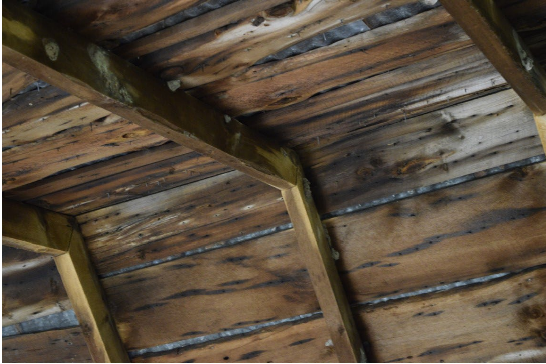
Figure 60: Close up of rafter and roof planking
