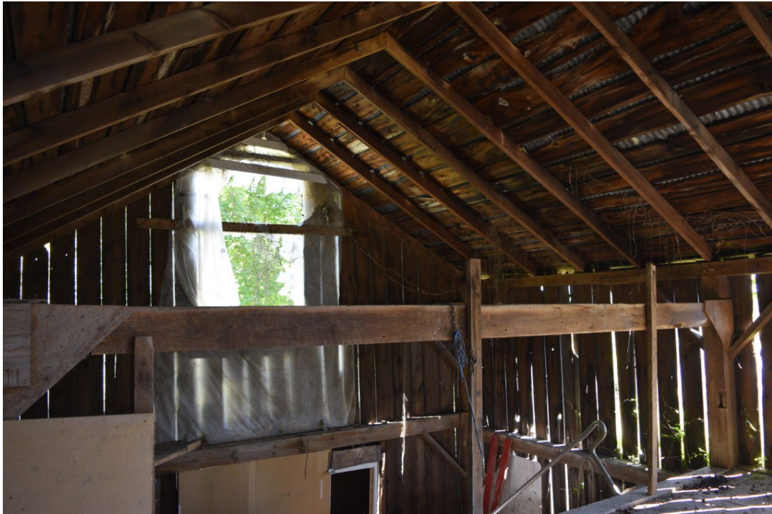
Figure 58: Interior of outbuilding, facing southwest
