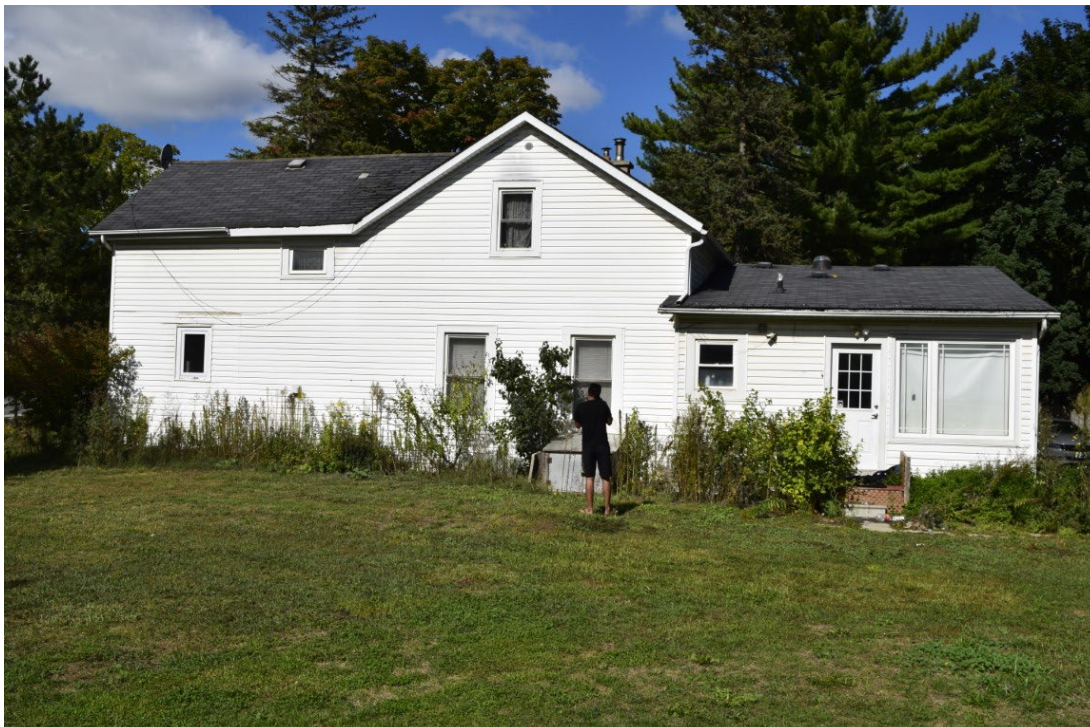
Figure 15: South face of residence, 1973 addition is on right side of image, original house is on left
