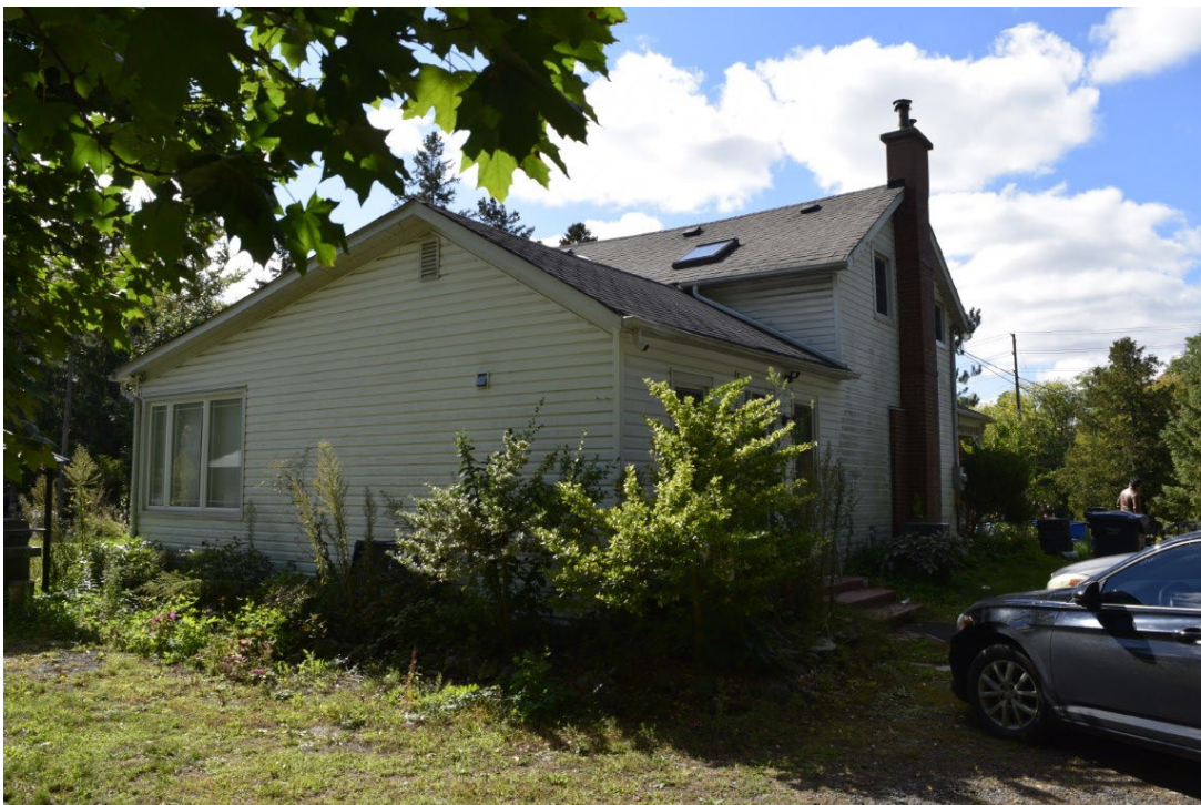
Figure 17: Northeast face of residence
