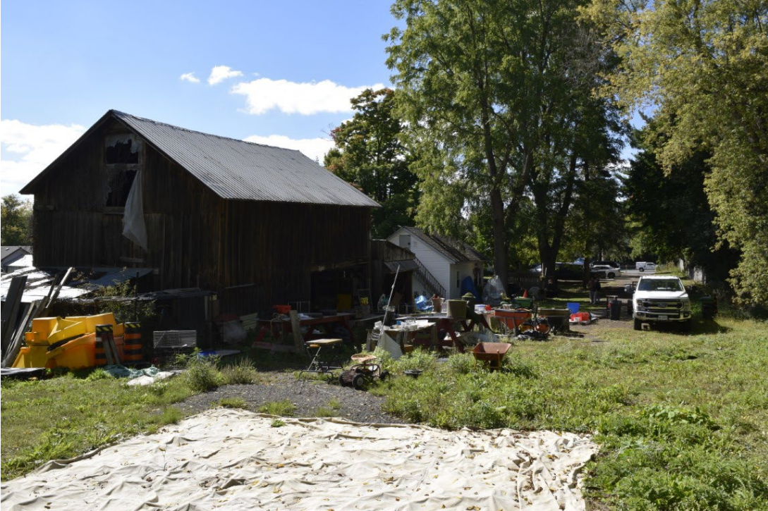
Figure 55: Northeast corner of outbuilding
