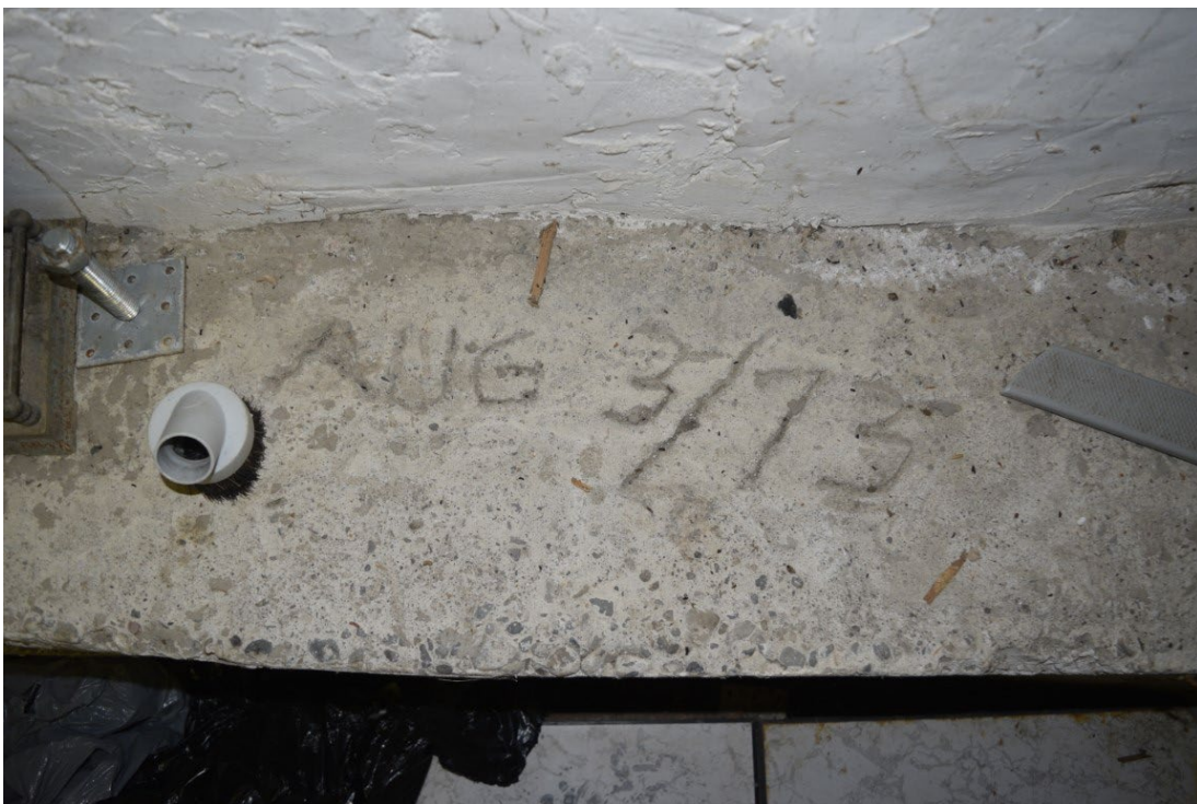
Figure 45: August 3 1973 has been written in the concrete foundation associated with the rear addition
