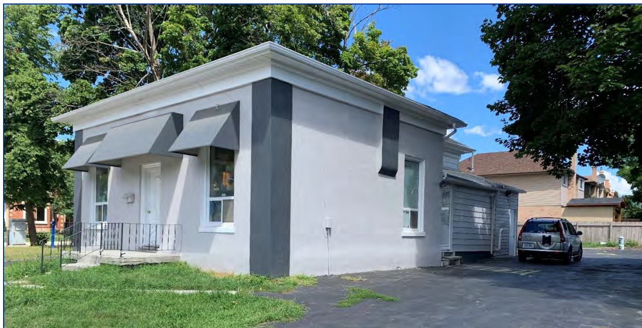
Photo 5: View of the north elevation and the side parking lot.
