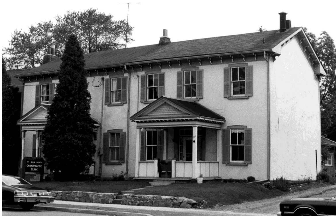
Figure 6: Photograph of 164 & 166 Main Street North in the early 1980s (Source: City of Brampton)
