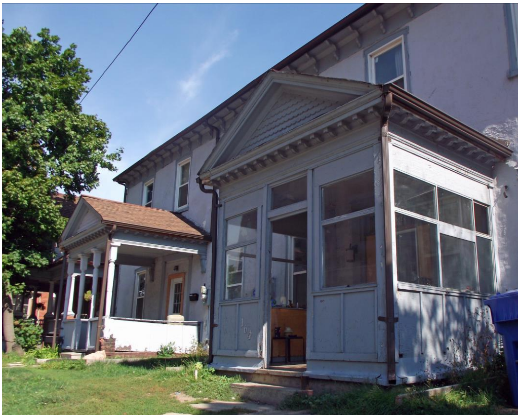
Figure 8: Current front porches with original pediments adorned with scalloped siding (Source: City of Brampton)
