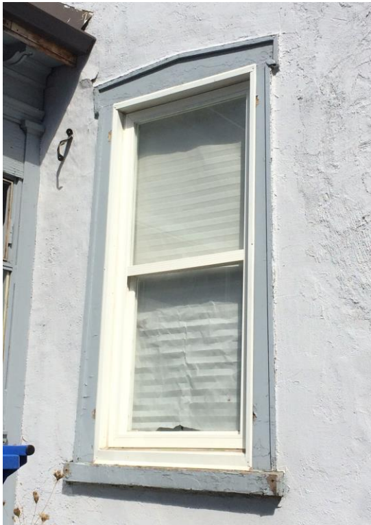
Figure 12: Unique wood window casing (Source: City of Brampton)
