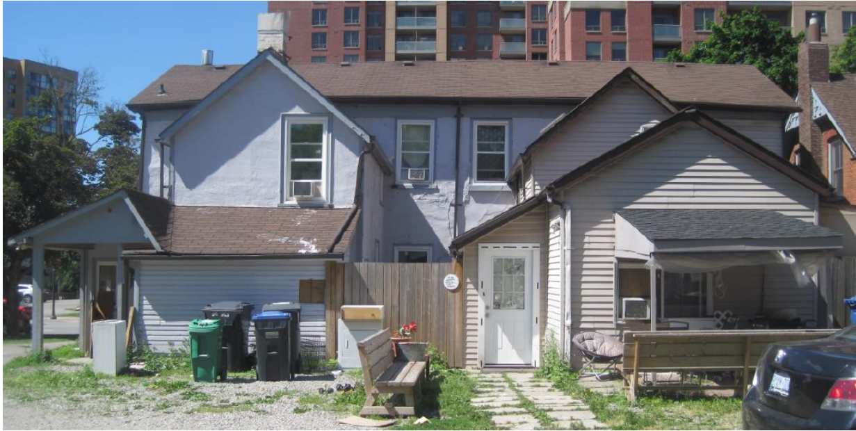
Figure 13: Rear facades showing variety of additions (Source: ATA Architect)
