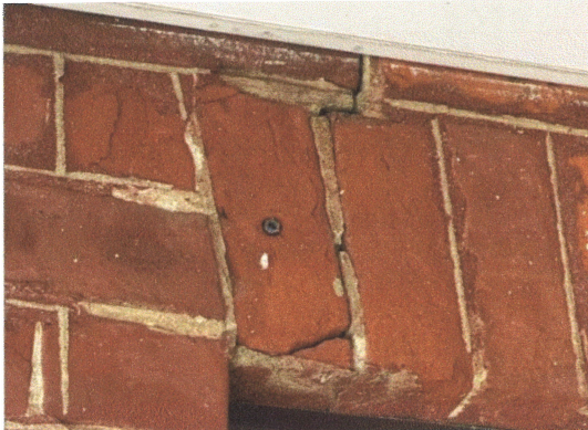
Movement at Voussoir Brick (Arch Brick) Gap Beside Door Frame
