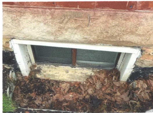
Caulking & Painting Req. at Basement Window
