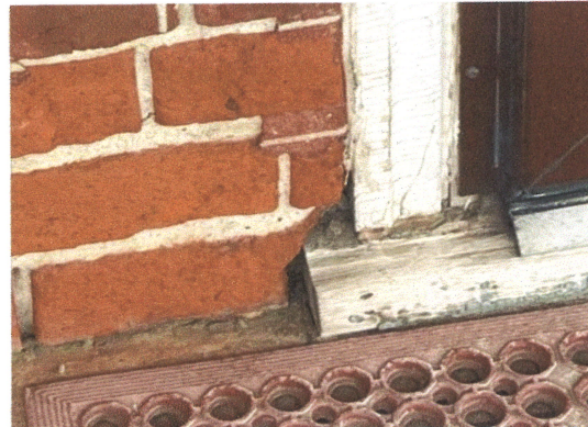
Movement at Voussoir Brick (Arch Brick) Gap Beside Door Frame
