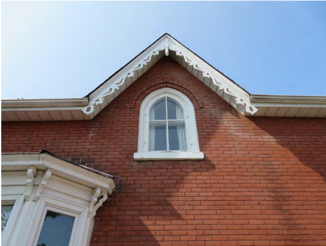
GABLE ON SOUTH ELEVATION – DECORATIVE BARGEBOARD - GOTHIC WINDOW - RAISED BRICK HOOD MOULD – TWO OVER TWO WOOD SASH
