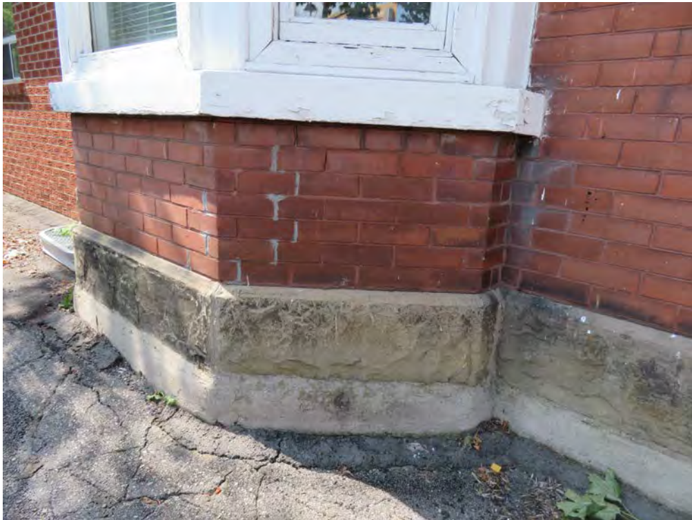
STONE FOUNDATION WITH QUARRY-CUT FACE - UNDERPINNED WITH CONCRETE
