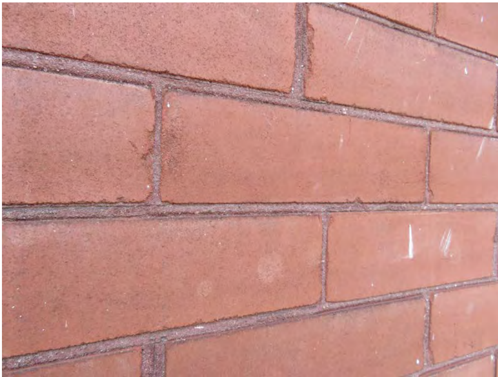
TUCK-POINTED MORTAR JOINTS
