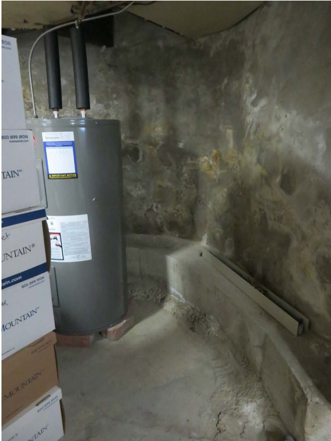
PARGING ON INTERIOR FACE OF THE FOUNDATION AND CONCRETE SHELF WHERE IT HAS BEEN UNDERPINNED
