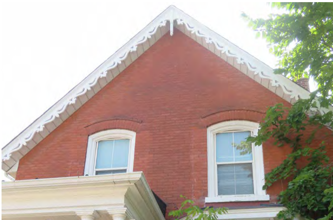
GABLE ON FRONT ELEVATION – DECORATIVE BARGEBOARD – SEGMENTALLY ARCHED WINDOWS – BRICK ARCH AND RAISED BRICK HOOD MOULD – REPLACEMENT WINDOWS
